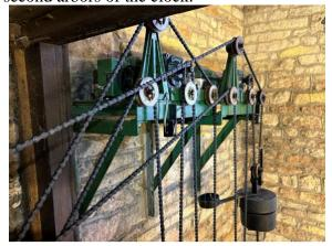
The going winder is operating satisfactorily, but the striking winder had stopped working with the weight right down and the counterweight jammed against the idler pulley. I reset the overwind switch and the winder resumed normal working.
