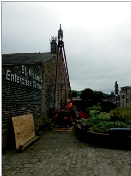
Plate 8: General working shot of trench 7, borehole BH013
