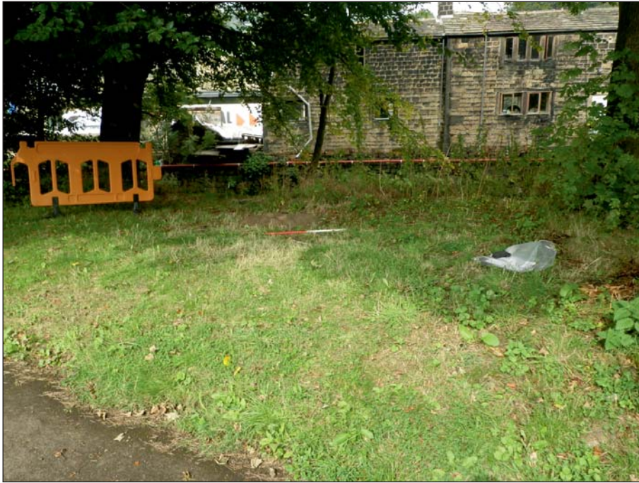
Plate 11: General view of trench 11, window sample BH011
