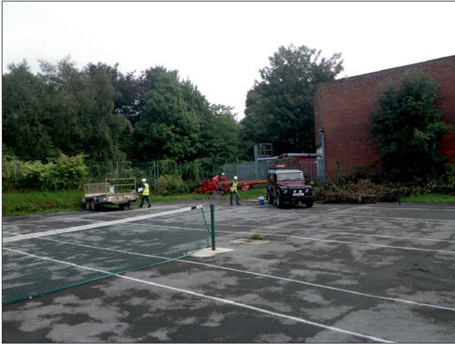
Plate 9: General working shot of trench 9, borehole BH034
