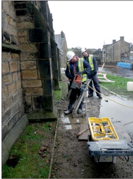
Plate 1: General working shot of inclined core at St Michael's Church
