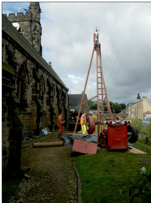
Plate 6: General view of borehole rig at St Michael's Church
