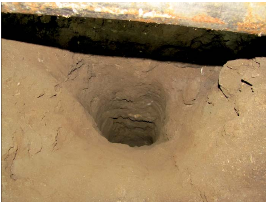
Plate 4: Trench 3 (TP 103) excavated
