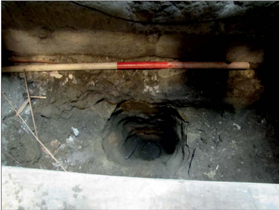
Plate 5: Trench 4 (TP 101) excavated
