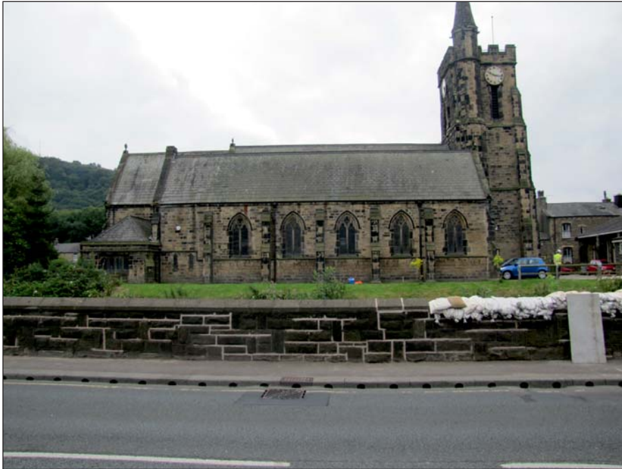
Plate 1: View of the northern facade of the Church
