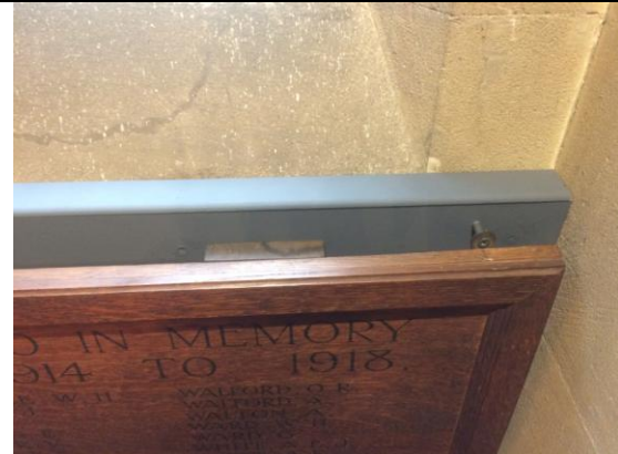
Detail view of screw fixing at upper hanging plate and with metal tube spacer to secure memorial board to secondary board support.
