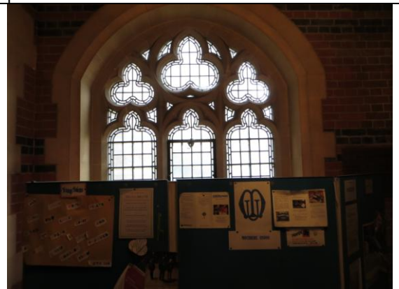
16. Overall view of previous location of memorial board (West window) from front, showing unfiltered/uncontrolled natural light through window
