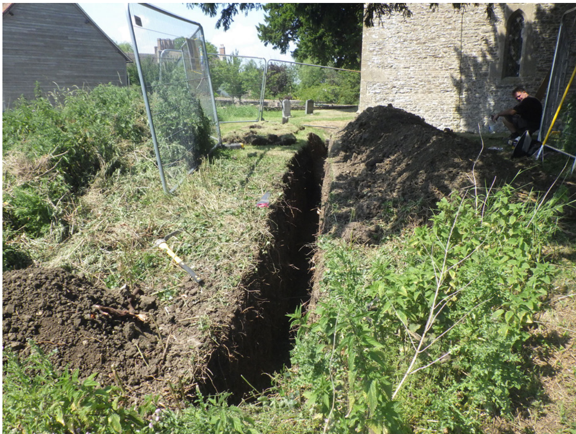
Plate 11: Drainage Trench – looking NNW
