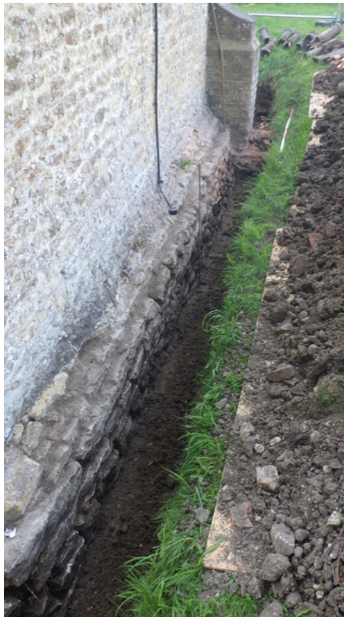
Plate 5: West Wall of Nave – looking SSE
