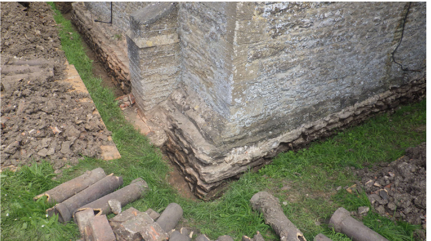
Plate 4: Southwest corner of Nave – looking north-east along west wall
