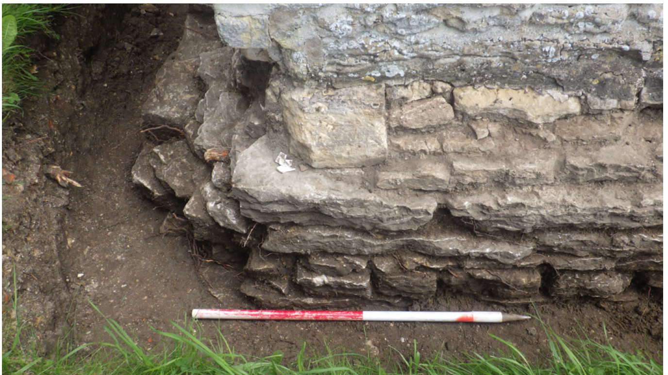
Plate 6: North-west corner of Nave – detail looking east
