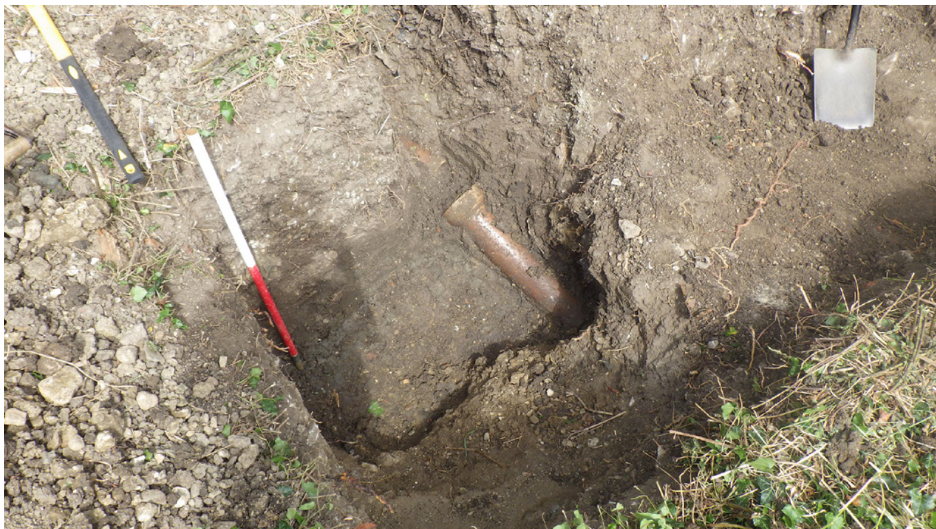
Plate 12: Soakaway – looking north-west
