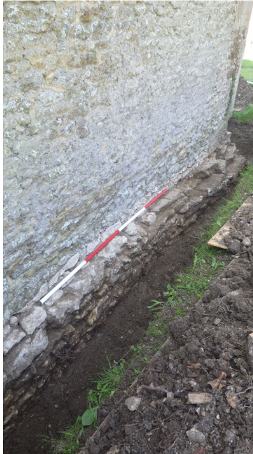
Plate 7: North Wall of Nave – looking south-west
