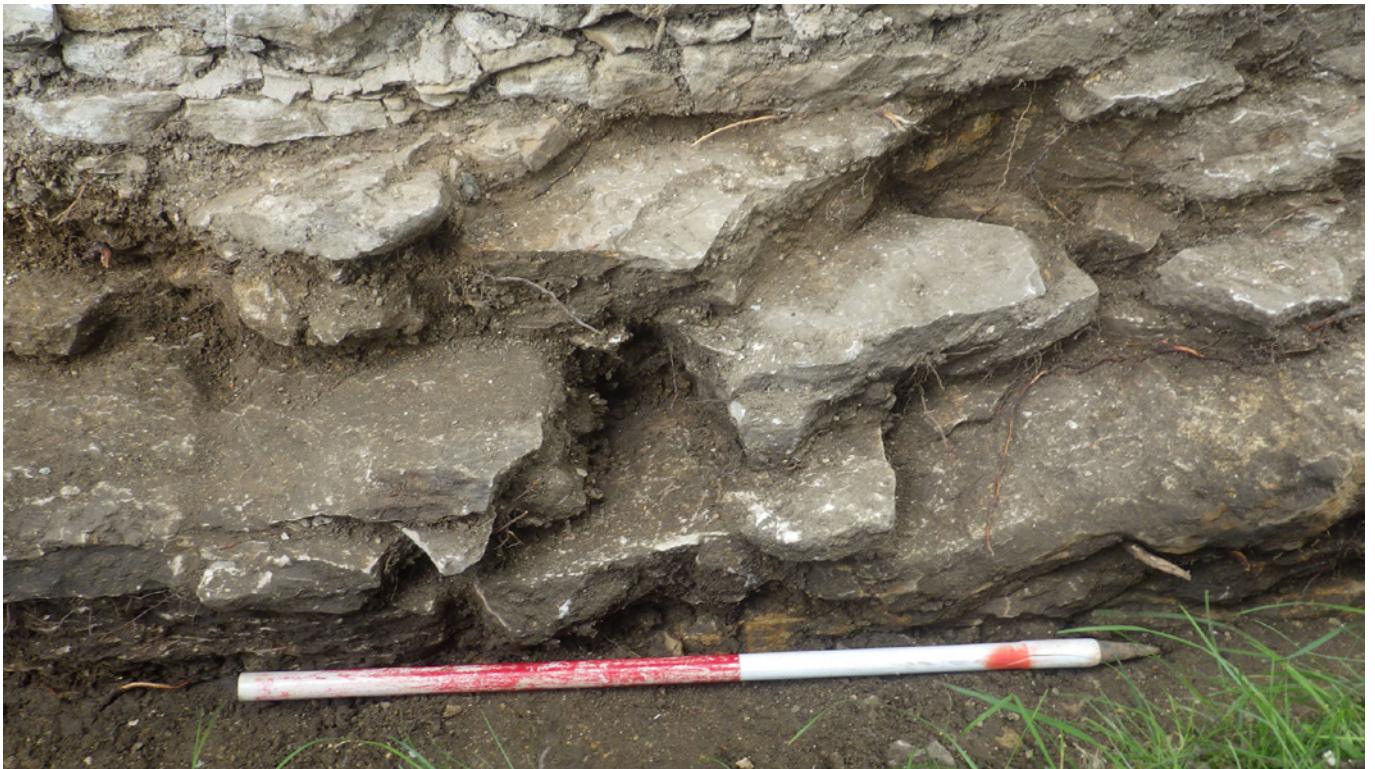
Plate 8: North Wall of Nave – looking south
