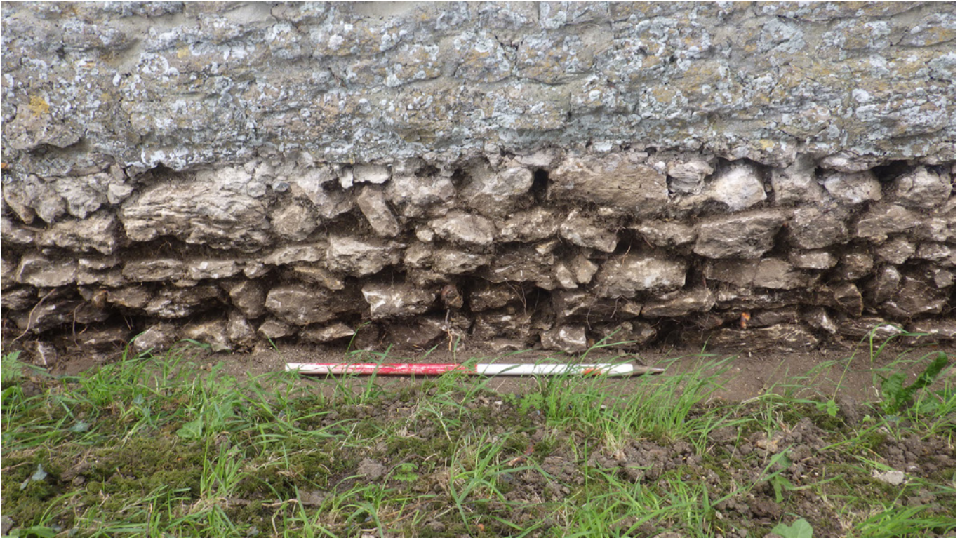
Plate 3: South Wall of Nave - looking N
