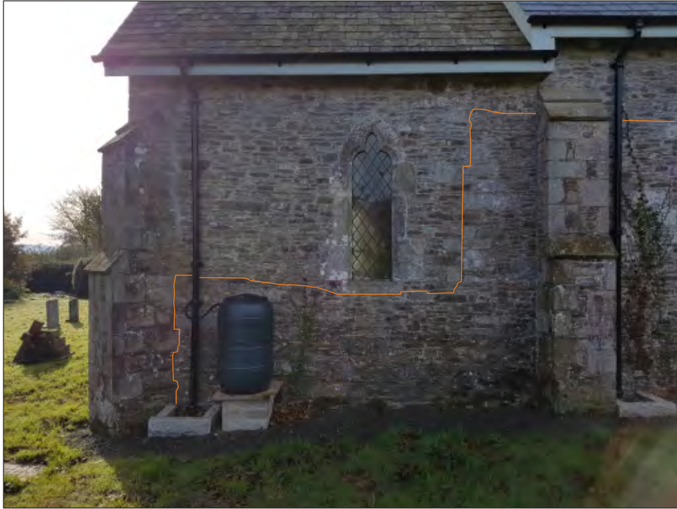
Pl. 16 General view of north elevation showing sections rebuilt in the late 19th century. Looking south.
