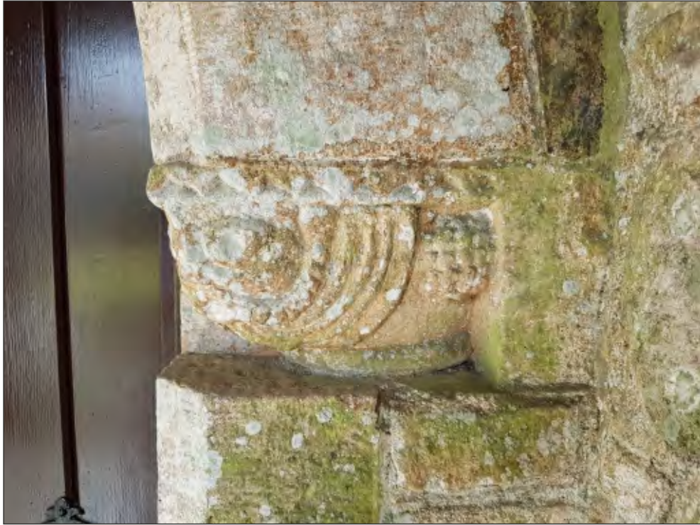
Pl. 6 Close-up of eastern impost. Looking south.
