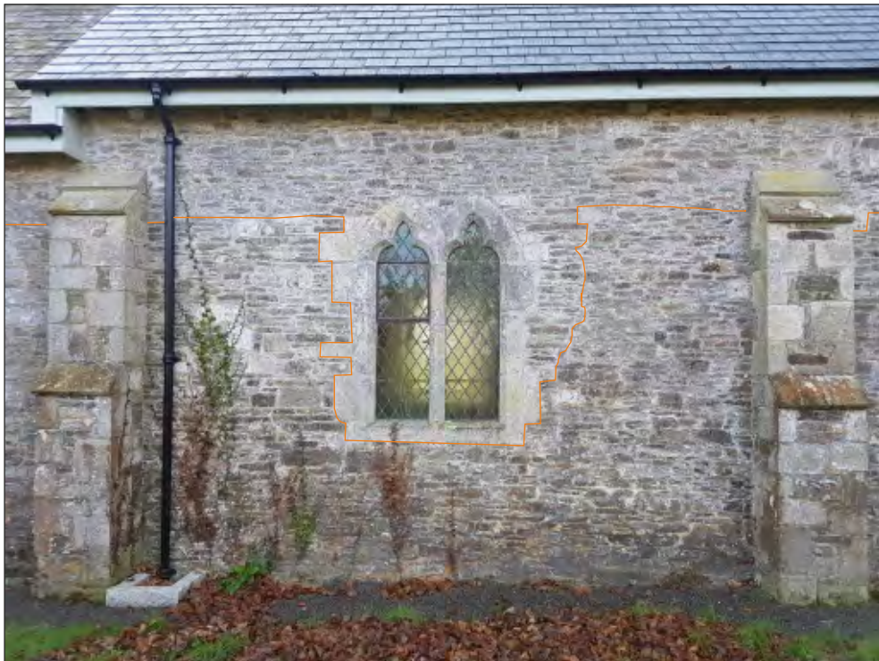
Pl. 17 General view of north elevation showing sections rebuilt in the late 19th century. Looking south.
