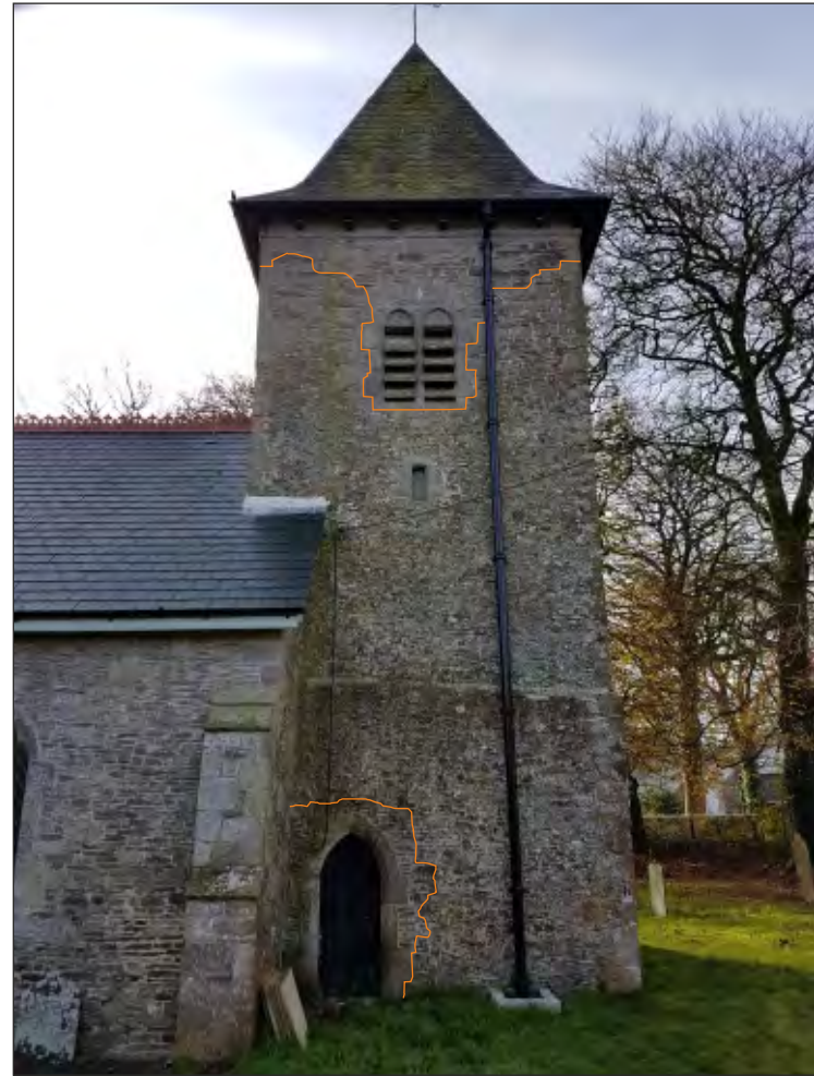
Pl. 13 General view of church tower showing 19th century rebuild (top) and door insert. Looking south.
