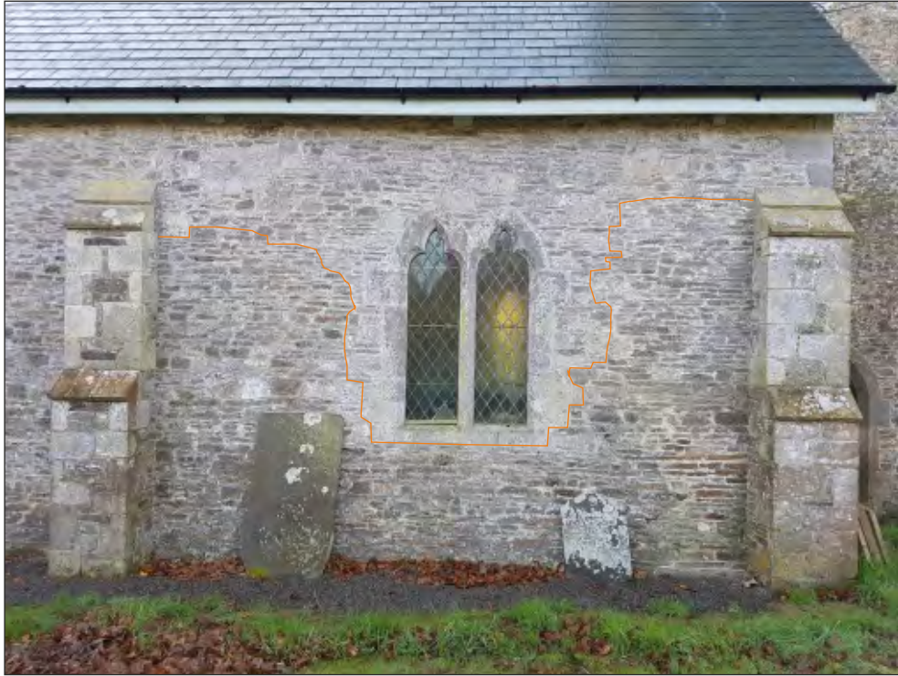
Pl. 18 General view of north elevation showing sections rebuilt in late 19th century. Looking south.
