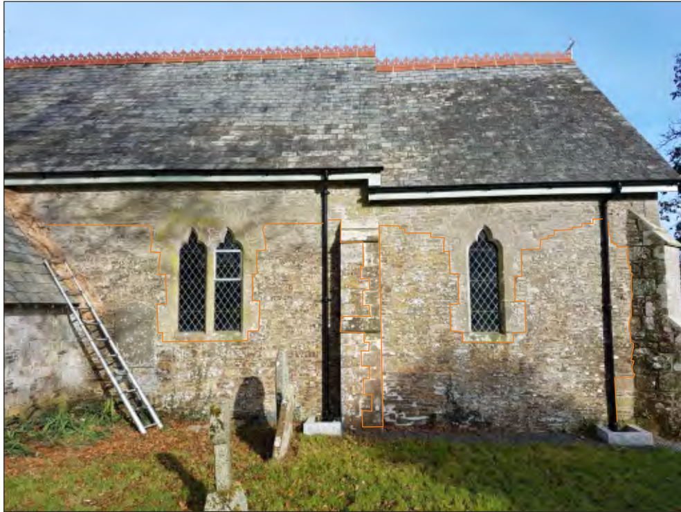
Pl. 14 General view of south elevation showing sections rebuilt in the late 19th century. Looking north.
