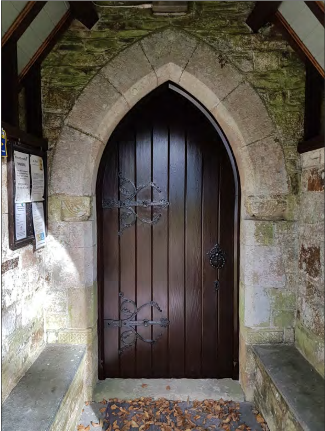
Pl. 3 General view of south doorway showing two Norman impost blocks (middle) and remains of capitals (bottom). Looking north.
