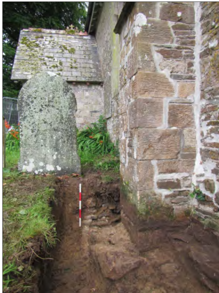
Pl. 9 General view of early foundation (111). 0.5m scale. Looking northwest.
