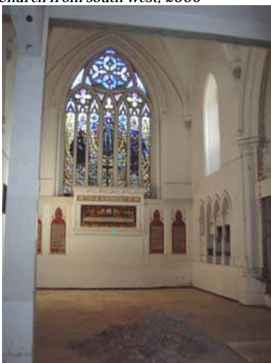
Interior looking east, 2006
