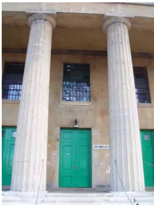
West front (doors to private flats), 2006
