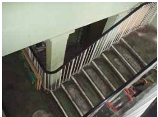
North west staircase (now a fire escape), 2006
