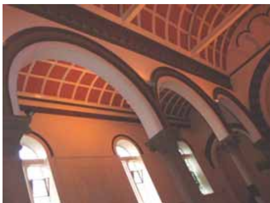
G.E. Street's nave arcading (1871-2)
