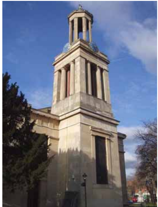
Church tower to east end of church, 2006
