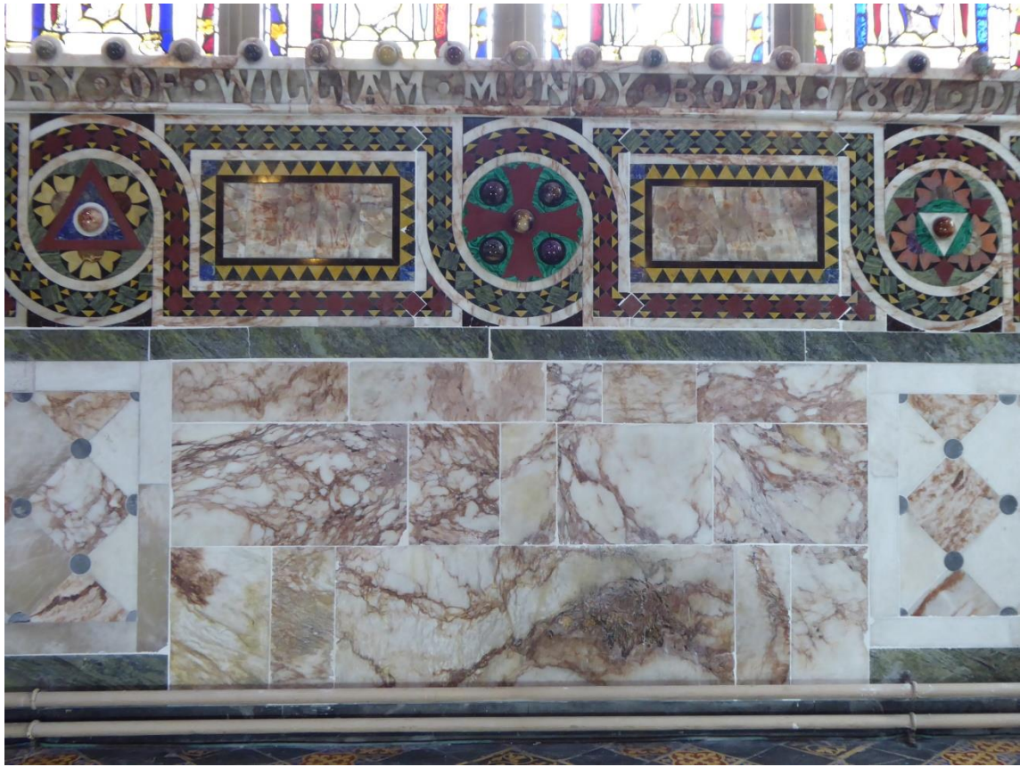
Figure 63 Pointing mortar before toning down
