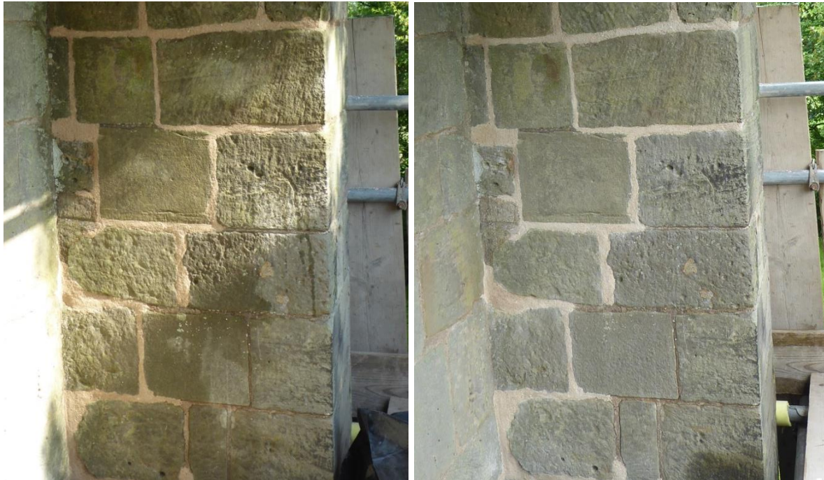
Figure 37 Re-pointing top coat mortar while still wet (left) and dry (right)
