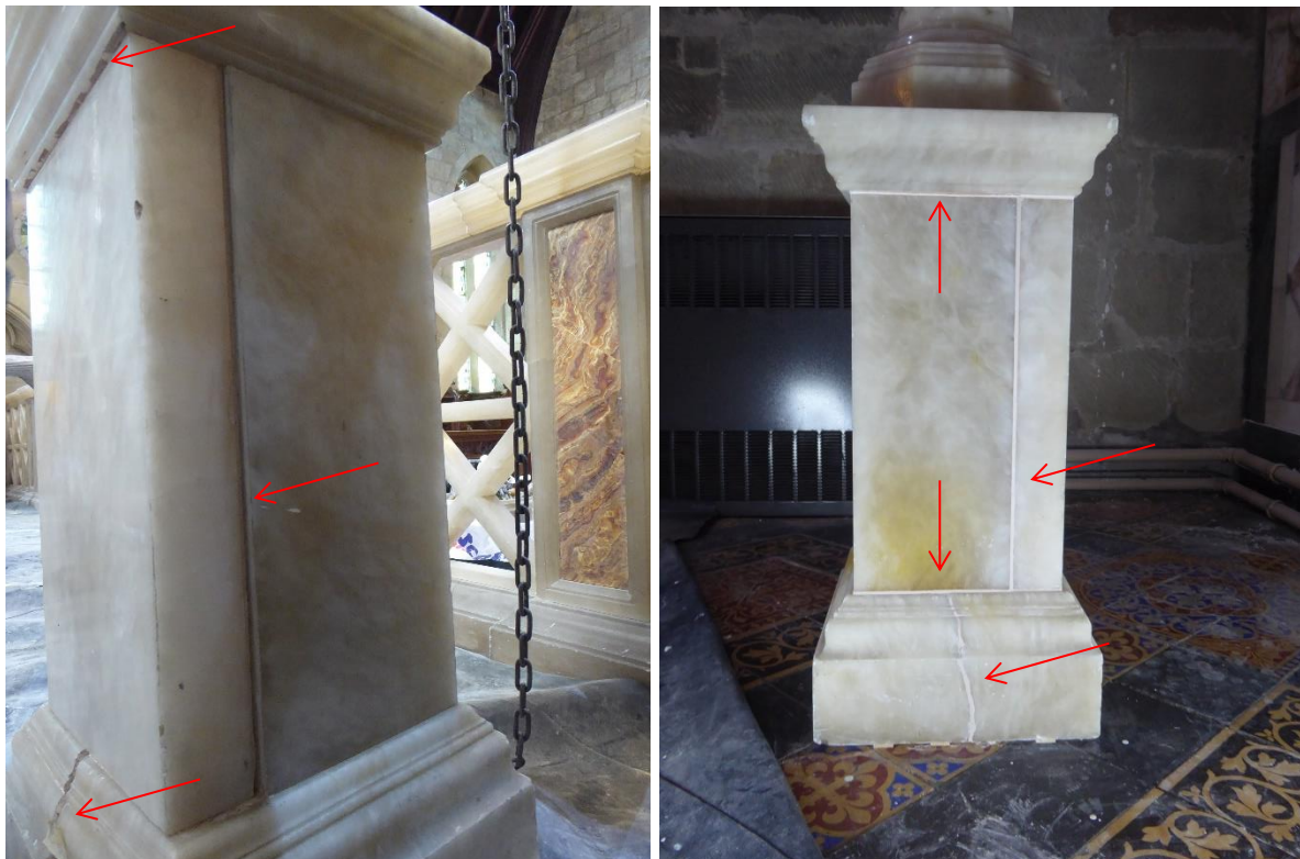
Figure 23 Plinth joints and cracks before raking out and after filling
