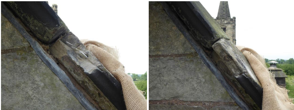
Figure 47 Pinning of failed previous mortar repair
