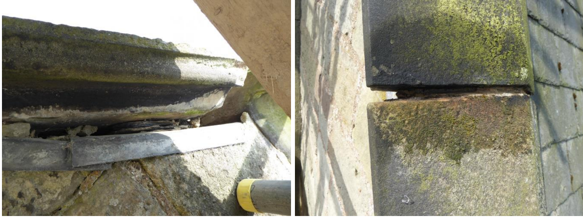
Figure 46 Removal of failed pointing mortar to coping stones
