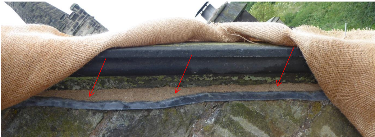
Figure 49 Top mortar coat for pointing works to the coping stones
