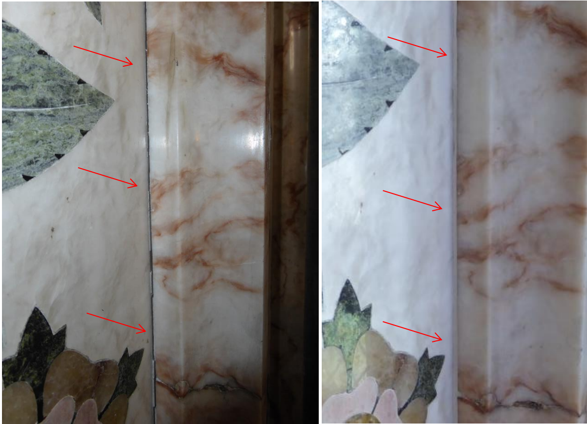
Figure 18 Joint before raking out and after repointing
