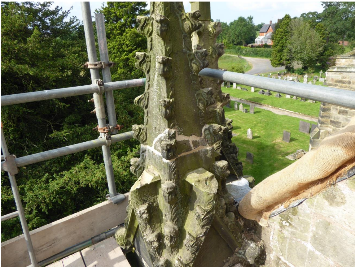
Figure 82 Final condition of pinnacle with pointing works
