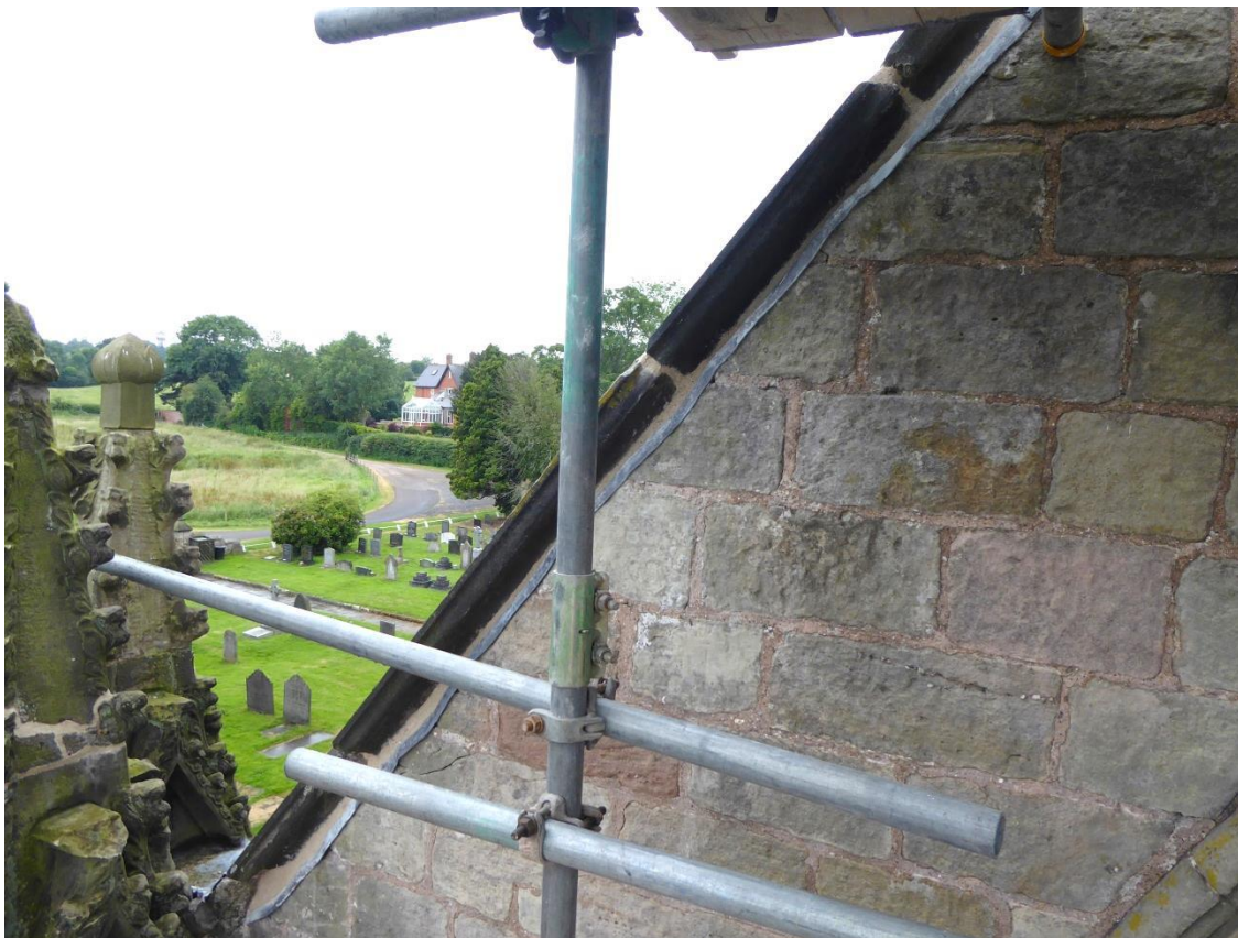
Figure 86 Pointing top coat to coping stones
