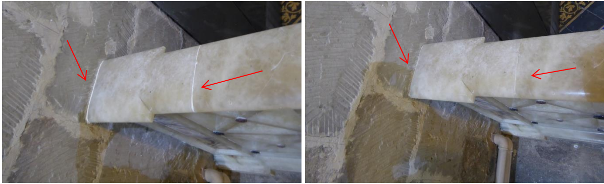
Figure 28 Pointing before and after toning down with water colours
