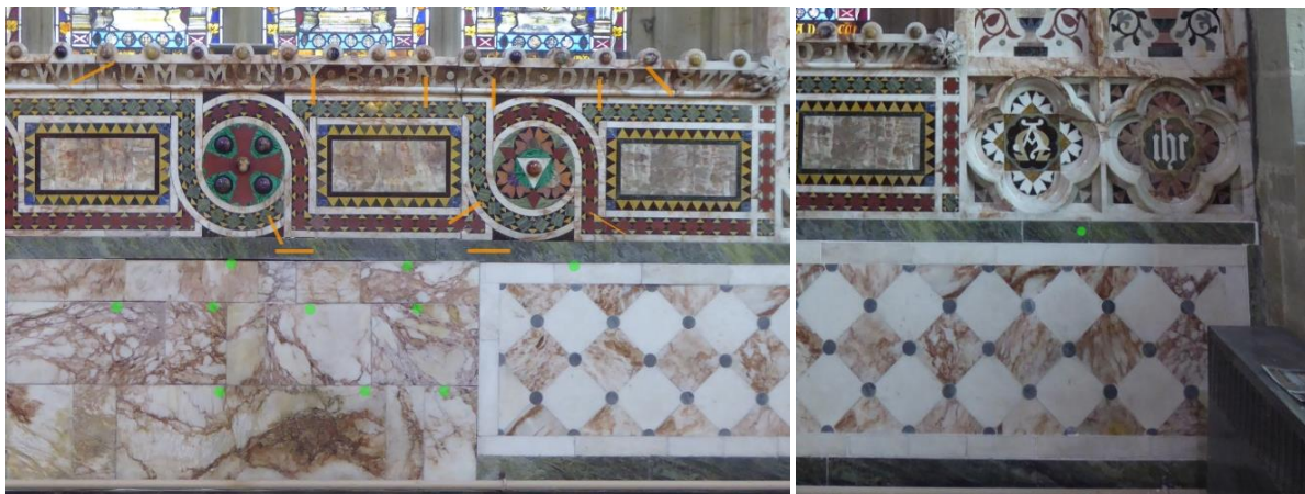
Figure 12 Location of pinning between stone blocks (orange) and pinning to wall (green)
