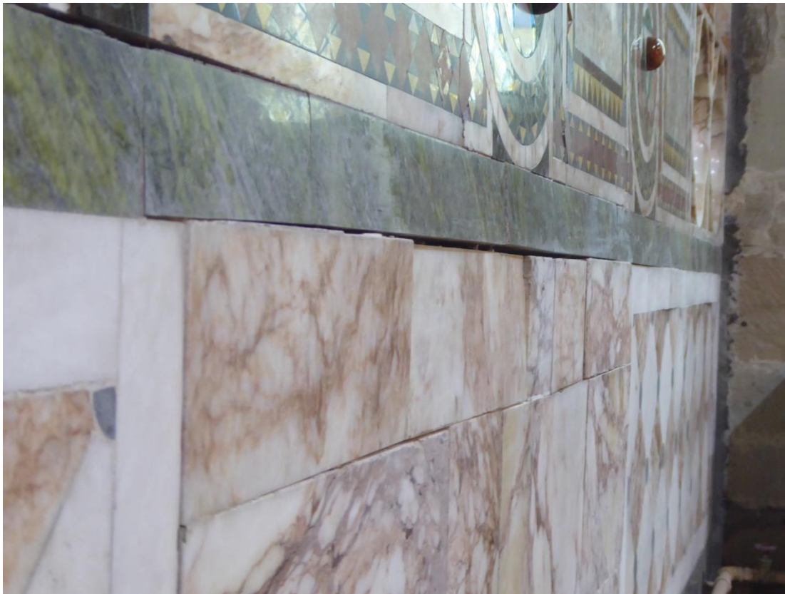
Figure 51 Initial condition of alabaster blocks to the central section
