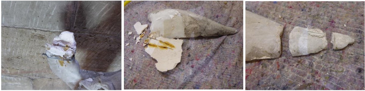
Figure 30 Dismantling of angel wing in three pieces
