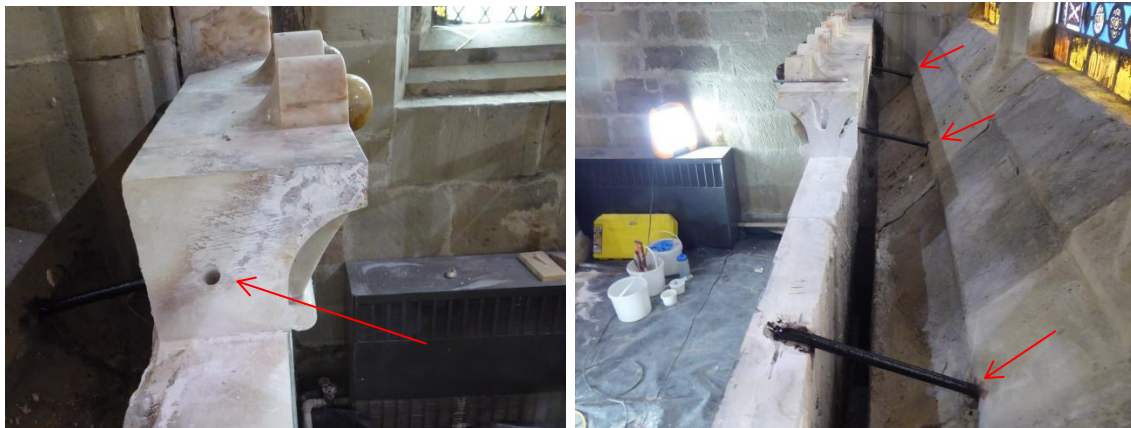
Figure 9 Pinning dismantled block and treated metal rods behind the reredos
