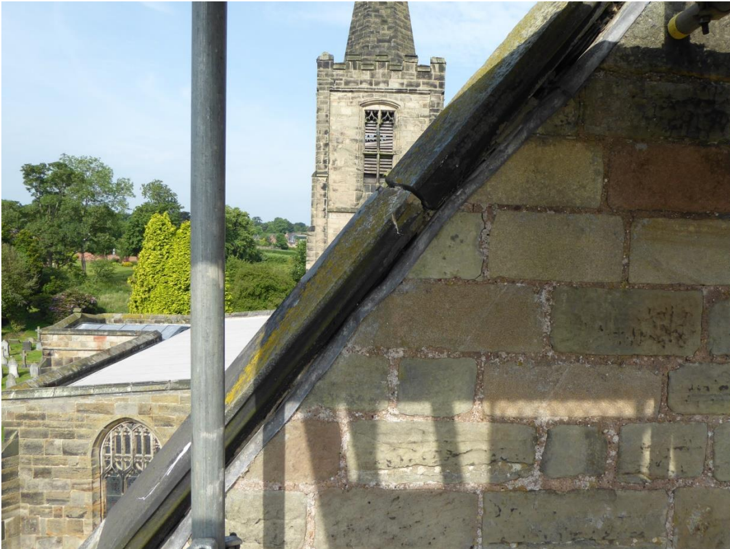
Figure 83 Initial condition of pointing to coping stones
