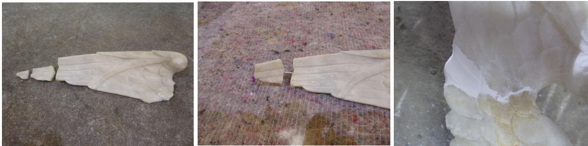
Figure 31 Pinning and re-fixing angel wing
