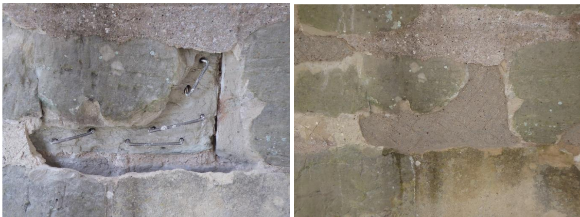
Figure 40 Preparatory armature and application of base coat
