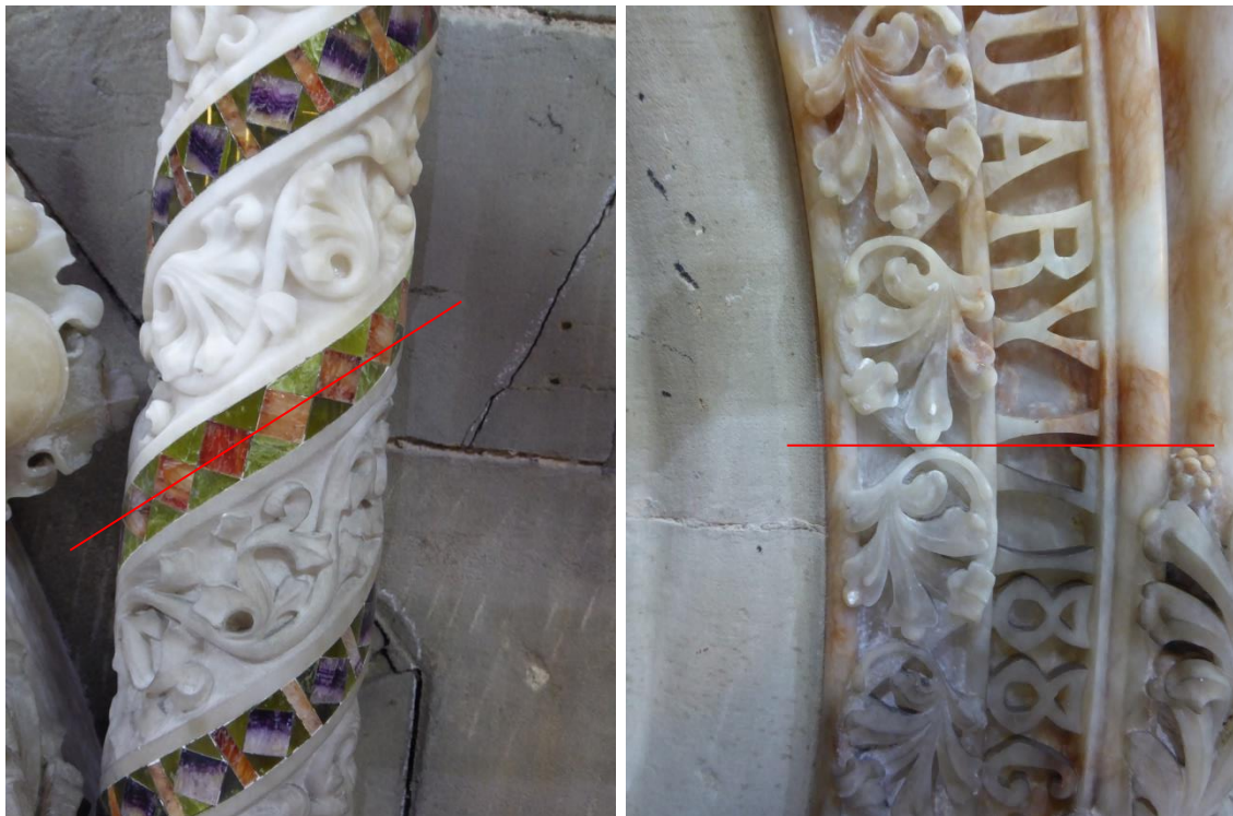
Figure 32 Examples of cleaned and uncleaned sections
