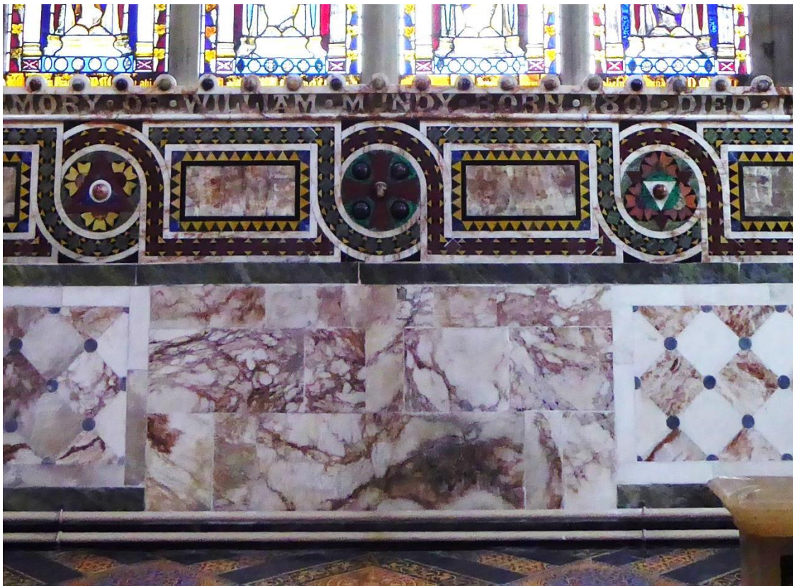
Figure 54 Final condition of central section
