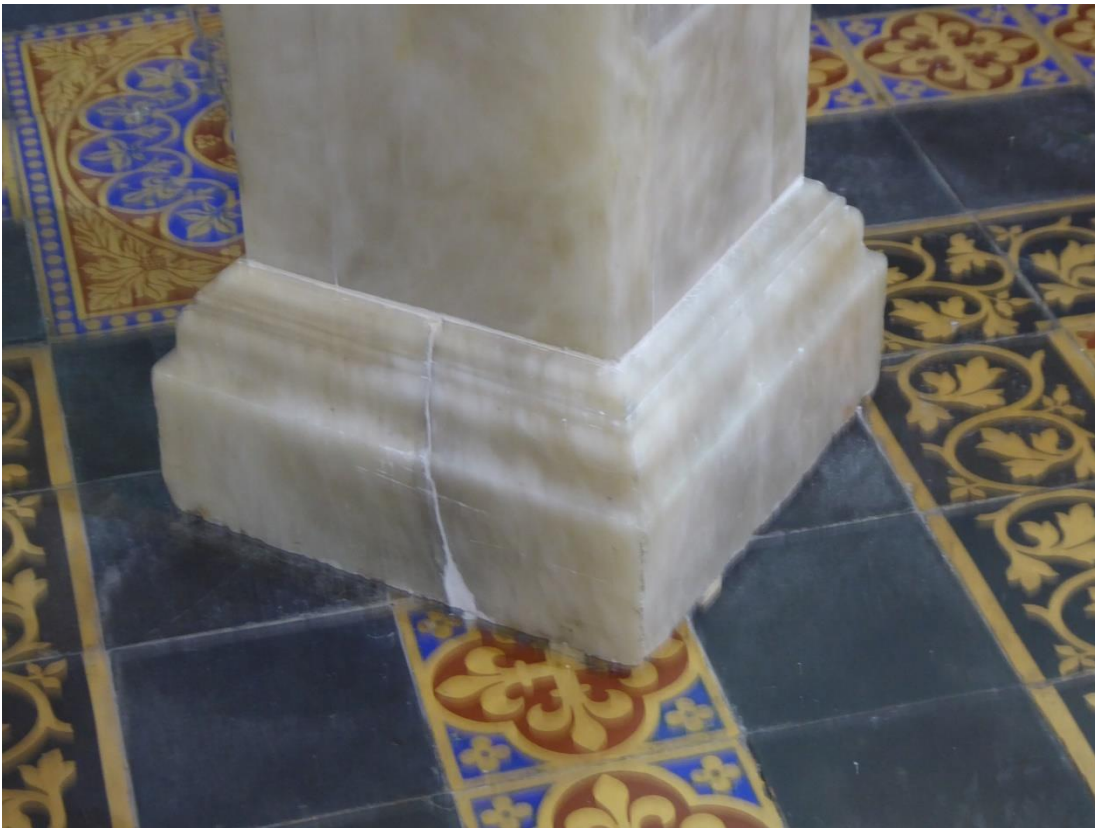
Figure 66 Crack condition after fixing and filling
