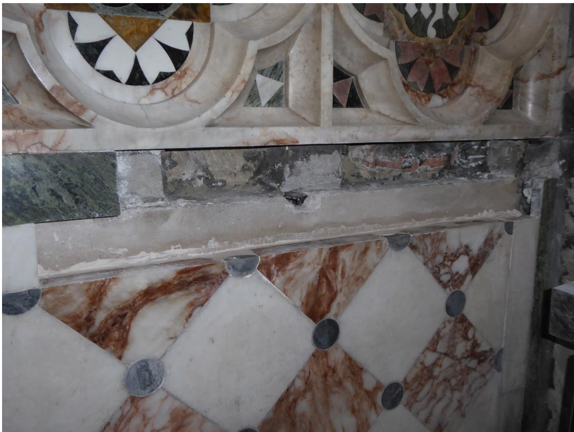
Figure 56 Dismantling alabaster and marble blocks to right area of reredos
