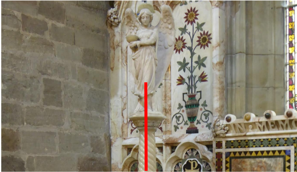
Figure 26 Location of the metal rod inside the angel and the column
