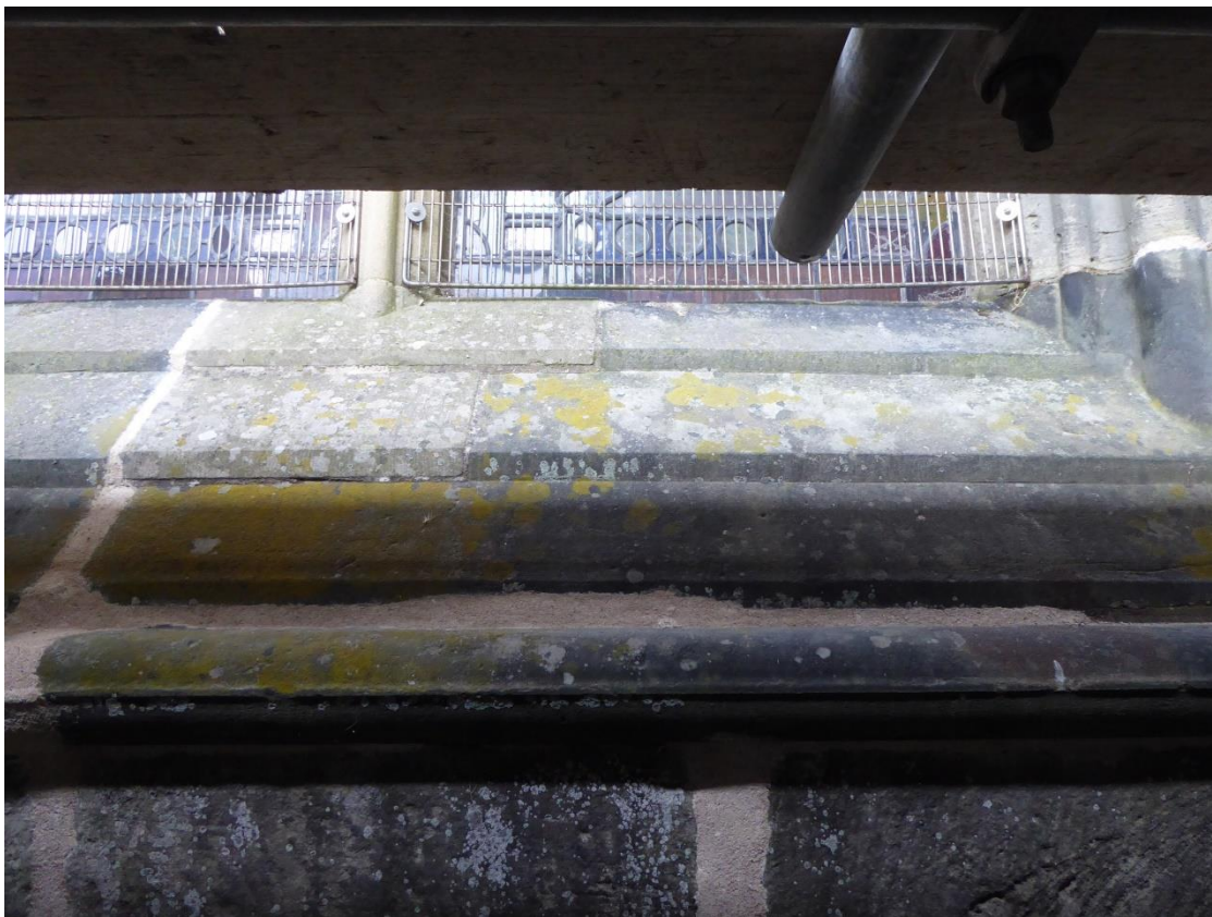
Figure 74 New pointing works to exterior wall
