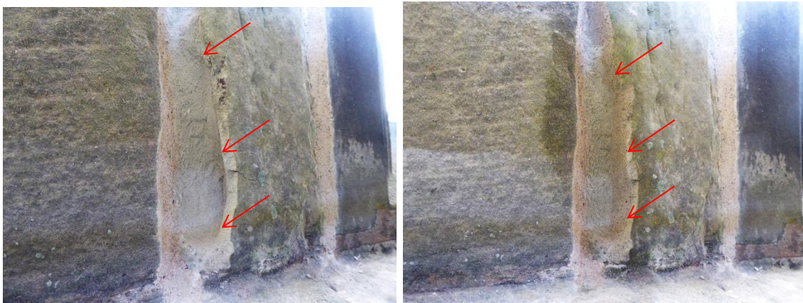
Figure 42 Before and after the capping repairs to stone
