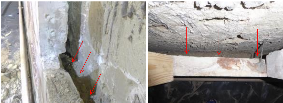
Figure 4 Debris to rear of reredos before and after removal
