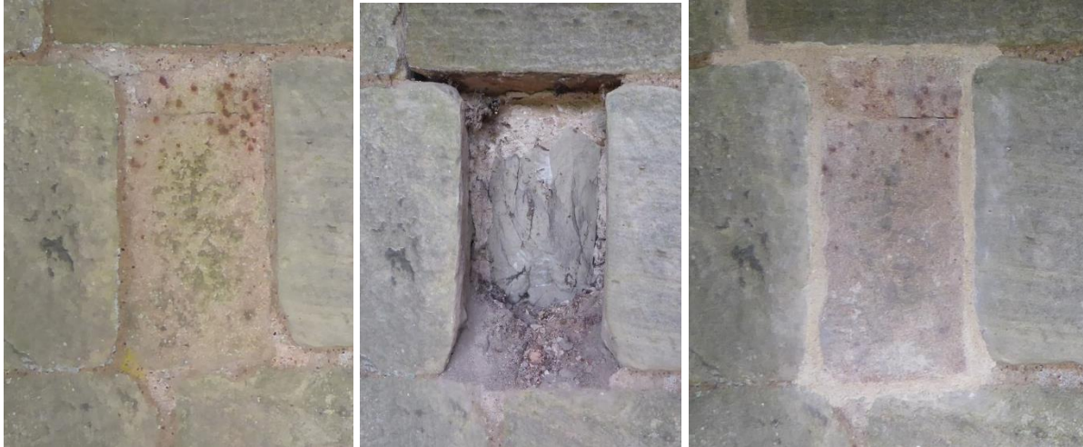
Figure 44 Dismantled block before, during and after relocation
