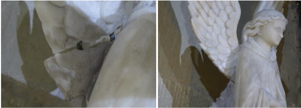
Figure 13 Angel wing before replacement of rods and after relocation
