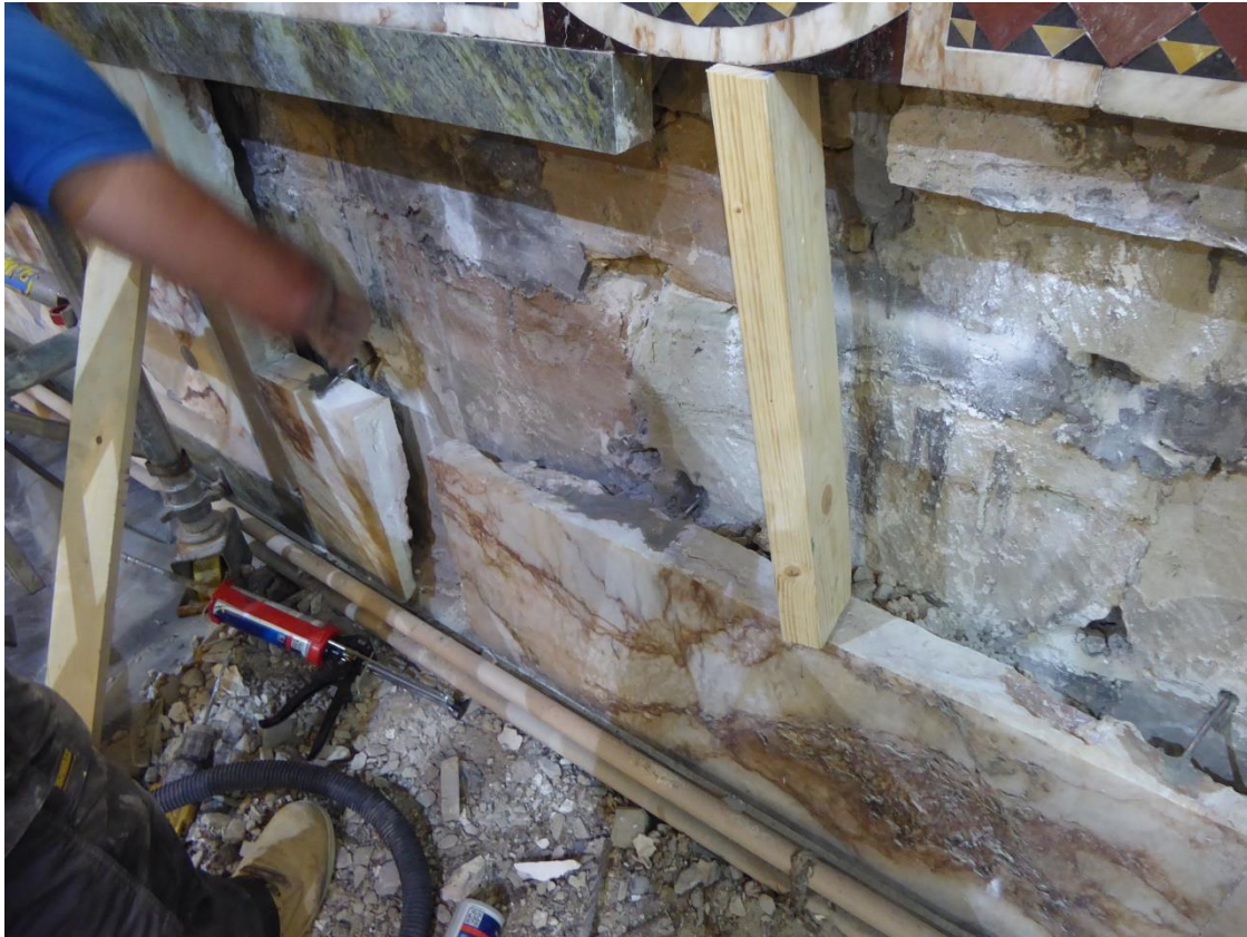
Figure 53 Fixing the alabaster blocks to the wall
