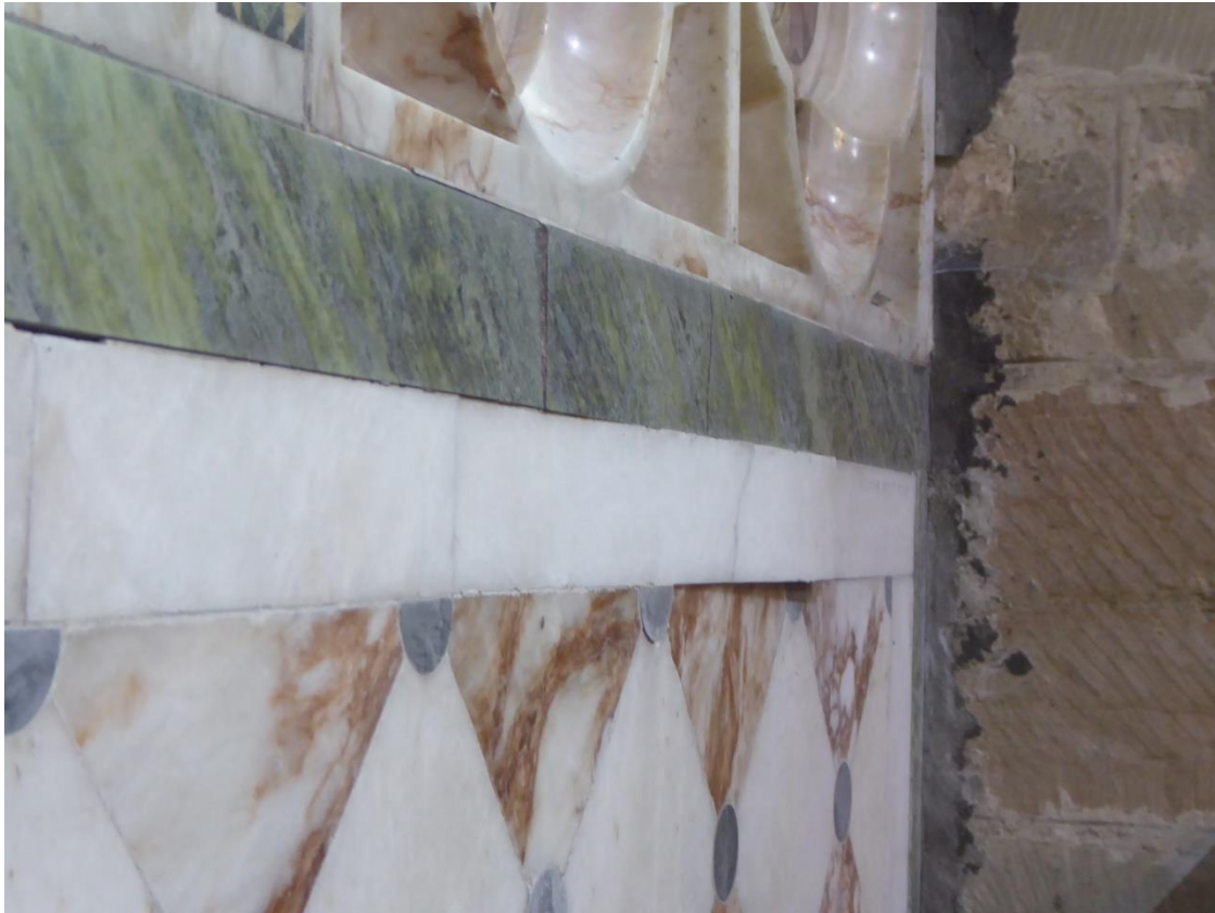
Figure 55 Initial condition of alabaster and marble blocks to right area of reredos
