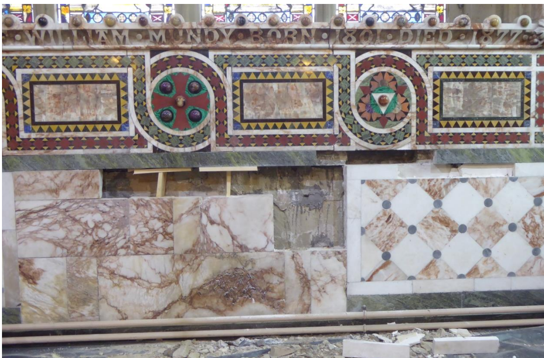
Figure 52 Dismantling of alabaster and marble blocks process
