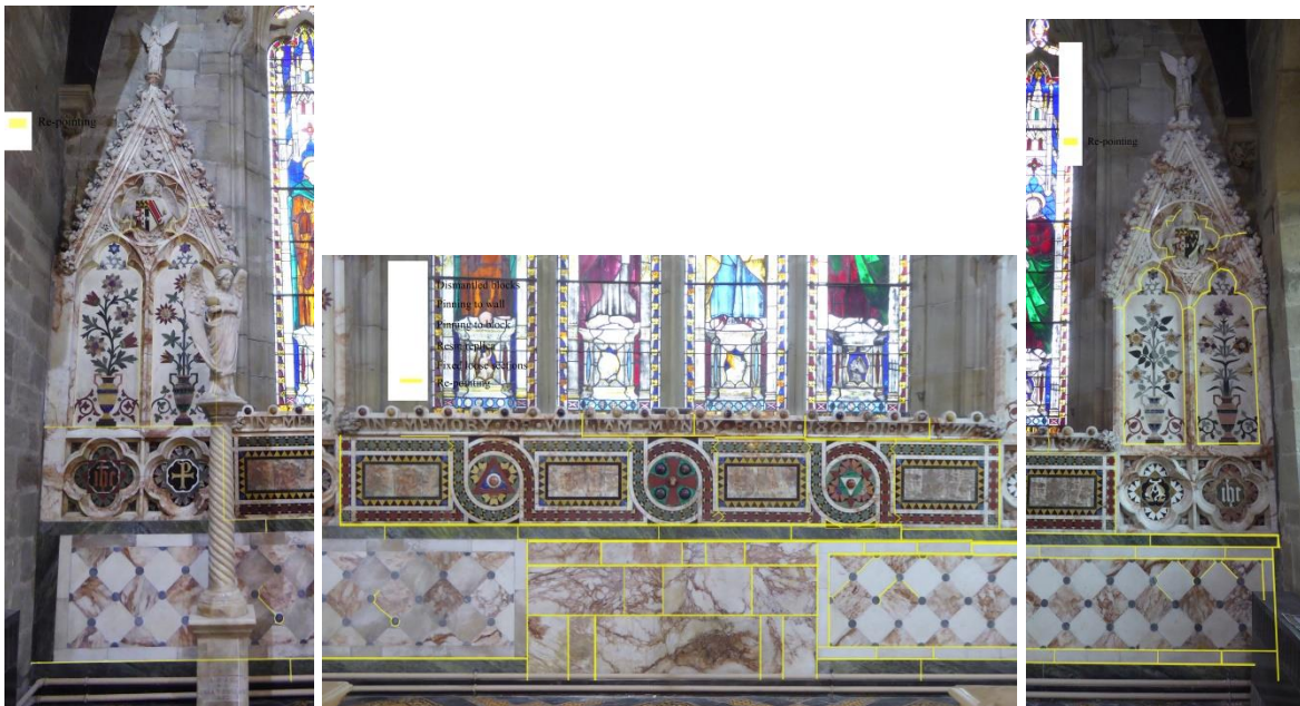
Figure 17 Location of the re-pointed joints
