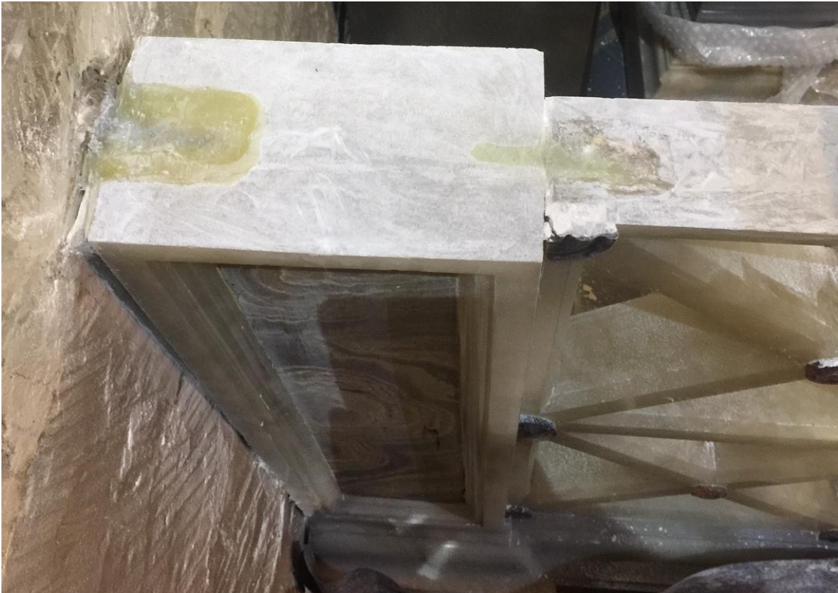
Figure 67 Replacement of two metal cramps and fixing with resin
