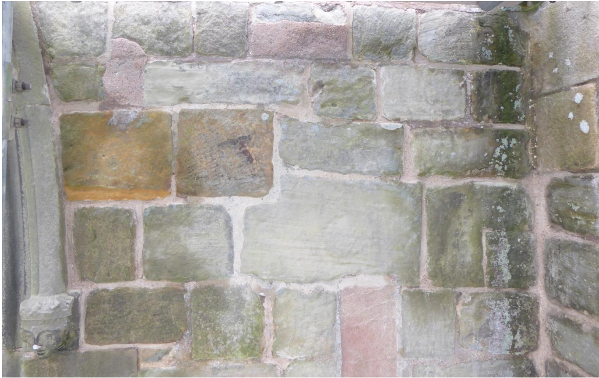
Figure 77 Application of first coat of pointing mortar to exterior wall
