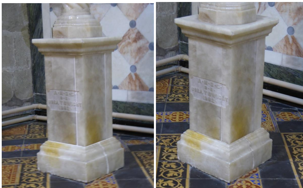
Figure 25 New pointing before and after the colour retouching
