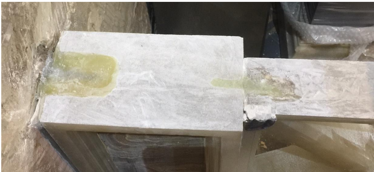
Figure 27 Replacement of ferrous cramps for stainless steel cramps and polyester resin
