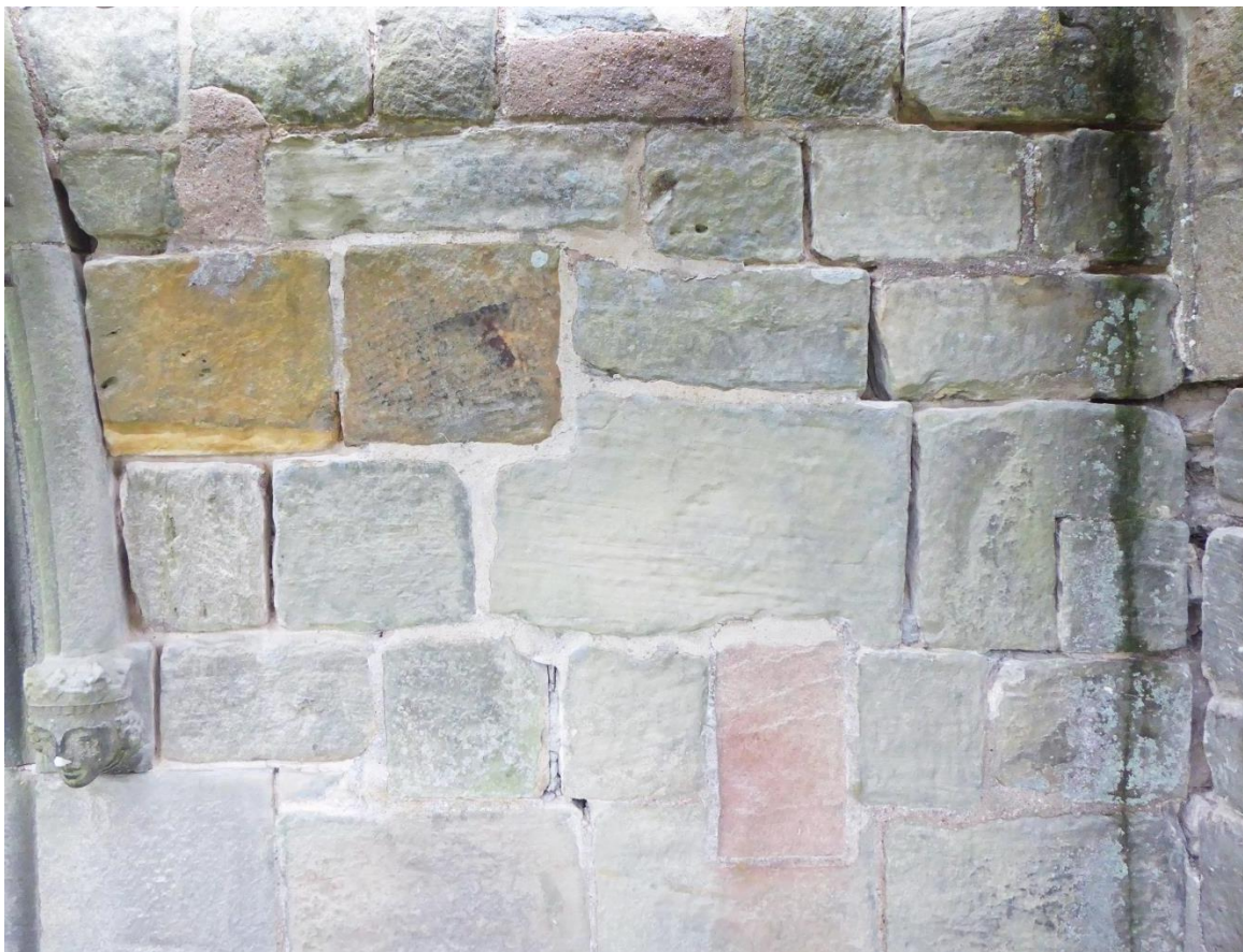
Figure 76 Raking out of failed pointing mortar
