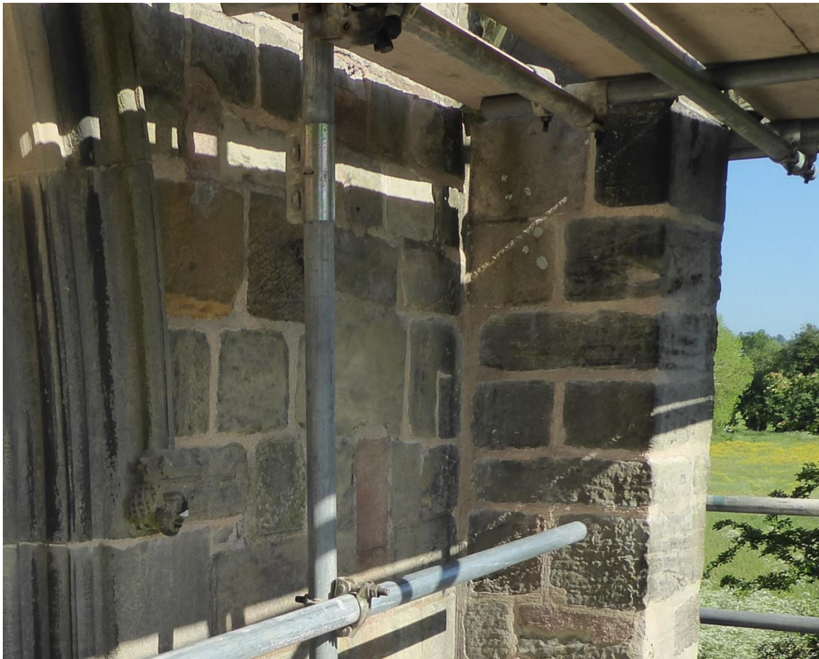
Figure 78 Application of pointing top coat to exterior wall
