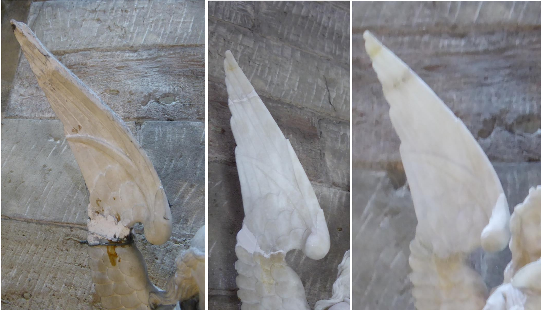
Figure 70 Initial, during process and final condition of the angel wing to the vestry door
