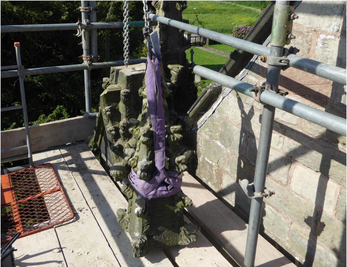
Figure 79 Dismantling top section of pinnacle
