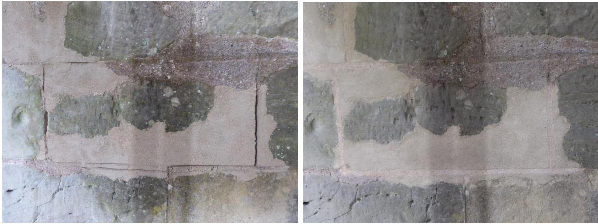
Figure 41 Application of top coat and final mortar repair with pointing lines
