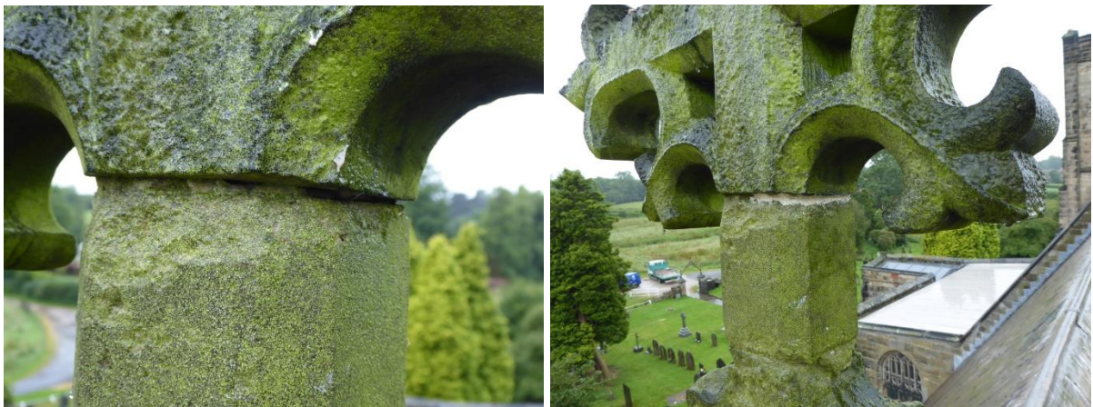
Figure 50 Injection of polyester resin to joint of the cross
