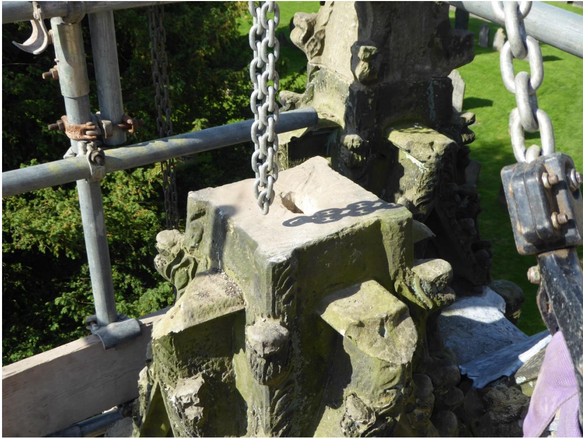
Figure 81 Cleaning of joint from previous mortars and resins
