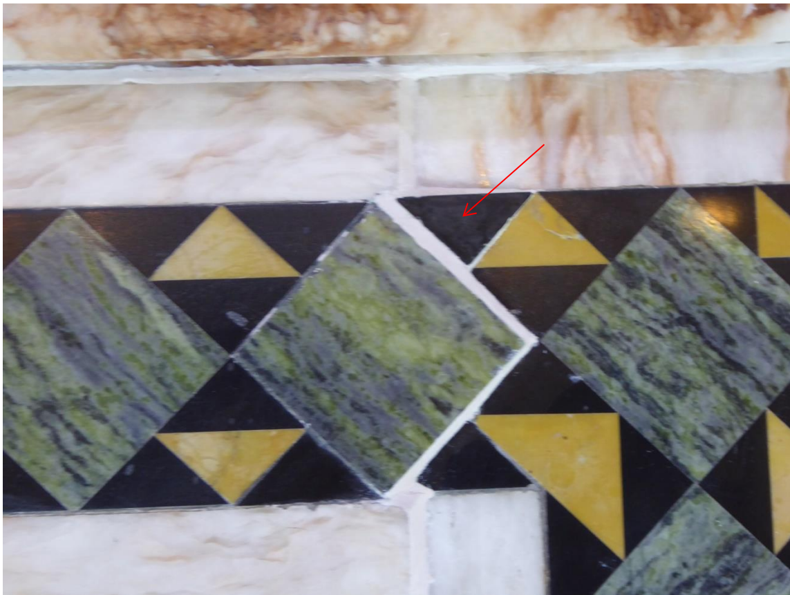
Figure 60 Fixing replica piece to reredos
