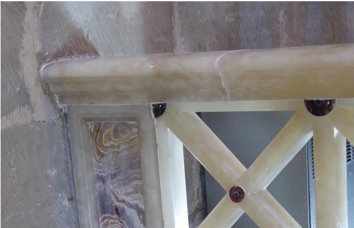
Figure 68 Relocation of block and new pointing
