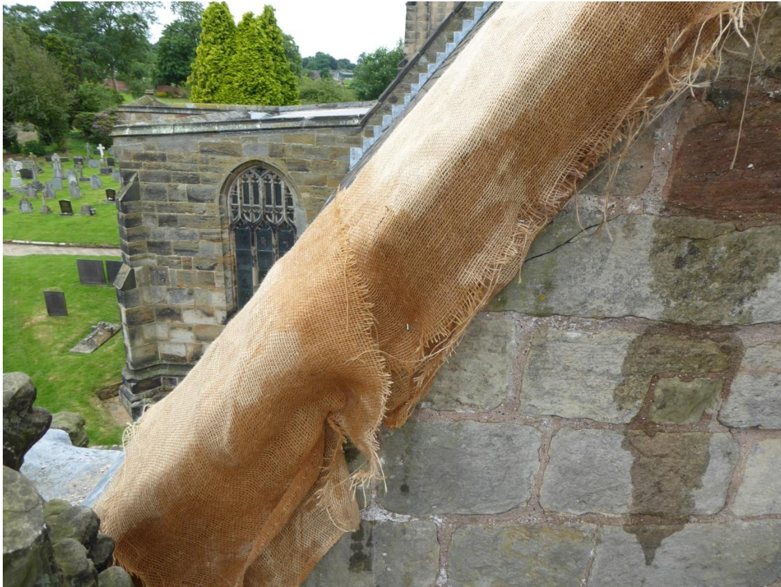
Figure 85 Wetting and protection with hessian of new pointing mortar
