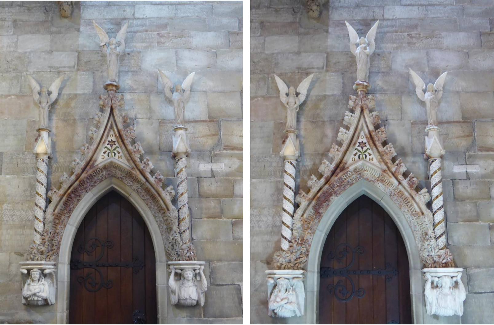
Figure 69 Initial and final condition of the vestry door
