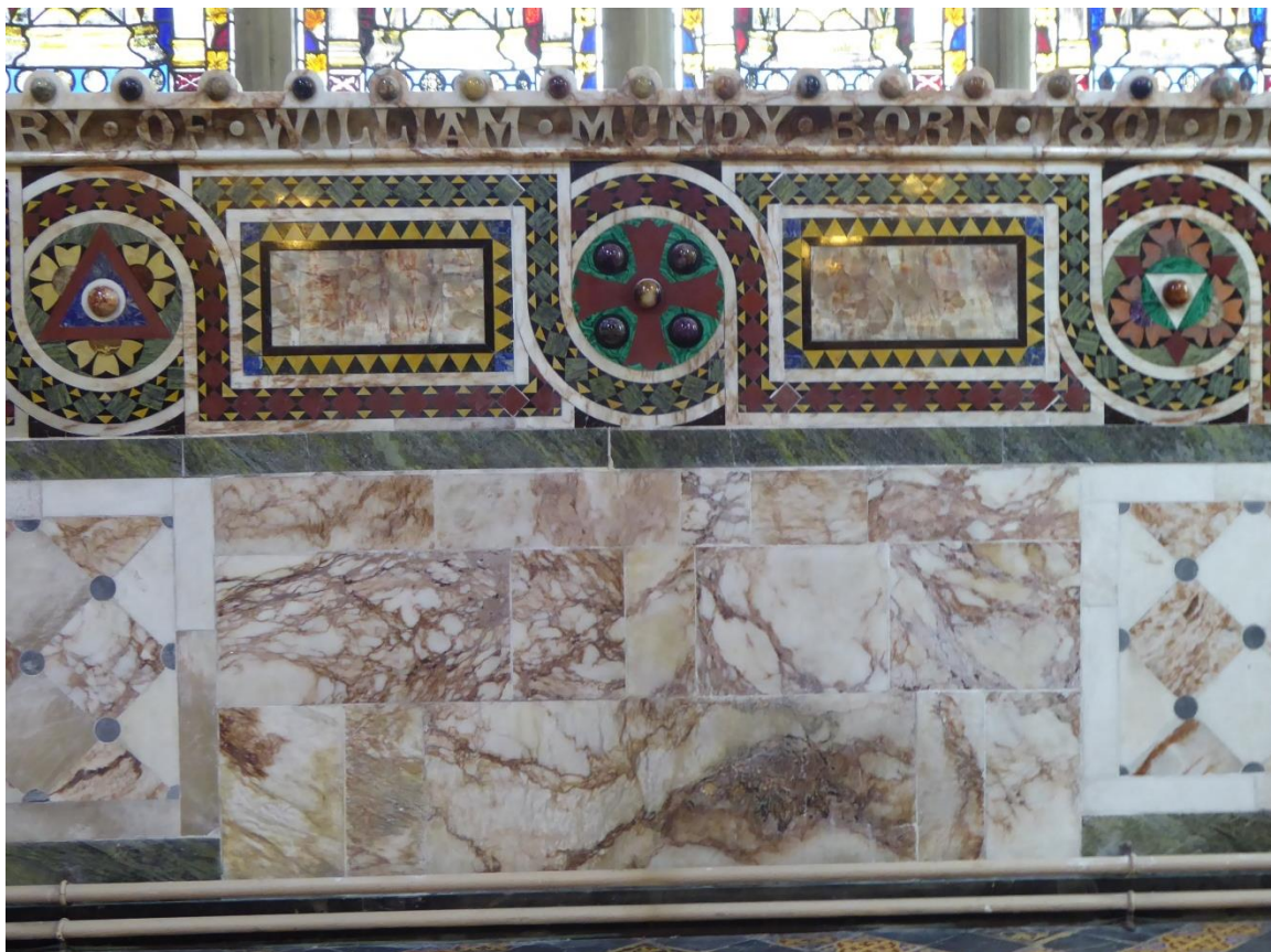
Figure 64 Pointing mortar after toning down
