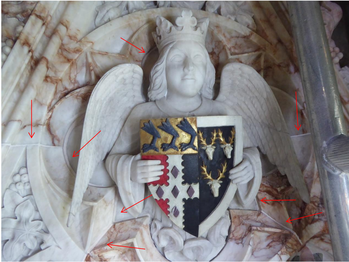
Figure 61 New pointing to reredos
