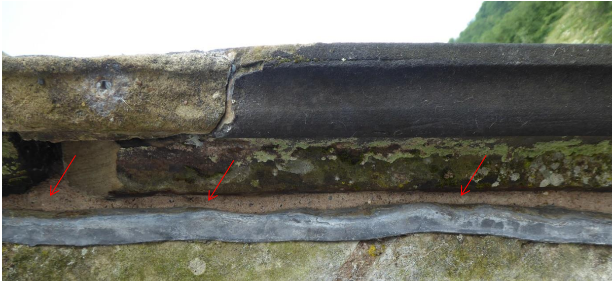
Figure 48 Base mortar coat for pointing works to the coping stones
