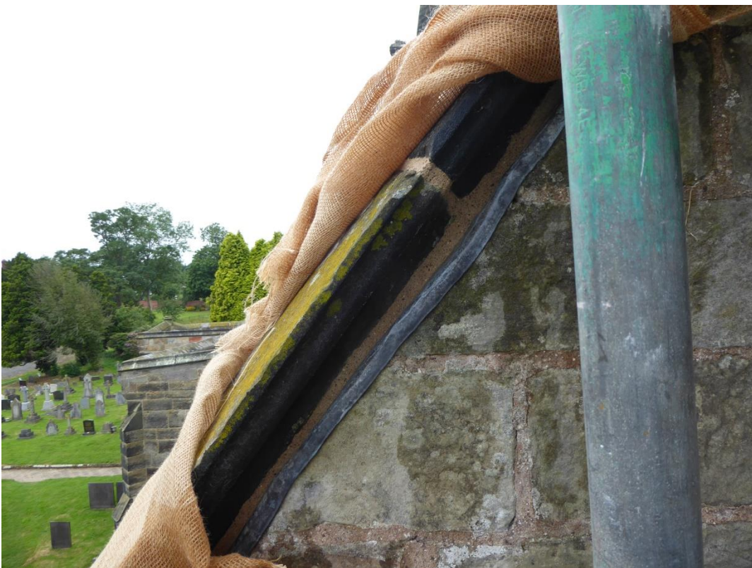
Figure 84 Pointing base coat to coping stones
