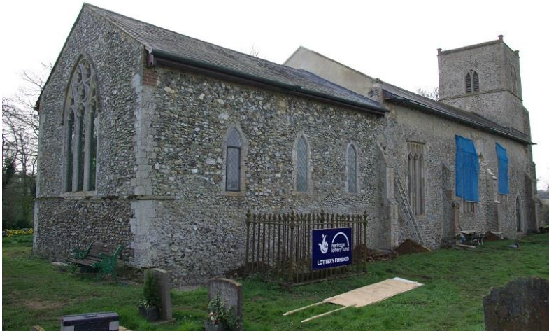
Plate 7: Work in progress N of church, looking SW
