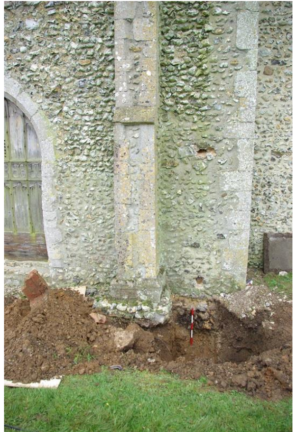
Plate 10: Trench 7; buttress footings at NW corner of nave, 0.5m scale
