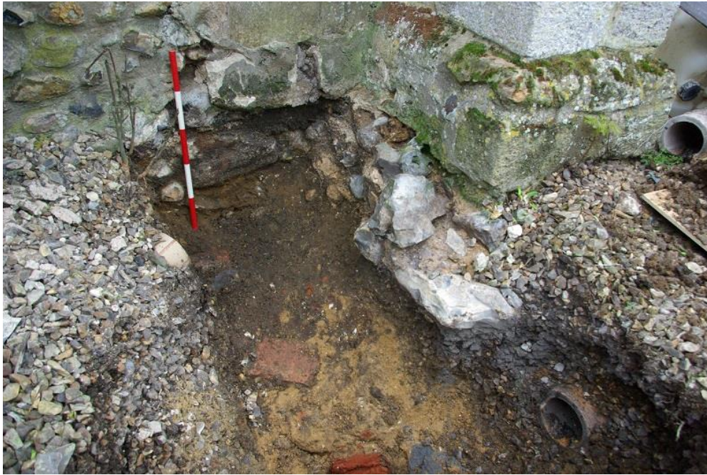
Plate 3: Trench [2]; nave and buttress footings, looking NNE, 0.5m scale
