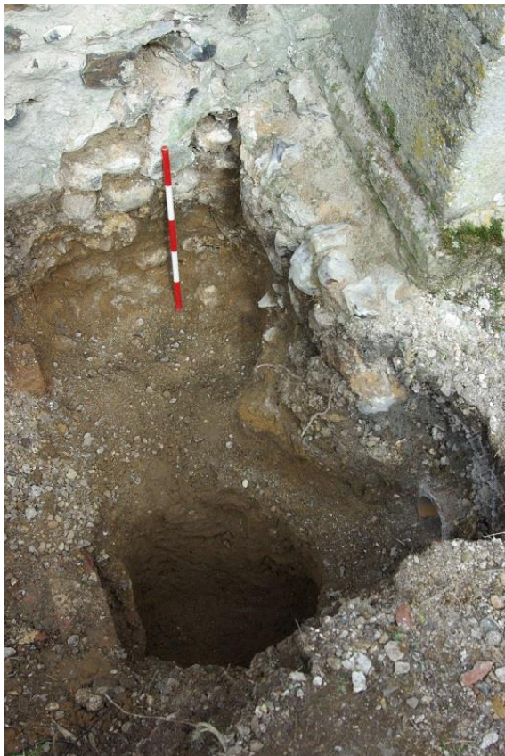
Plate 4: Trench [3]; nave and buttress footings, looking NNE, 0.5m scale
