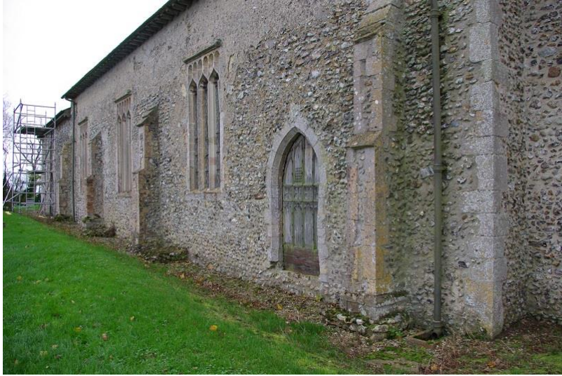
Plate 6 'Dry area' at N side of church prior to work, buttress footings visible, looking SE,
