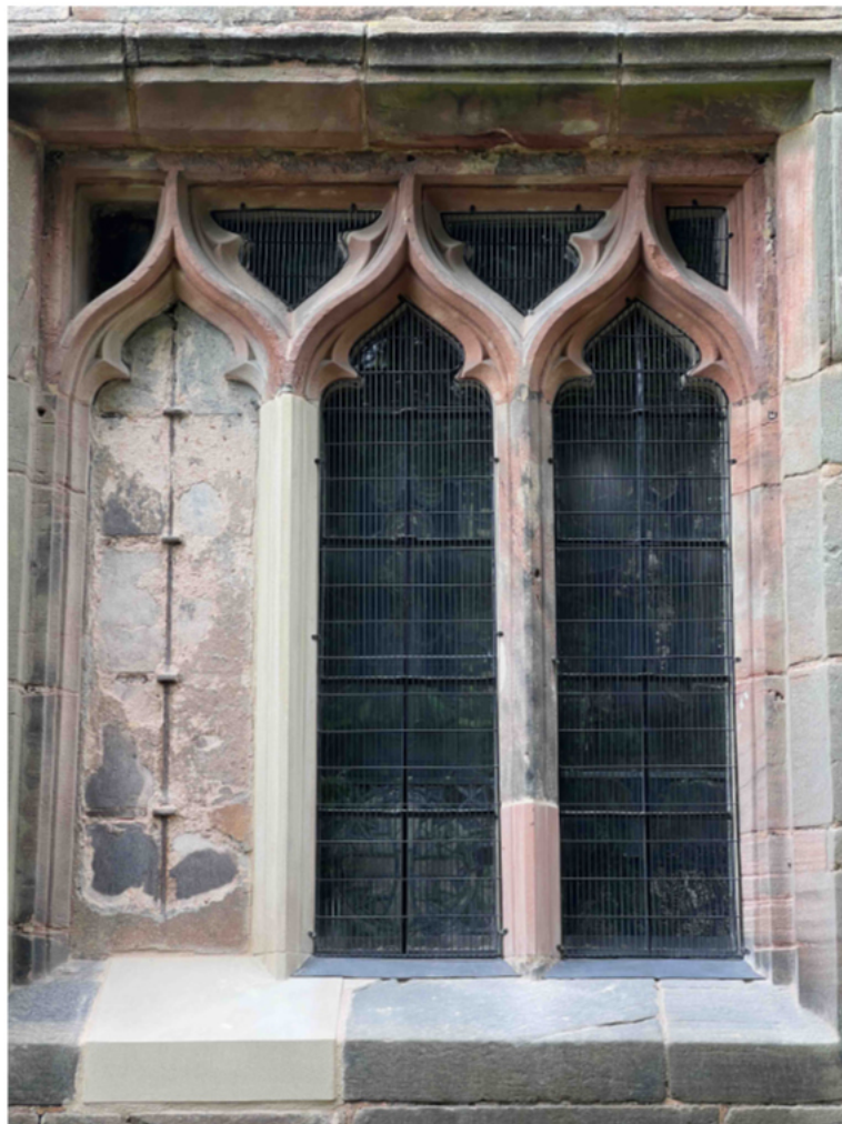
Above. sII. Exterior view of glazing. Before and after conservation.
