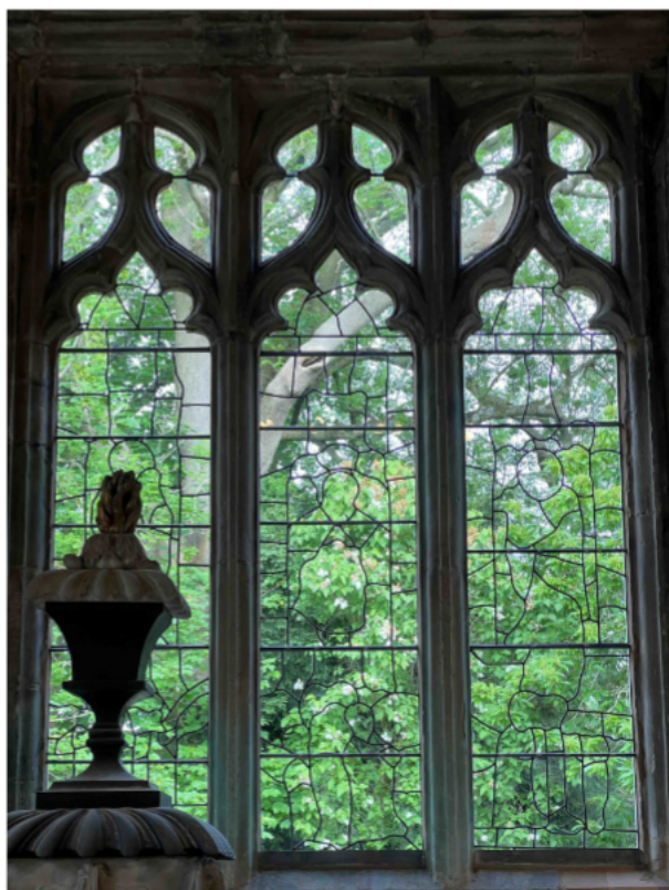
Above. sII. nII. Interior view of exterior secondary glazing prior to installation of the stained glass.
