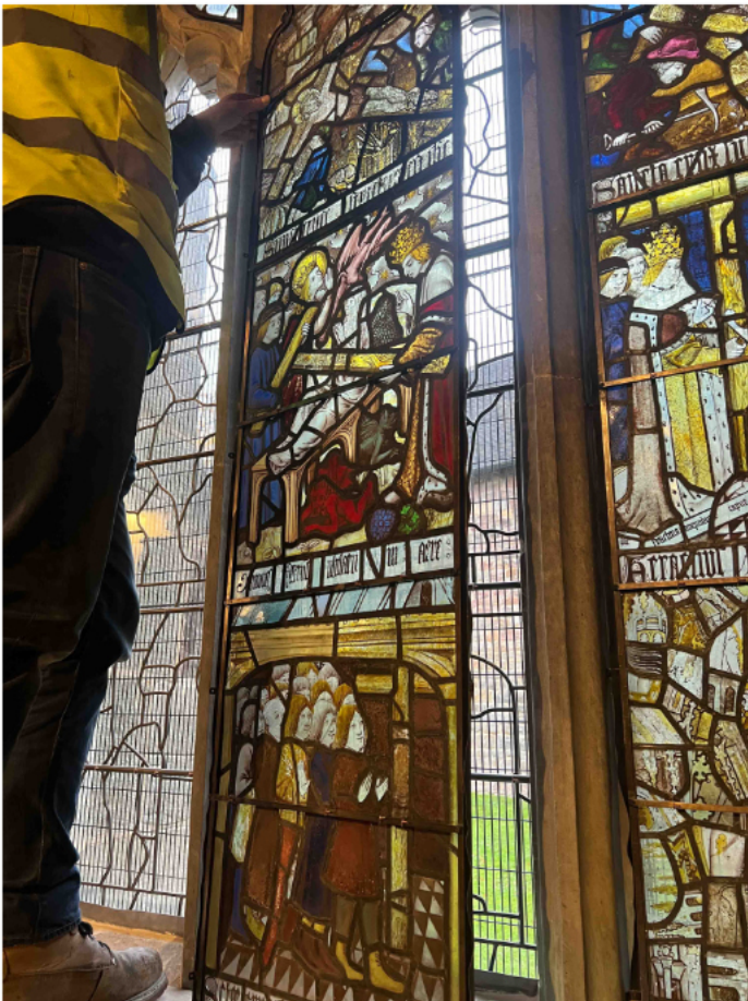
Above left. Installation of stained glass in bronze frames.
