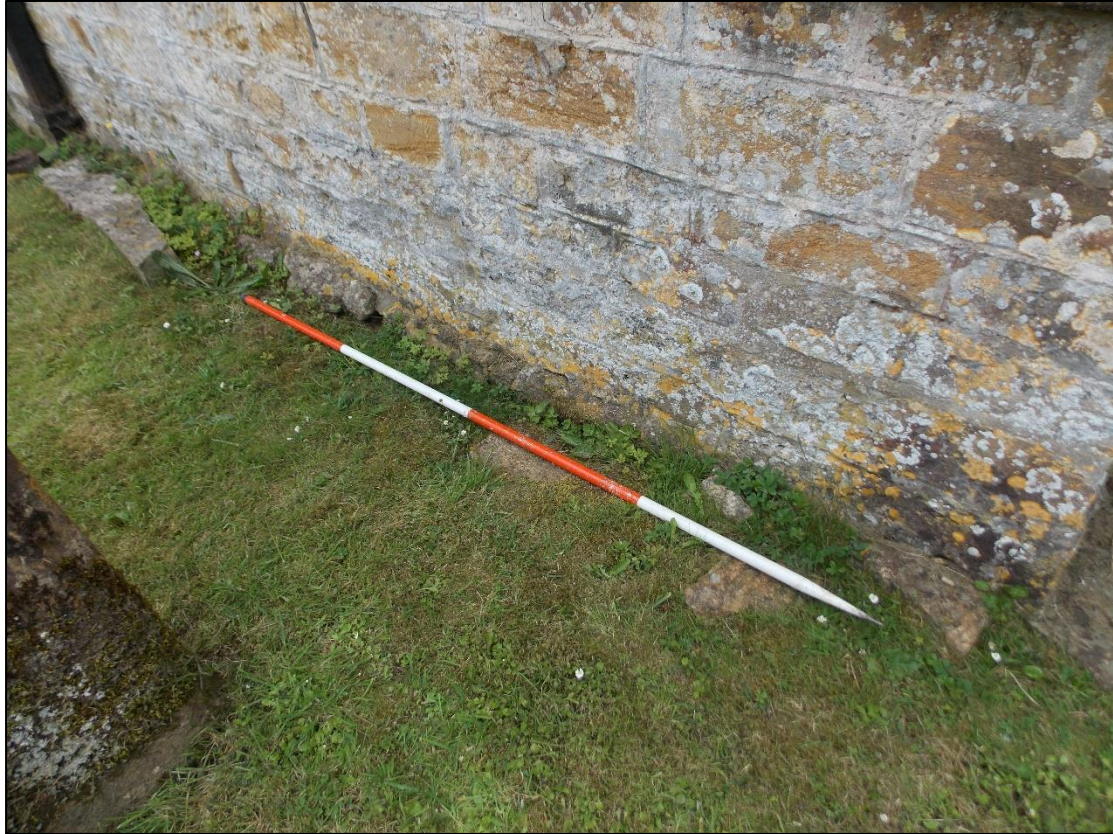
Figure 10. Offset footings on N Transept wall: facing SE, 2m scale.
