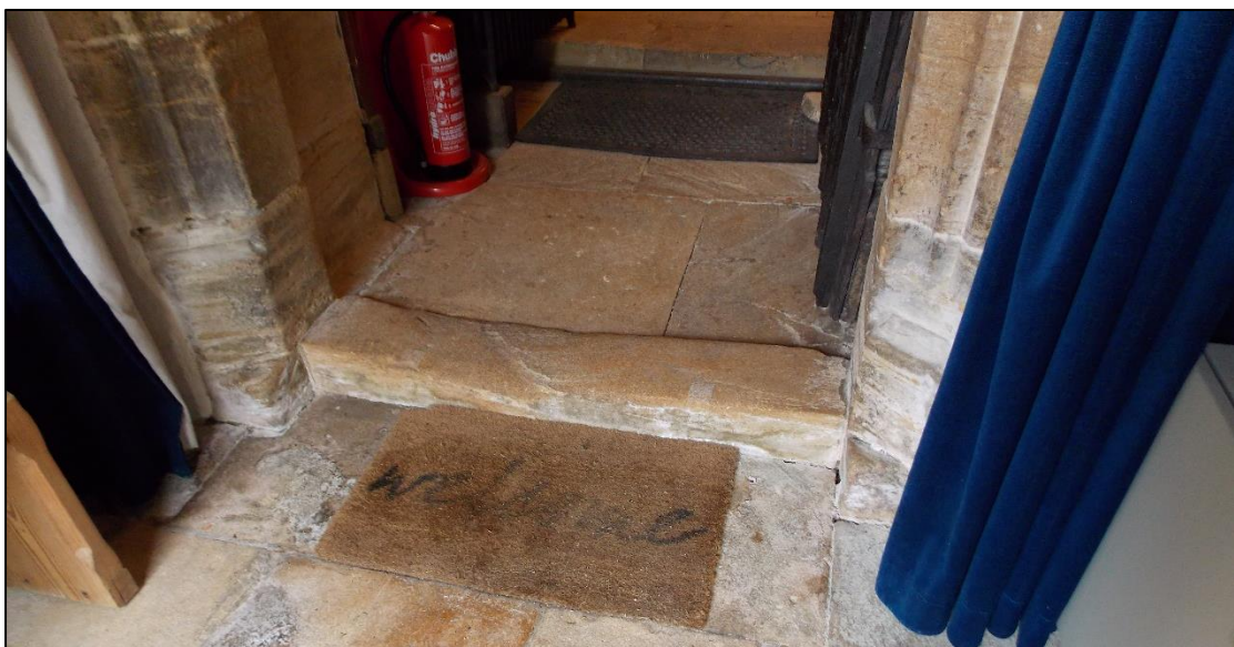
Figure 6. Worn Ham Stone step: facing SE
