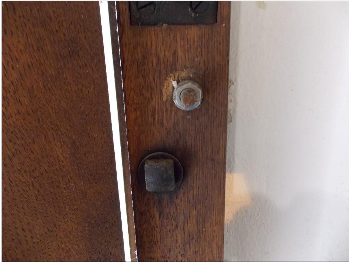
Figure 3. Fixings on timber framework
