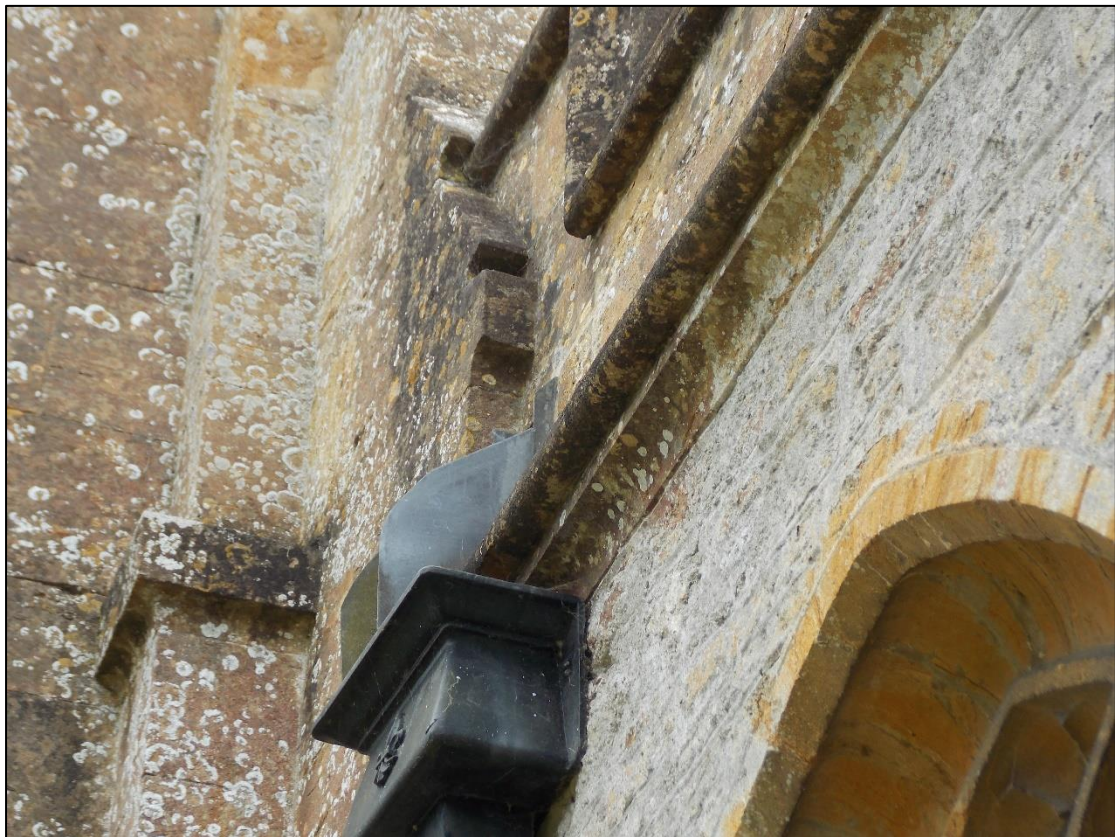
Figure 7. N Transept Parapet, constructed around Tower Buttress: facing E.
