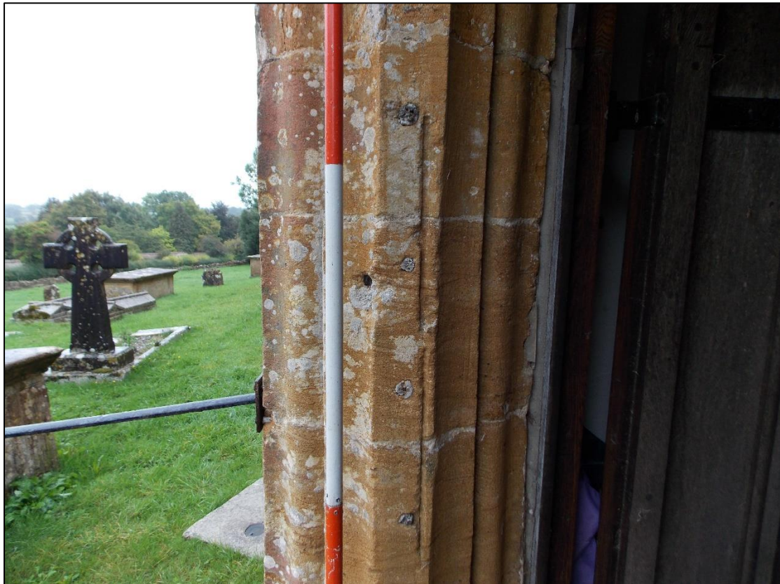
Figure 4. Wood dowels set within jambs, E side of porch entrance: facing E, 0.5m scale
