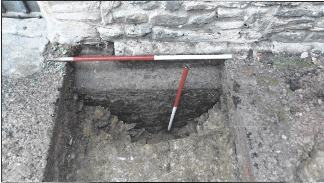
Figure 8. Chamfered plinth course/offset footings (105) : facing E, 1m scales.
