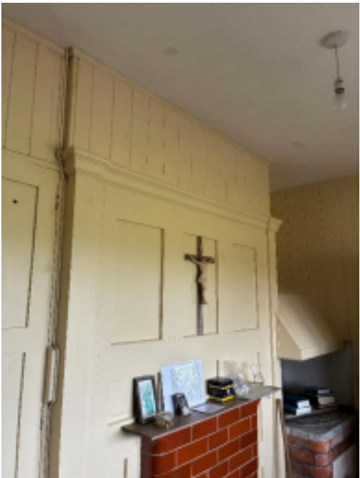
KITCHEN New location for 1800W heater Surface wiring from intake board to left
