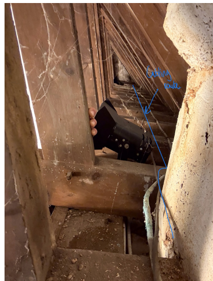
Cabling route through eaves at wallplate
