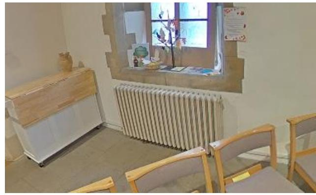
In order to improve the insulation directly behind the radiators, a reflective panel can be installed. This helps to make sure more of the heat from the radiator goes into the space and requires less overall heating from the boiler to achieve the set point. There are a wide variety of reflective panels for installing behind radiators on the market. It is recommended that these panels are installed behind all radiators within the building.
