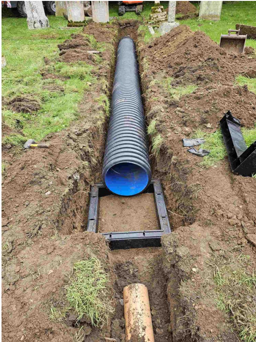
East soakaway 450mm diameter perforated Twinwall pipe in situ with 150mm plastic pipe from north drains. Looking east prior to back filling.
