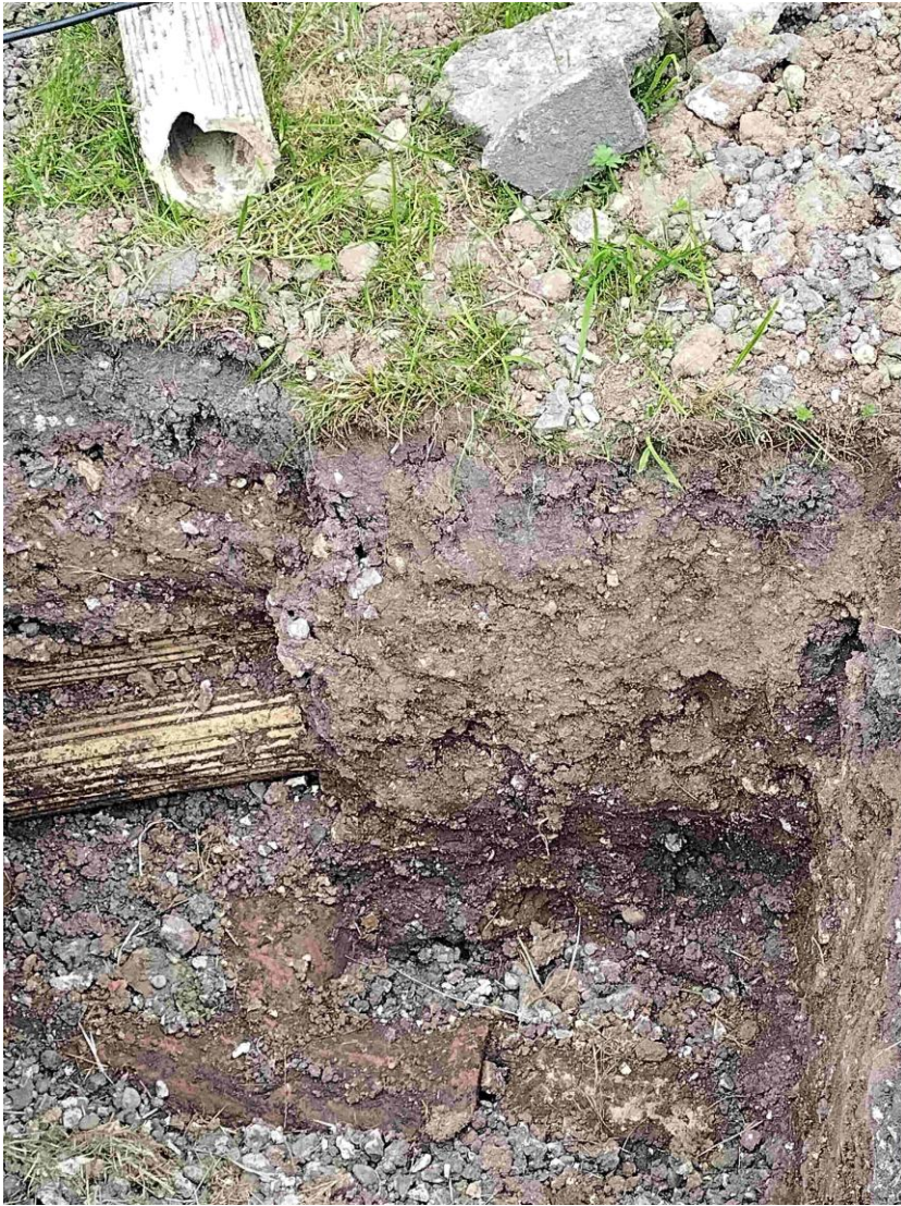
Previously disturbed layers at land drains and early form of socketed drain pipes in white clay with later red clay pipes not salt glazed.
