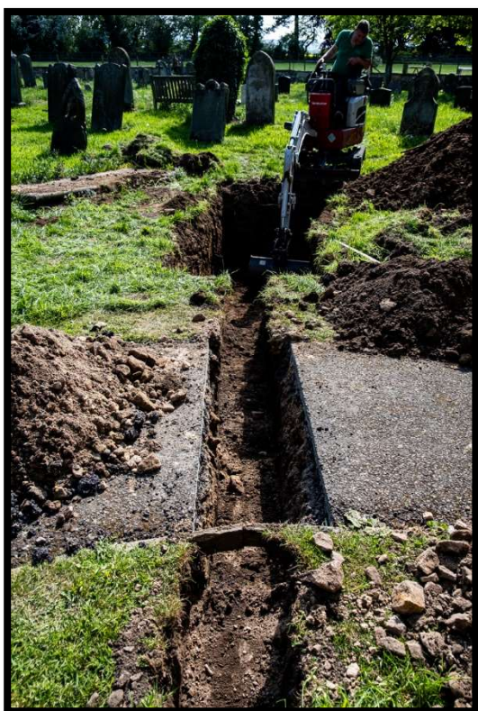
Fig 8 Drain cut from porch, through path, to soakaway (Whorlton May 25-9)
