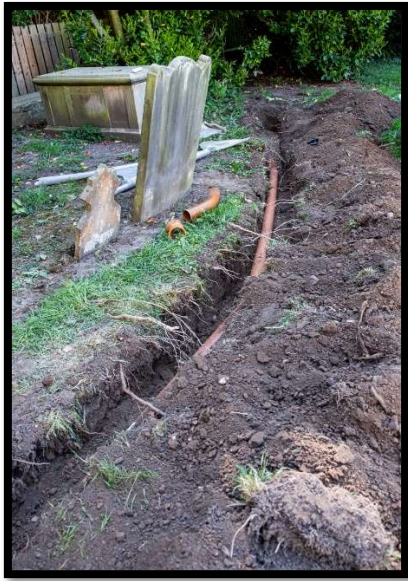
Fig 16 S side overflow pipe in place (Whorlton May 25-35)
