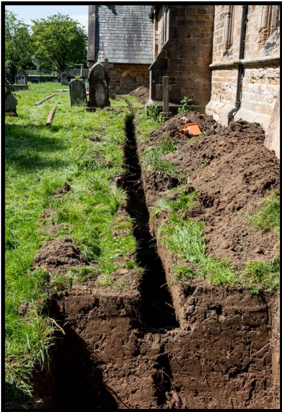
Fig 3 Drainage trench on South side from soakaway (Whorlton May 25-1)
