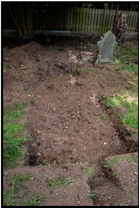
Fig 6 S side drain and soakaway cuts backfilled (Whorlton May 25-18)
