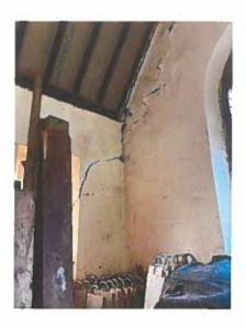
Photo 2 - Severe structural cracking around the east elevation south window (internal)
