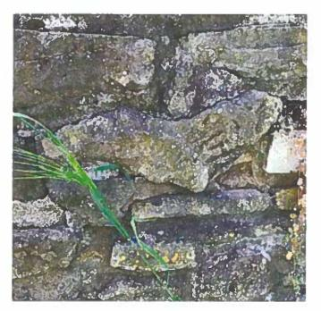
junction between the RHS pier and stone wall has an open joint indicating some settlement in the structure. Further south this boundary is formed with a split chestnut fence.
