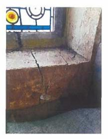
Photo 4 – Cracking to cill of East Chapel south window (internal)
