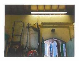
Photo 6 – Cracking to west wall of East Chapel (internal)
