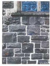
Photo 5 – Cracking below cill of East Chapel south window (external)
