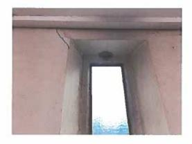
Photo 8 - Structural cracking around the east elevation north window (internal)
