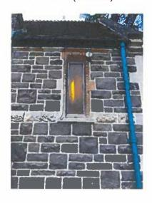
Photo 7 - Structural cracking around the east elevation north window (external)
