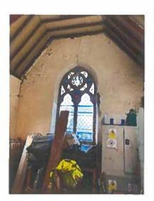
Photo 3 - Structural cracking and damp ingress to south wall of East Chapel (internal)
