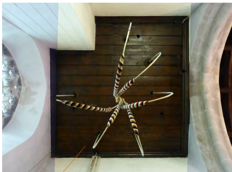
WEST TOWER CEILING VIEW
