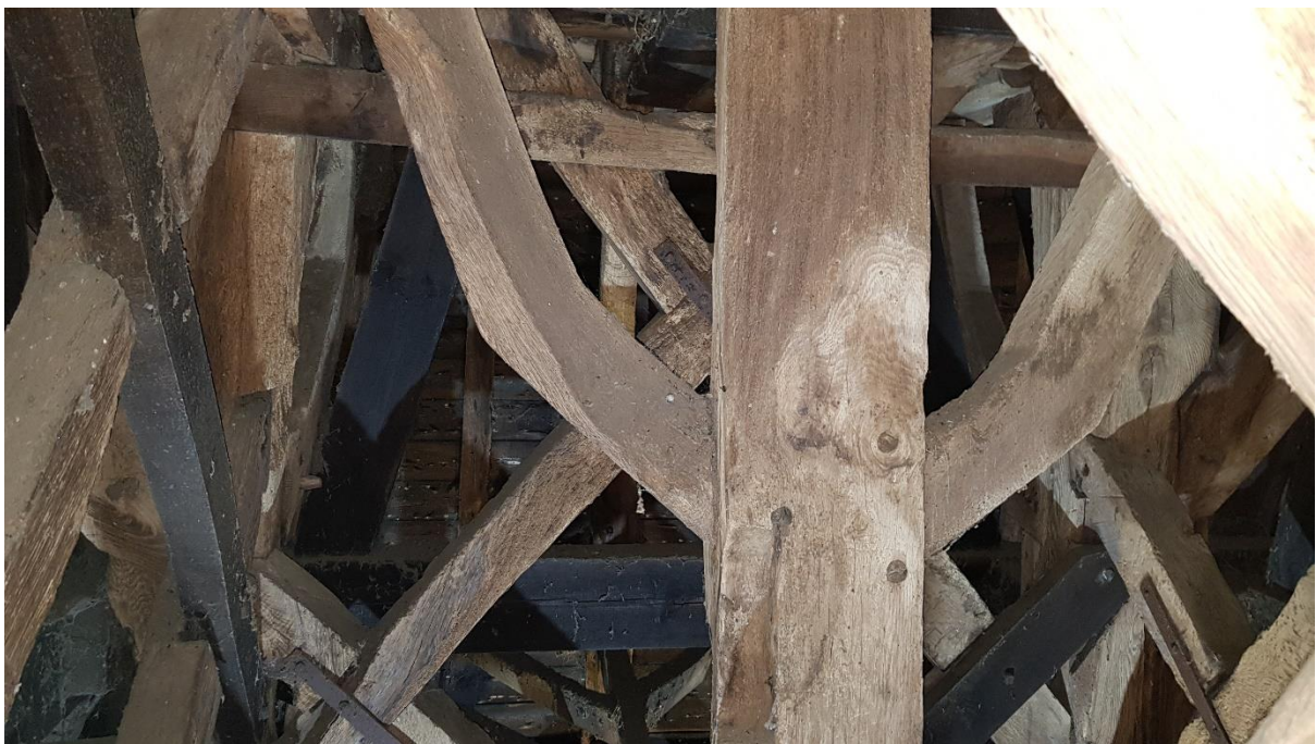
Interior framing (showing C13post structure with curved braces)
