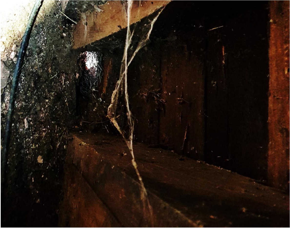
South side hole through wall-plate
