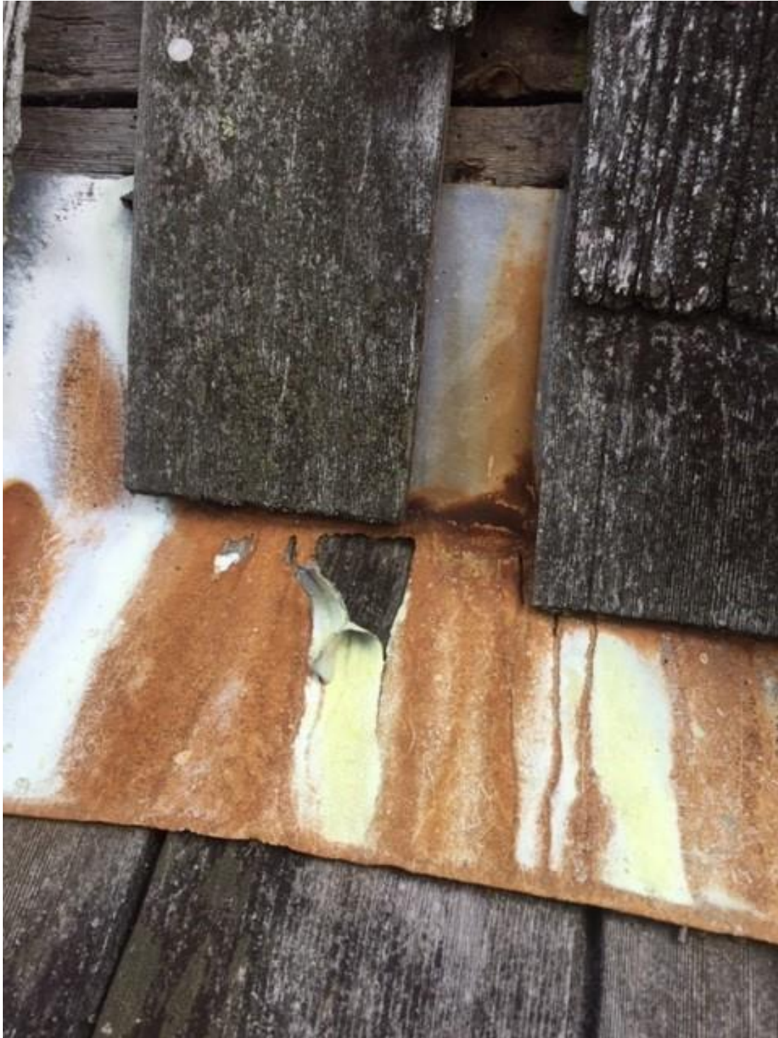
South side over sprocketed eaves, hole in lead (worn by acid run-off from shingles) and note condition of shingles with boarding below visible
