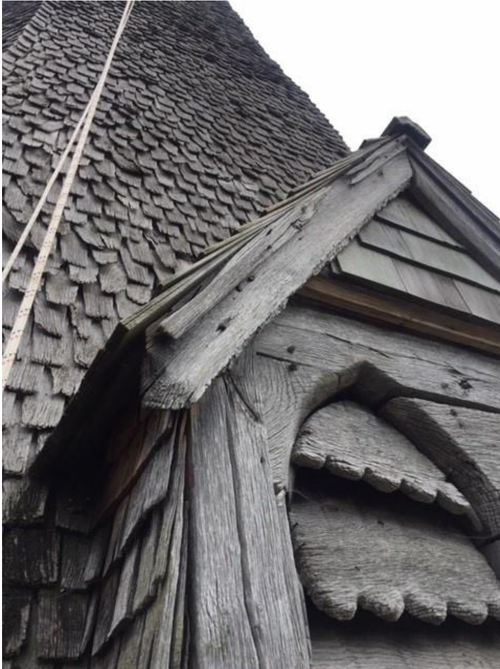
South lunette showing condition of barge and moulding and jamb
