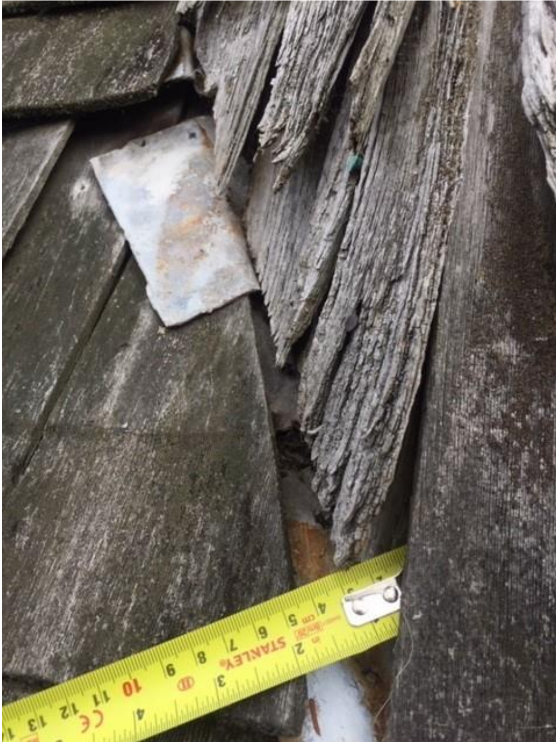
South valley very narrow flashings and note condition of shingles
