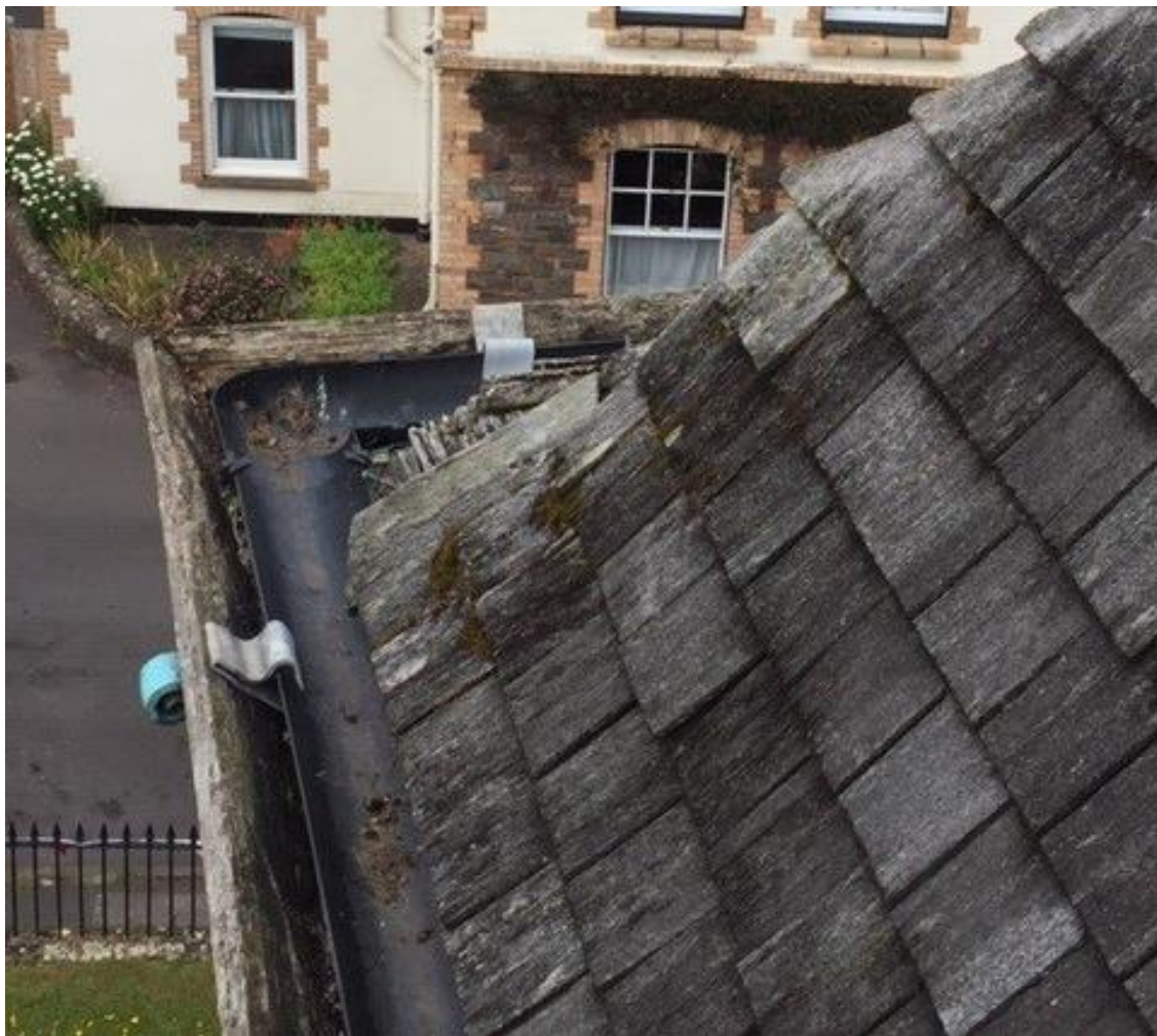
Southwest corner, missing shingles and rotten boarding
