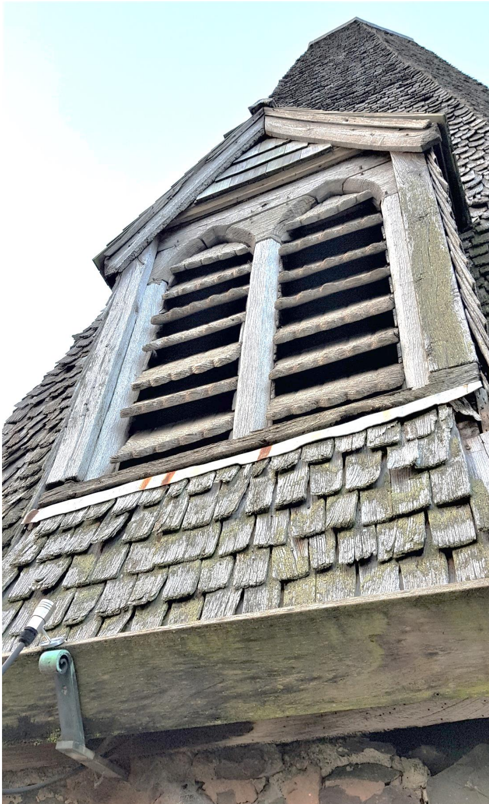
Lunette and gutter, west side note missing and curled shingles and rot in bottom of gutter
