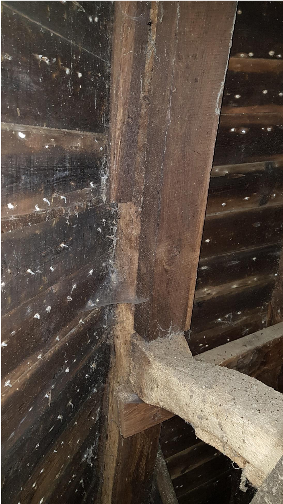
Joint between southwest hip and support member – multiple additional timbers and continued rot to hip
