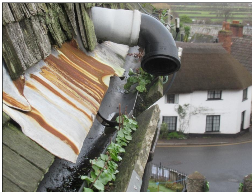
Inadequate guttering and spire roof rainwater collection requiring repair and renewal.
