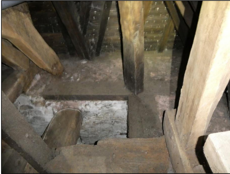
Typical wall plate arrangement on head of tower wall.
