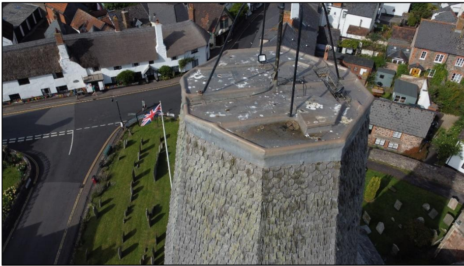
Octagonal lead flat roof to truncated spire.
