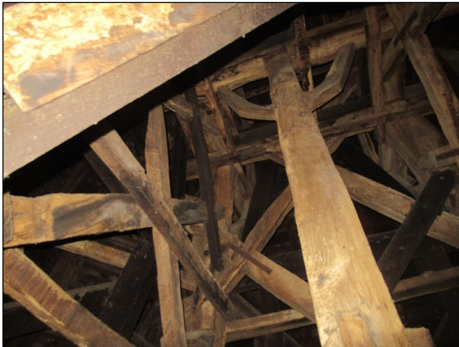
Central crown post showing original wing braces.
