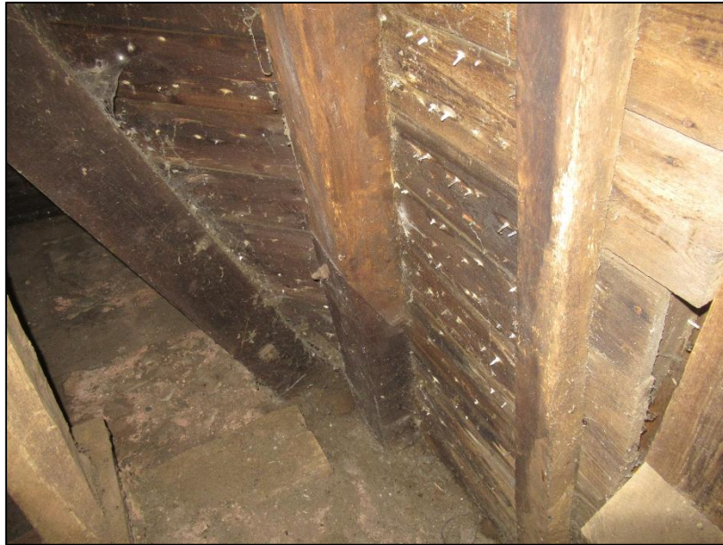
An example of a previous hip 'scarfed foot' repair undertaken in 1933.
