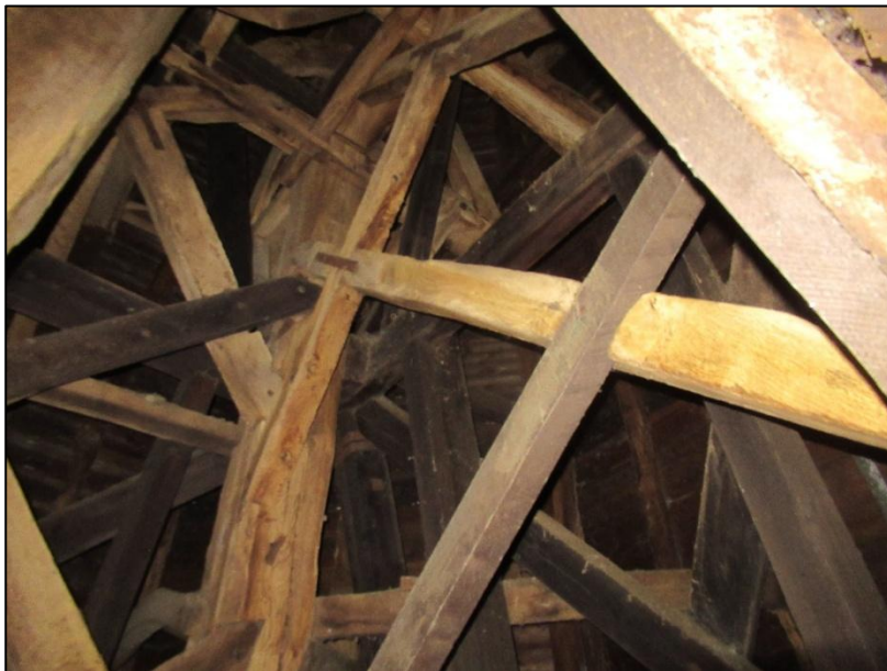
Strengthening timbers added in the late C19 and early C20.
