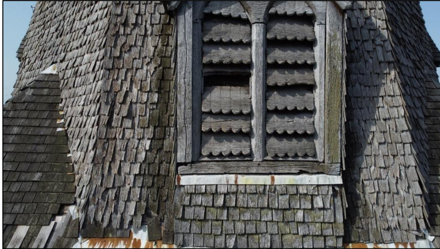
An example of deterioration of timber work around the southern lucarne.
