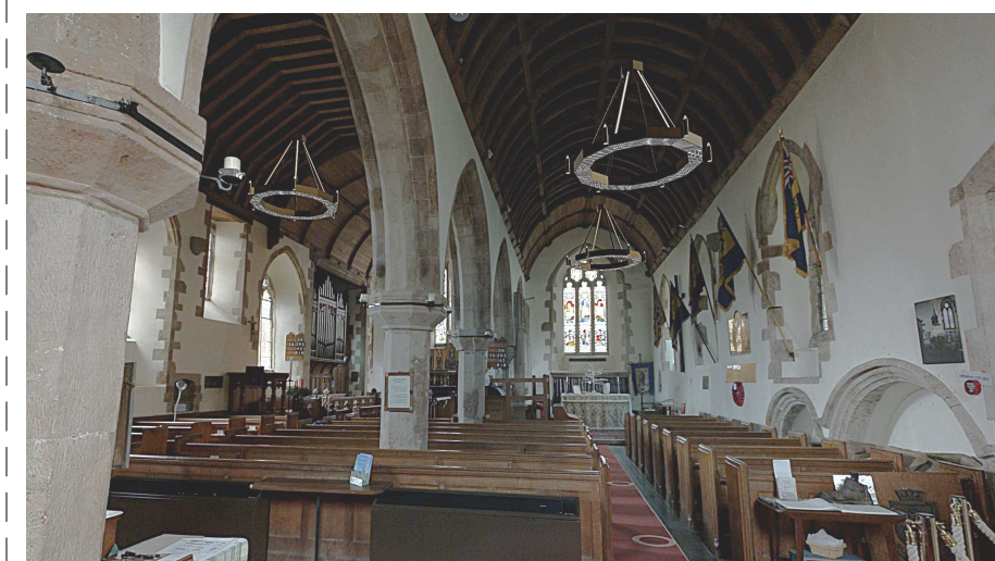
HERSCHEL HALO INFRARED HEATERS. FINAL POSITION TBC
