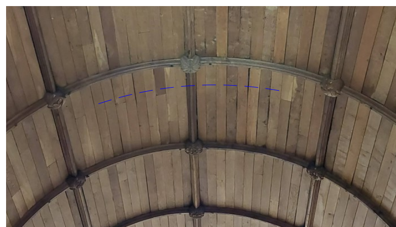
CHANCEL ROOF - (Strap to be fixed through board to truss behind)
