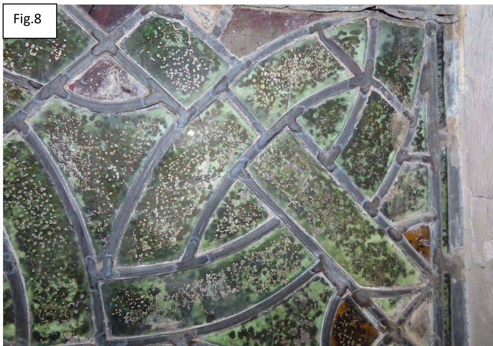
Corrosion pitting on the inside, showing white corrosion products
