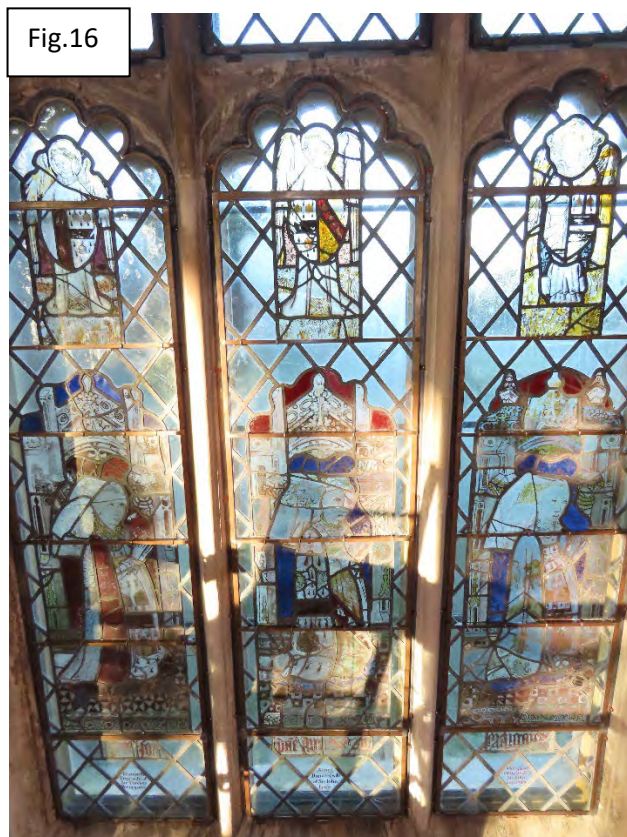
Examples of (from left to right) laminate glass; mouthblown glass in combination with wire grilles; mouthblown glass in simplified lead pattern
