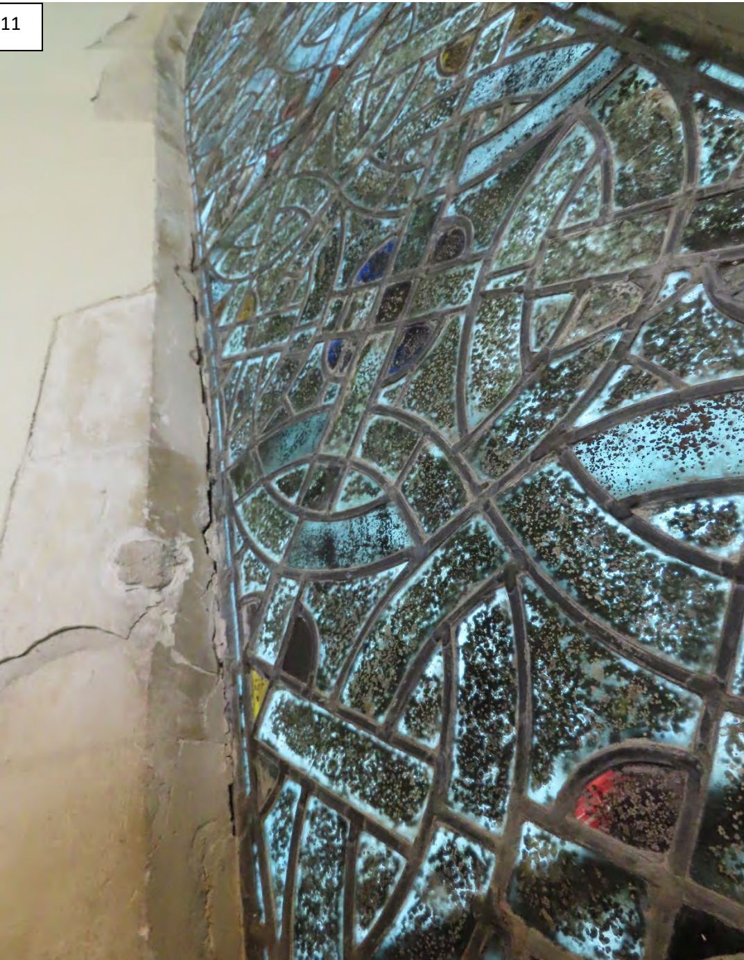
Damage to stonework through rust expansion of embedded ferramenta bar ends
