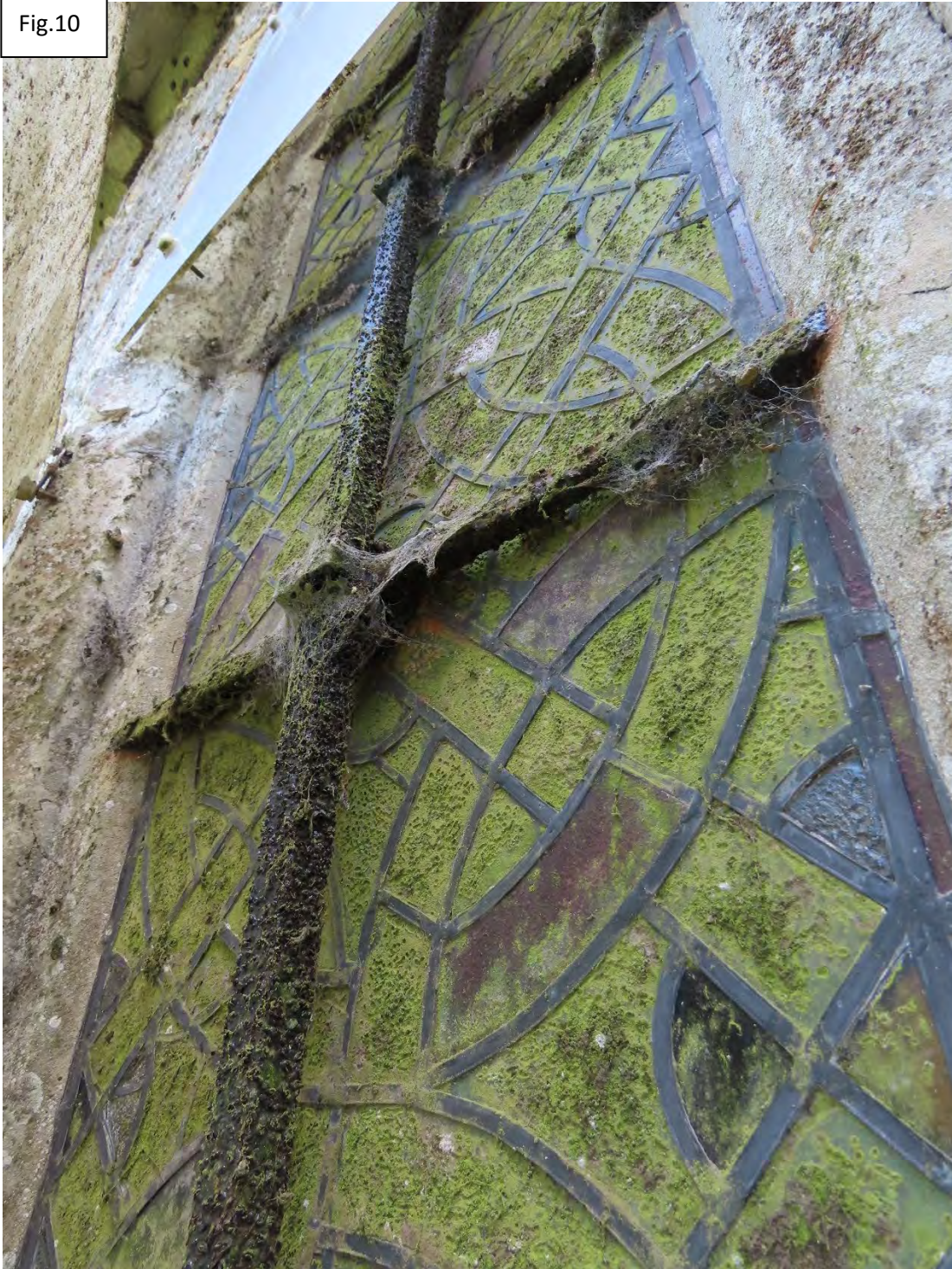
Microbial growths, dirt, cobwebs in interspace, rust staining of mortar at bar ends
