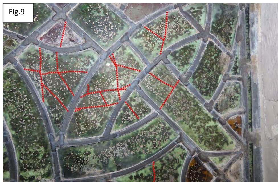
Glass fractures highlighted
