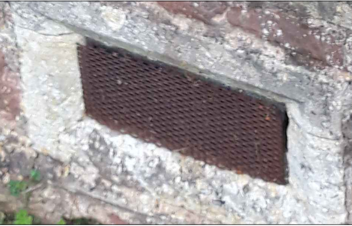
Cast Iron Grille. Above: Proposed, vent to provide 6500sqmm min vent area. Below: Existing on site south aisle elevation, with metal gauze.
