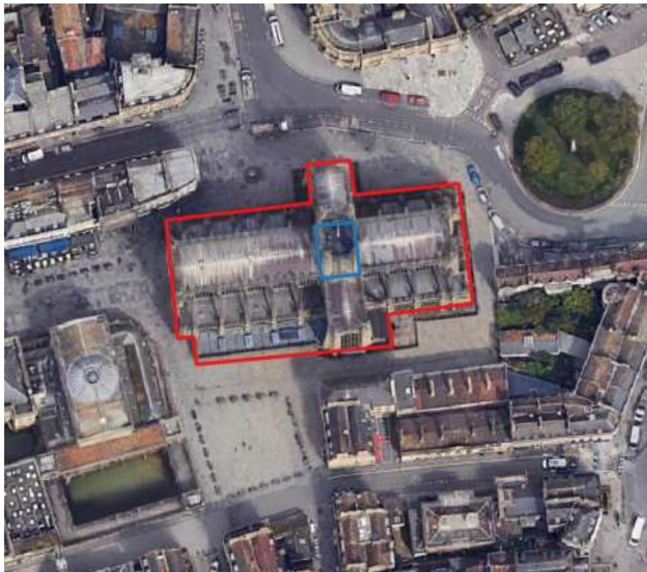
Image 1: Building subject to survey
