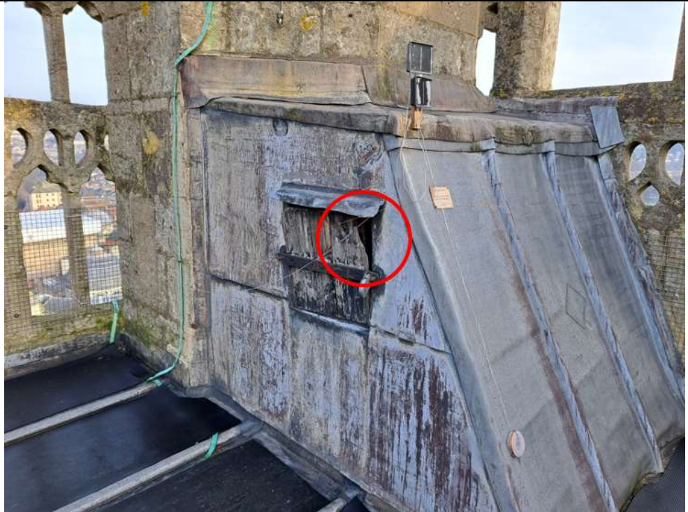
Access gap at side of timber hatch (leads to belfry)
