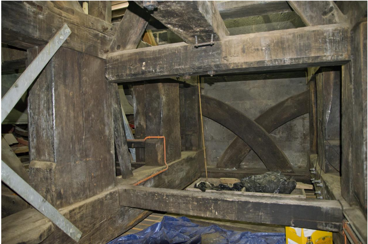
Plate 7 – Detail of the bell frame, showing curved braces
