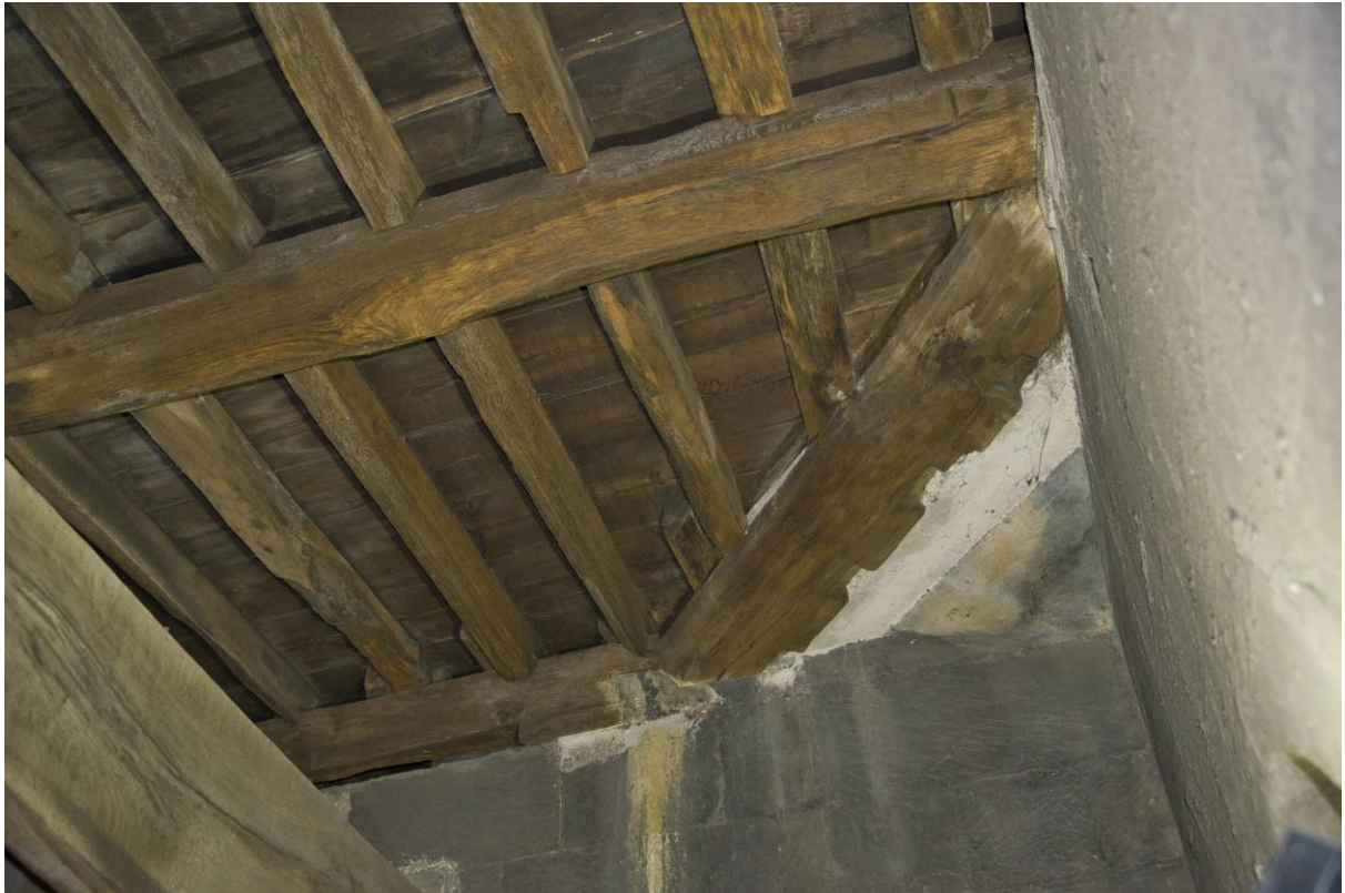
Plate 23 – South-east corner of the roof, dragon tie, looking east
