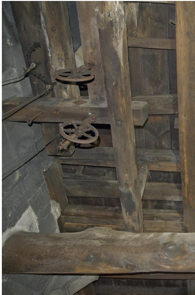
Plate 21 – North-east corner of the roof, 19 th century clock structure. View looking south
