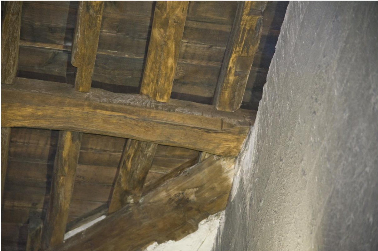
Plate 17 – Detail of original axial beam, showing chamfer stop
