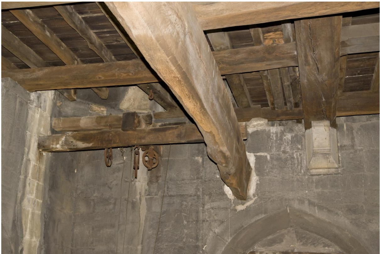
Plate 20 – North-east corner of the roof, showing lower cross-beam and 19 th century clock structure. View looking east
