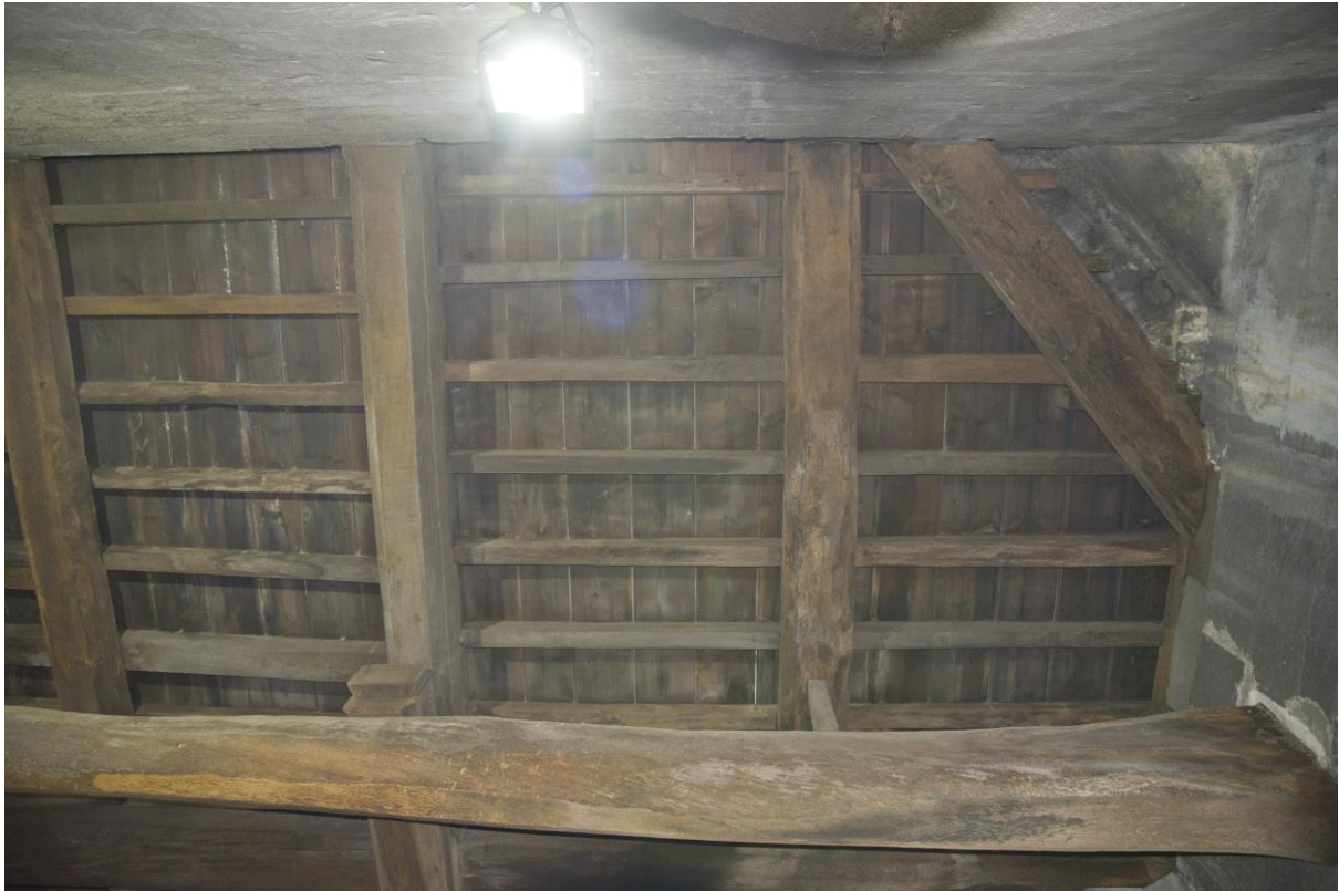
Plate 19 – Axial beams, joists and dragon ties, looking up
