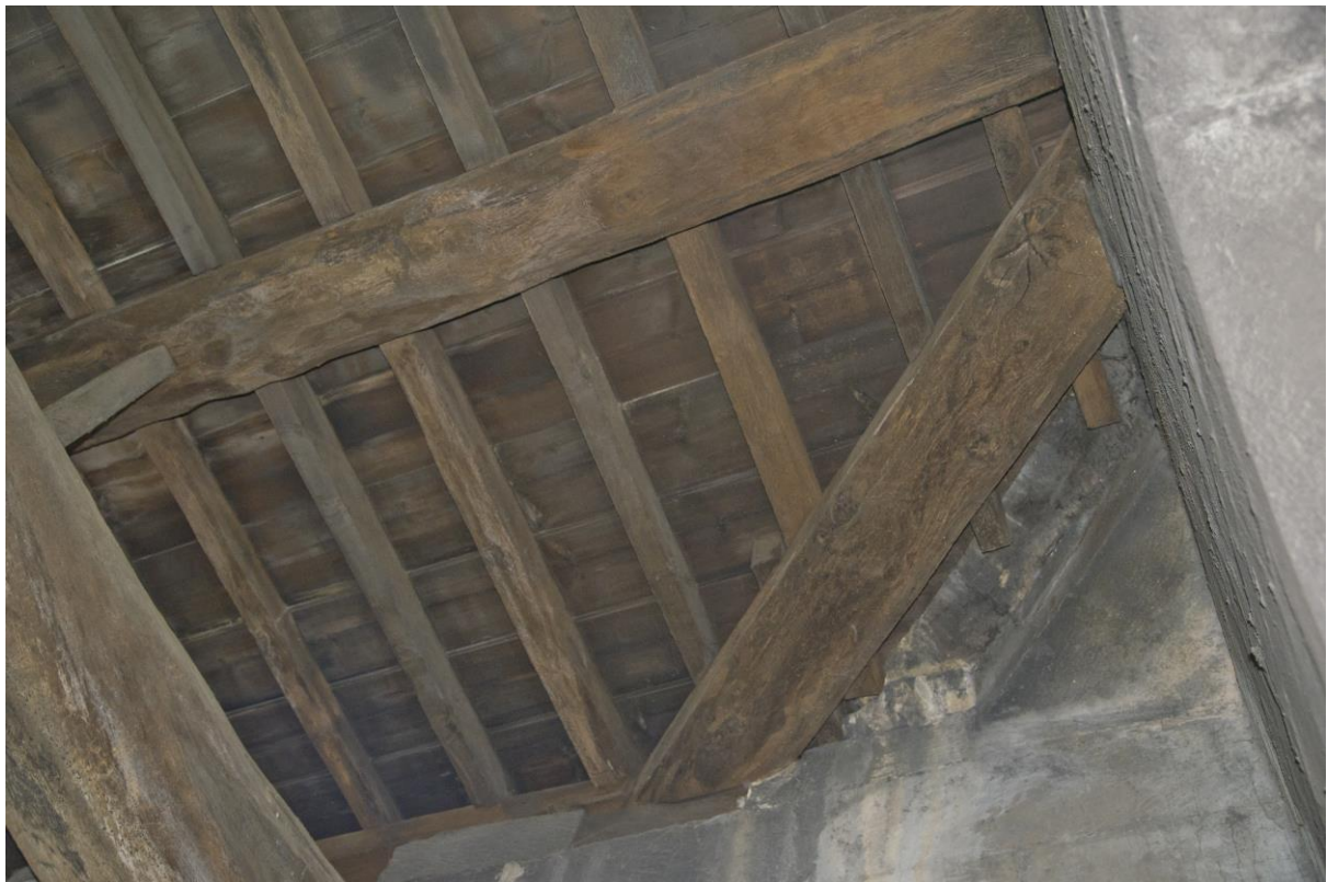
Plate 22 – North-west corner of the roof, dragon tie, looking south-west
