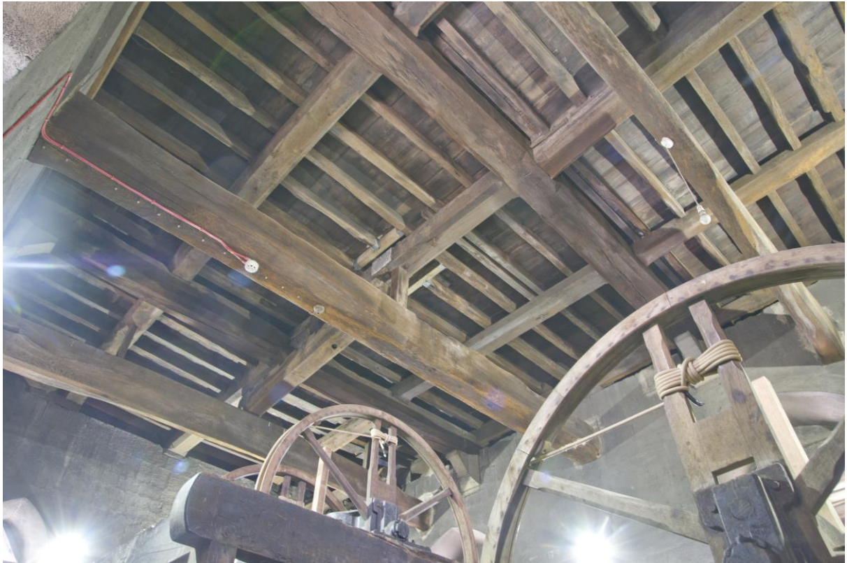
Plate 9 – General view of the roof structure, looking north-east
