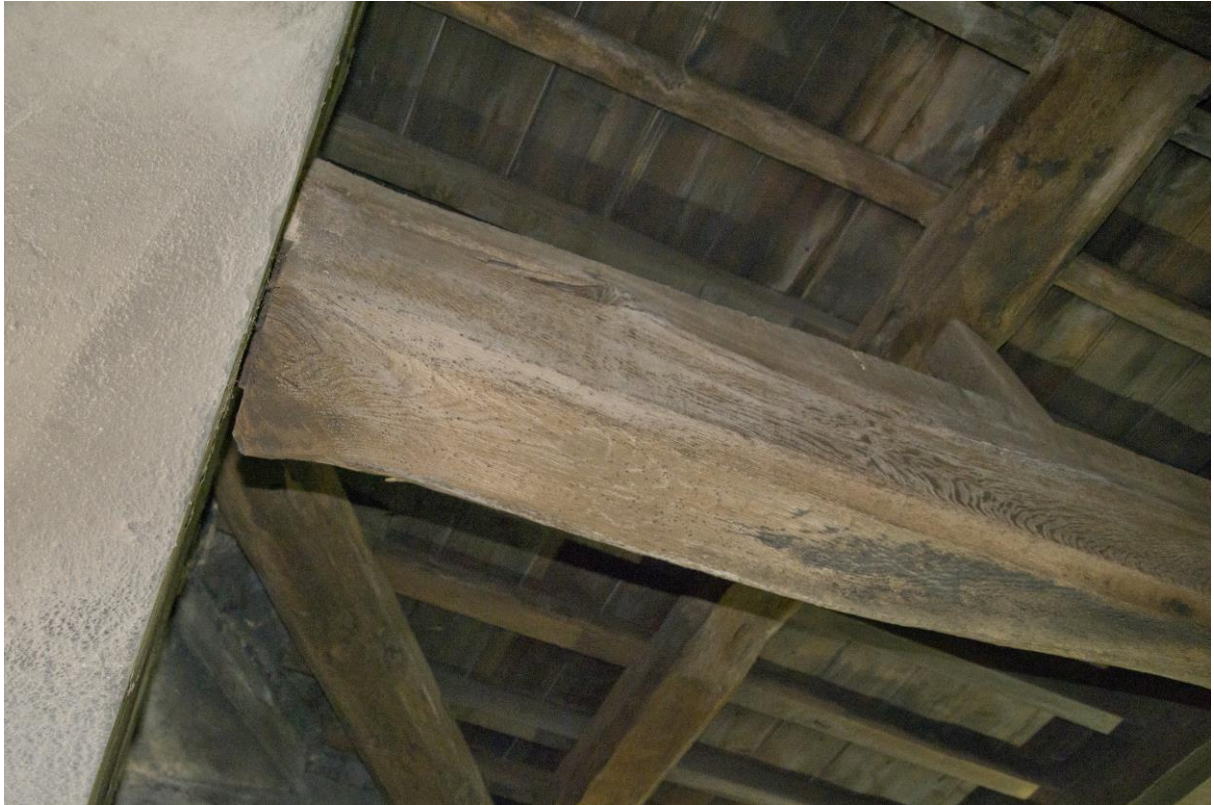
Plate 27 – Lower cross-beam, detail of chamfer stop
