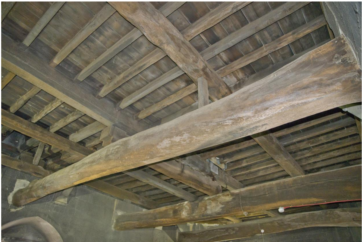
Plate 26 – Lower cross-beams, view looking south-east
