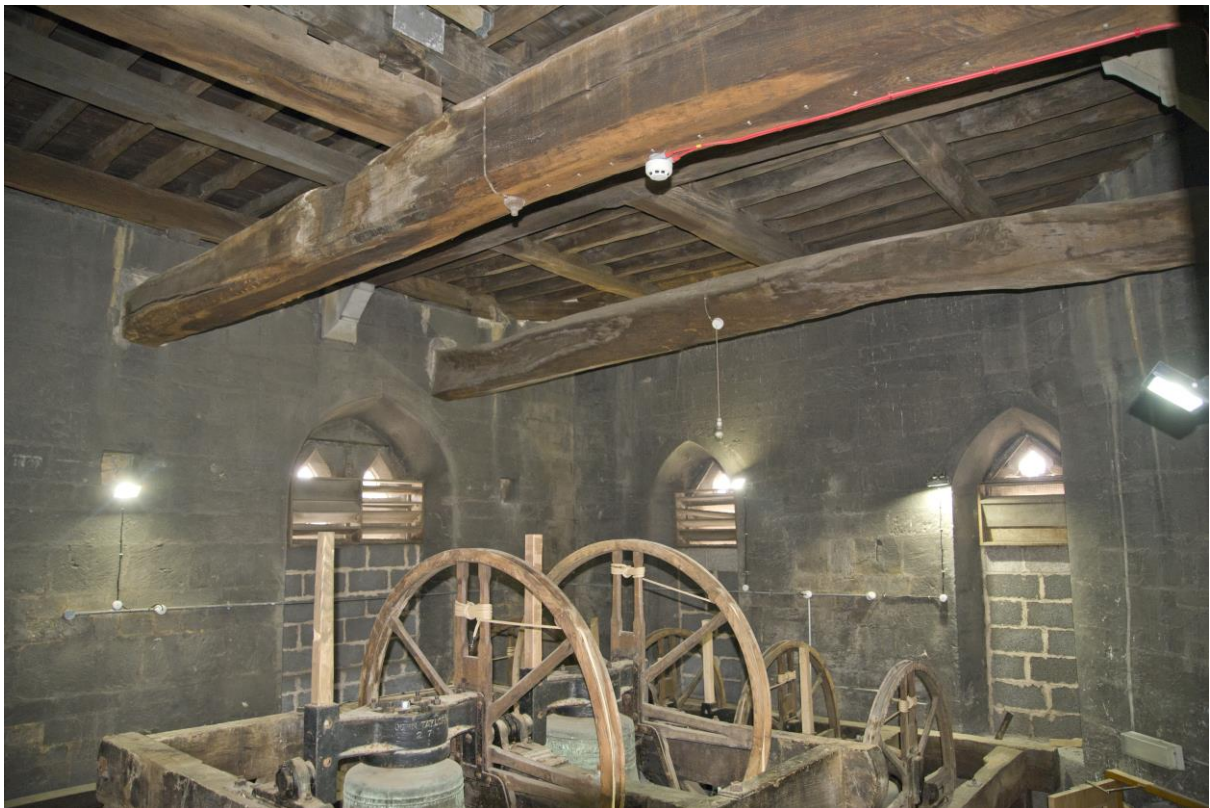
Plate 6 – General view of the belfry, looking south-east
