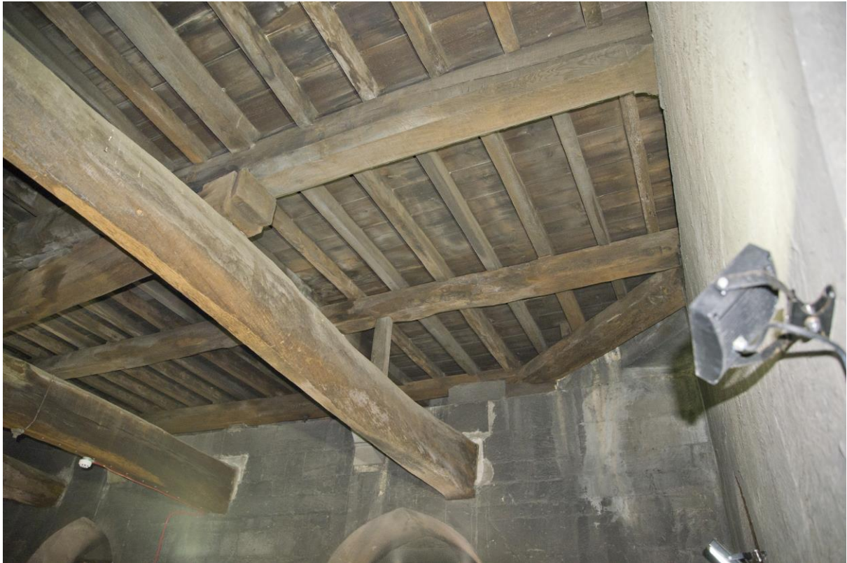
Plate 15 – Axial beams, joists and dragon ties, looking west
