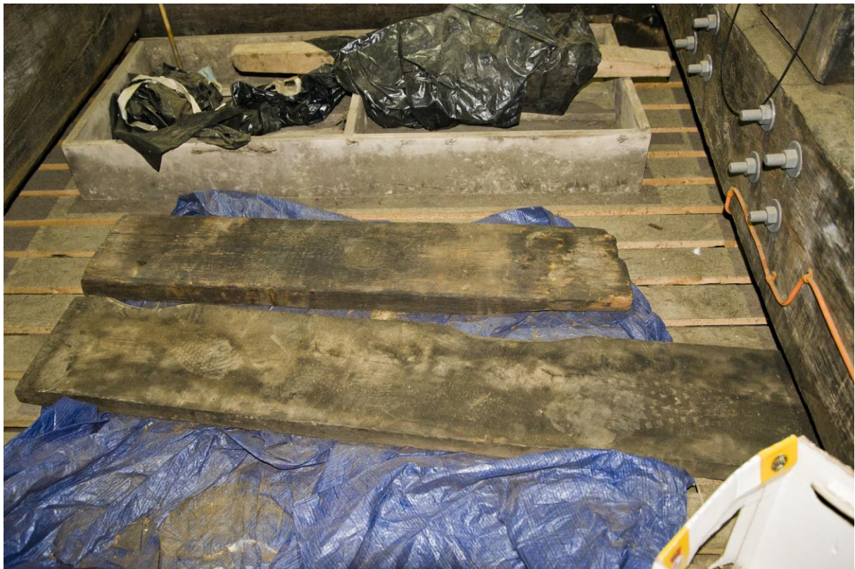
Plate 24 – Suspected historic sarking board retained within belfry level.
