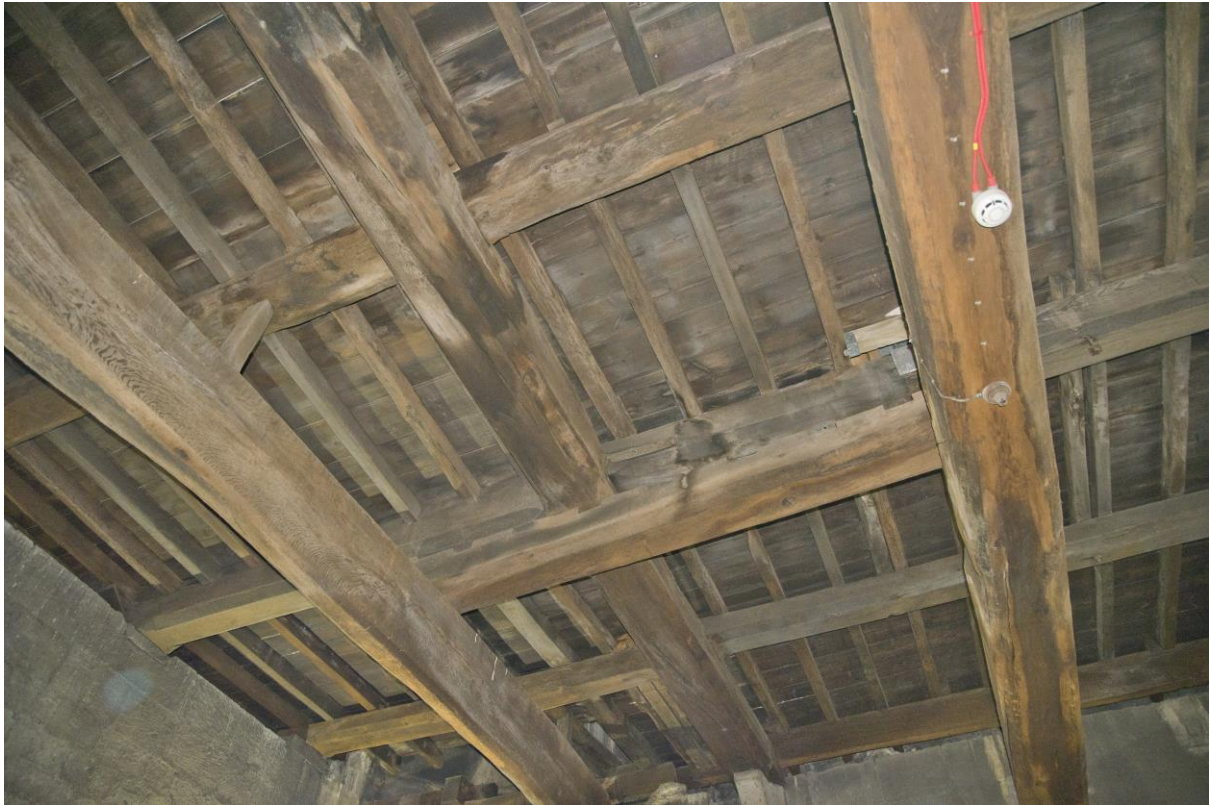
Plate 13 – General view of the roof structure, looking east
