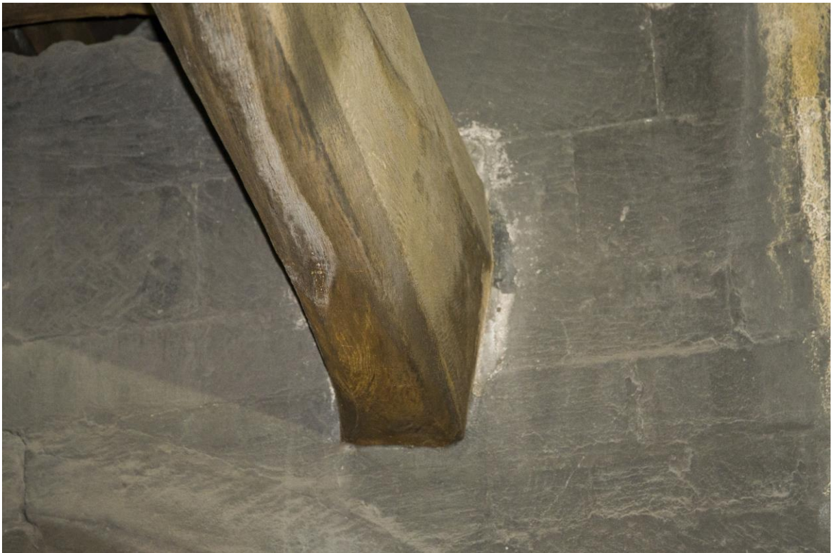
Plate 28 – Lower cross-beam, detail of chamfer stop
