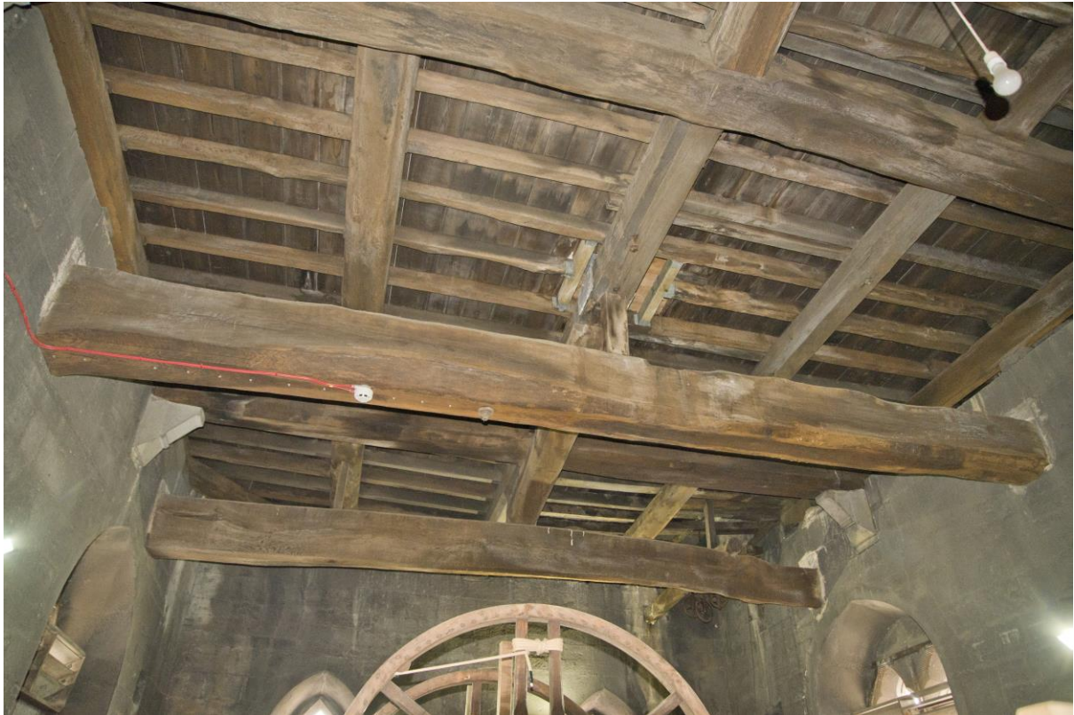
Plate 25 – Lower cross-beams, view looking north
