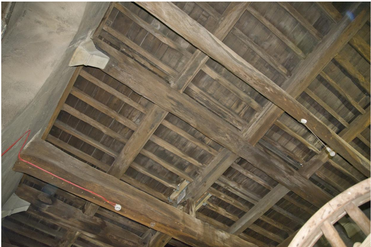
Plate 12 – General view of the roof structure, looking north-east
