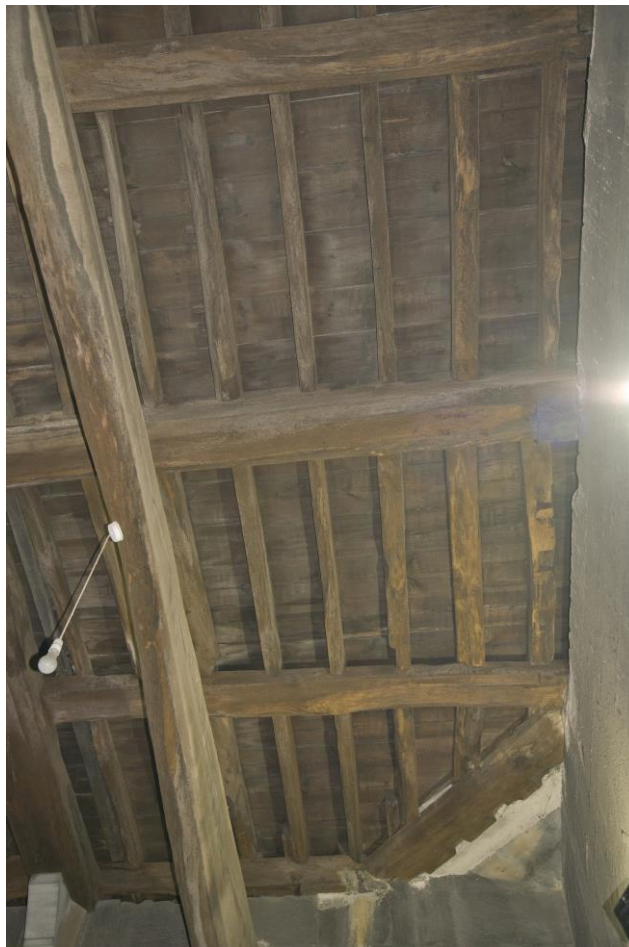
Plate 18 – Axial beams, joists and dragon ties, looking east
