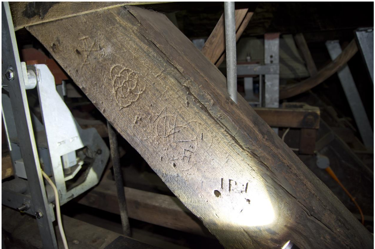
Plate 8 – Detail of the bell frame, showing apotropaic markings
