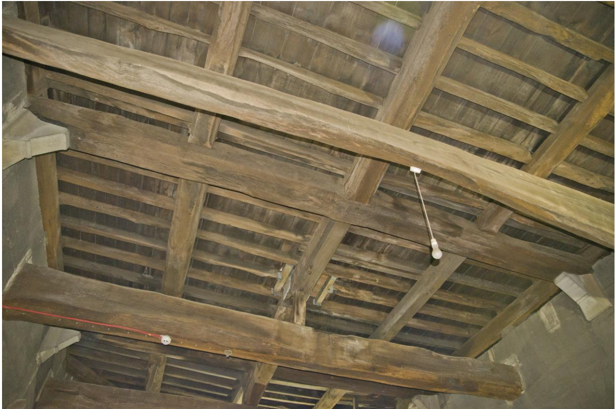
Plate 11 – General view of the roof structure, looking north
