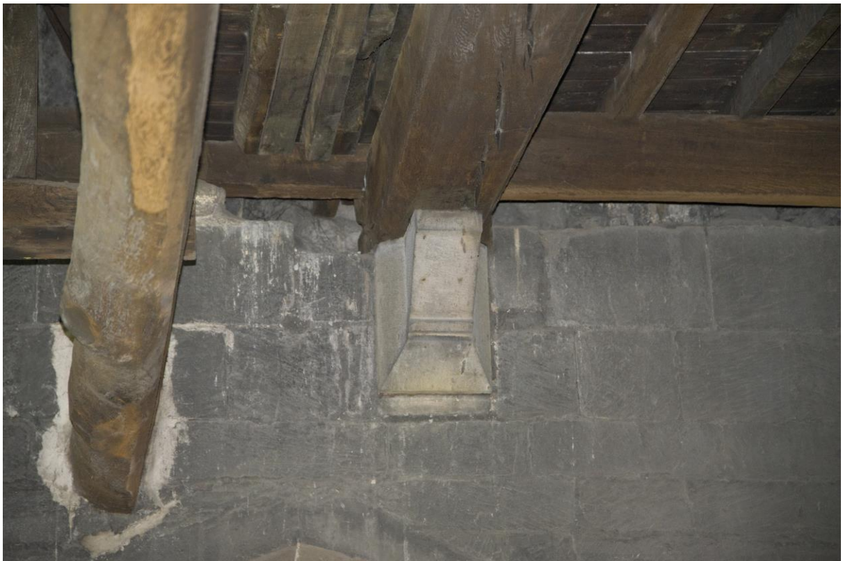
Plate 10 – Detail of an upper cross-beam corbel, looking east
