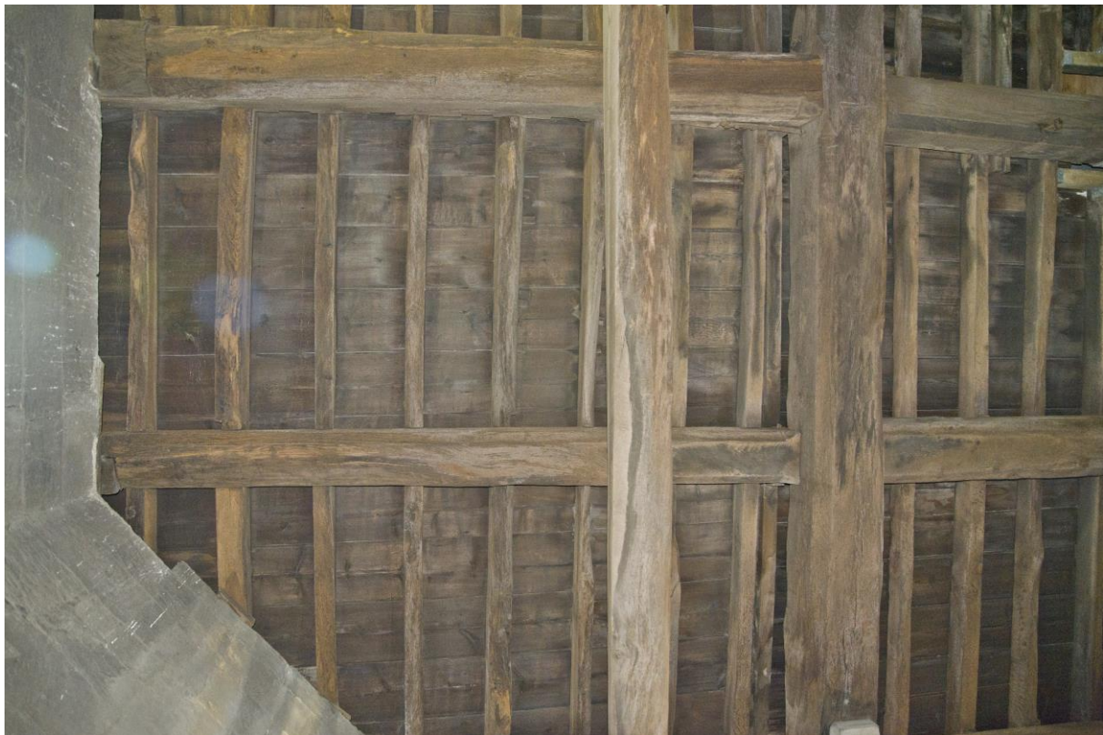
Plate 16 – Axial beams and joists, looking up
