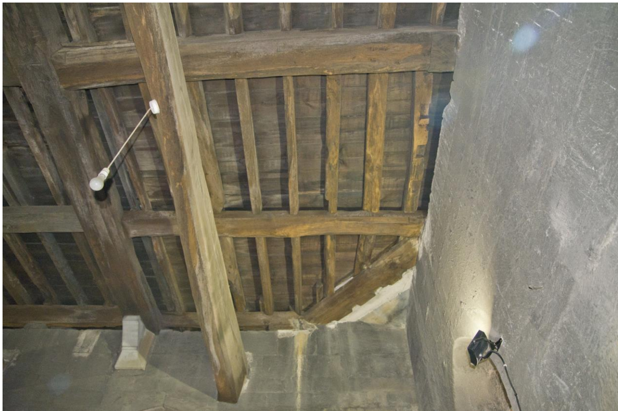
Plate 14 – Axial beams, joists and dragon ties, looking east
