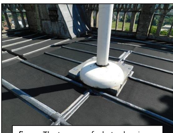
fig.02: The tower roof, photo showing flagpole connection and rubber matting laid over lead roof covering
