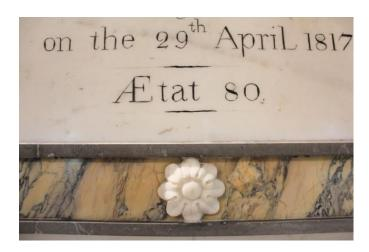
The ochre coloured, marble inlays have suffered dramatic *chromatic alteration* or loss of original surface polish. These areas were re-polished as far as possible using an abrasive softer than the host stone and treated with 2 layers of conservation-grade wax to protect them from poor ambient conditions within the building, due to sporadic heating.
