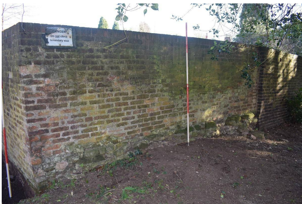
Plate D: Churchyard wall with rubble foundation, view: east
