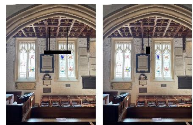
Australia chapel, looking south, with Aspect heater oriented either E-W ( left ) or N-S ( right ).
