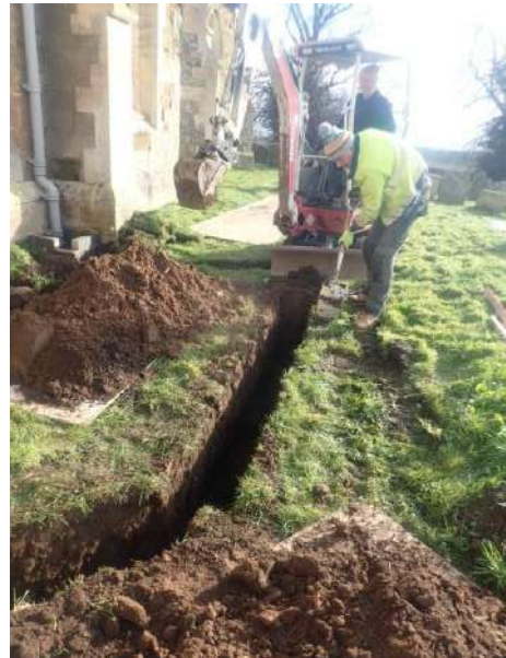
Plate 109: Excavation of main service trench, from the west
