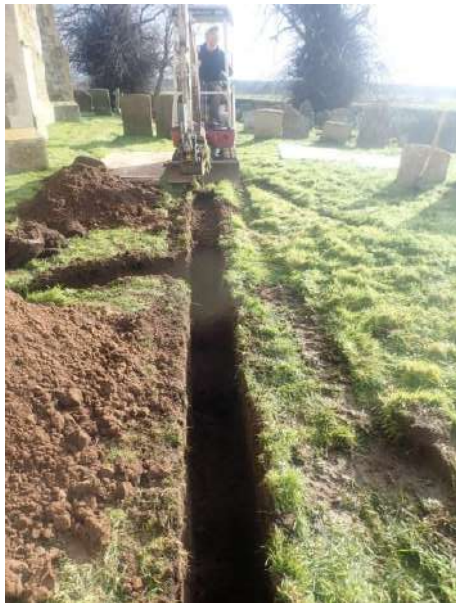
Plate 115: Excavation of main service trench, from the west
