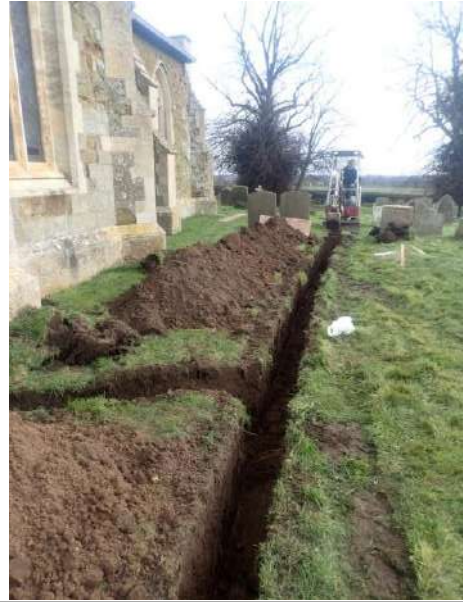
Plate 124: Excavation of main service trench, from the west
