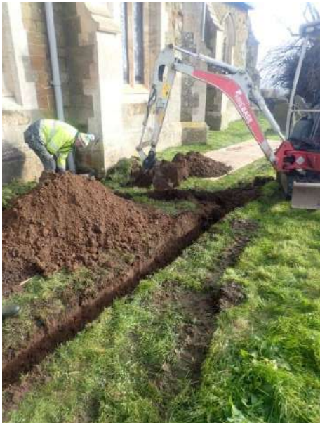
Plate 111: Excavation of main service trench, from the west
