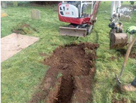
Plate 156: Excavation of the second soakaway, from the west
