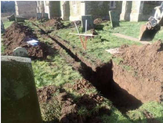
Plate 162: Excavation of the second soakaway, from the east
