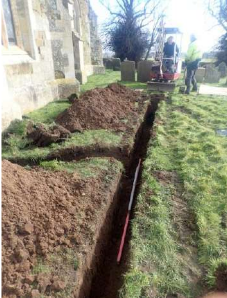
Plate 118: Excavation of main service trench, from the west
