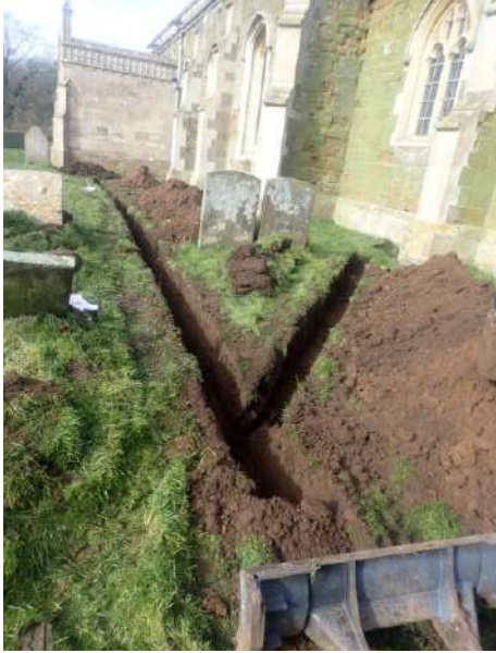
Plate 134: Excavation of main service trench and of the trench from the third gully, from the east
