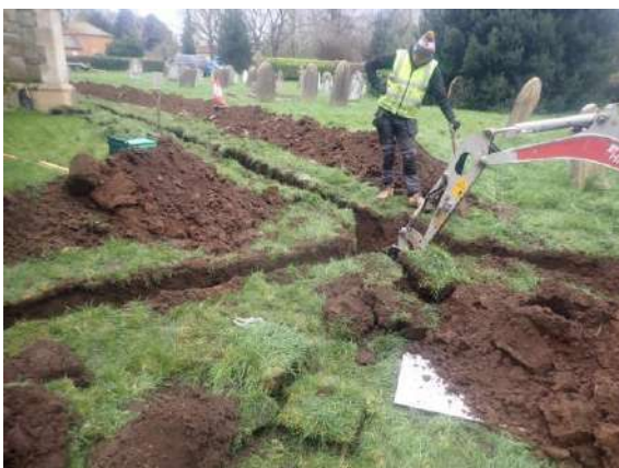
Plate 60: Excavation of the first catch water pit, from the south-east
