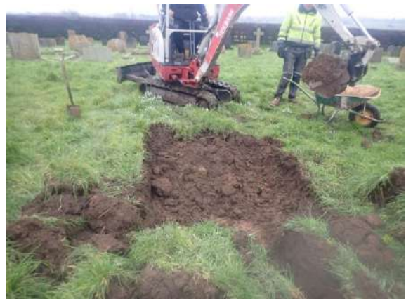
Plate 88: Excavation of the first soakaway, from the west
