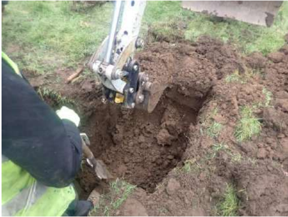
Plate 146: Excavation of the second catch water pit, from the west
