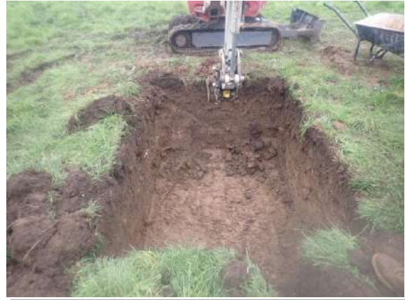
Plate 100: Excavation of the first soakaway, from the west
