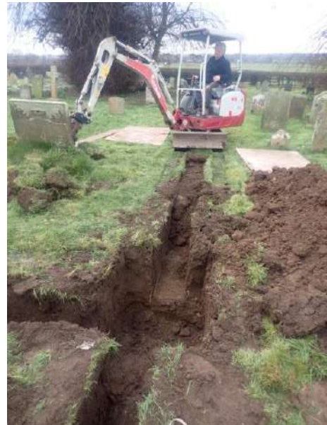
Plate 149: Excavation of the main service trench, from the west
