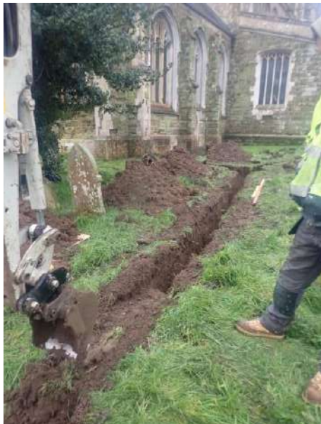
Plate 69: Excavation of the main service trench, from the east
