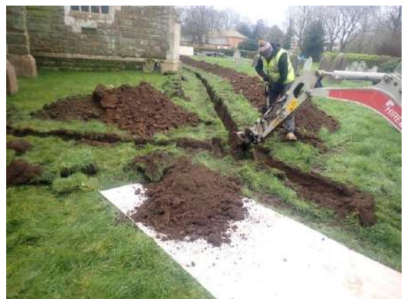
Plate 57: Excavation of the drainage trenches, from the east
