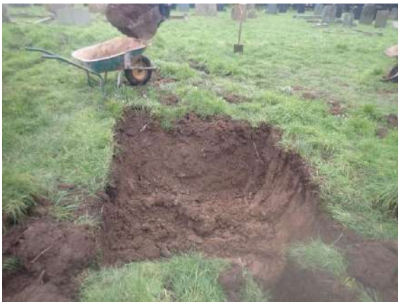
Plate 90: Excavation of the first soakaway, from the west
