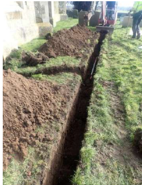
Plate 121: Excavation of main service trench, from the west
