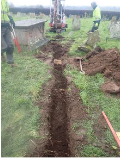
Plate 76: Excavation of the main service trench, from the west
