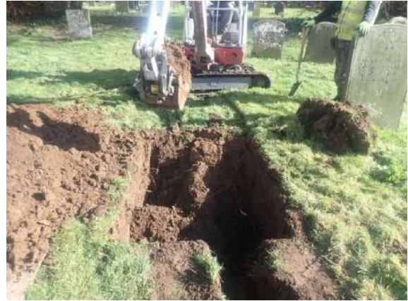
Plate 158: Excavation of the second soakaway, from the west
