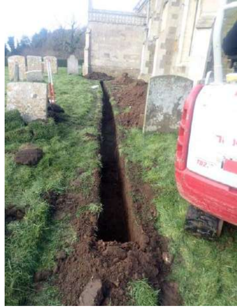
Plate 128: Excavation of main service trench, from the east
