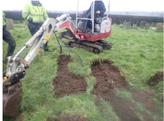
Plate 87: Excavation of the first soakaway, from the west
