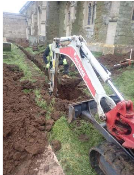
Plate 145: Excavation of the second catch water pit, from the east
