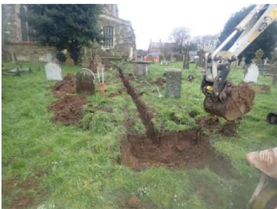
Plate 91: Excavation of the first soakaway, from the east
