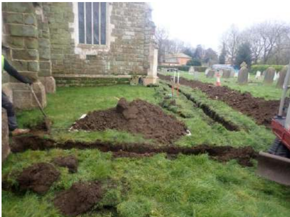
Plate 49: Excavation of the drainage trenches, from the east
