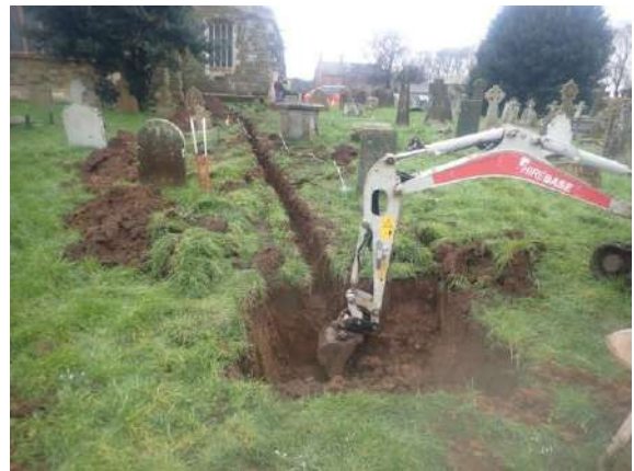
Plate 93: Excavation of the first soakaway, from the east
