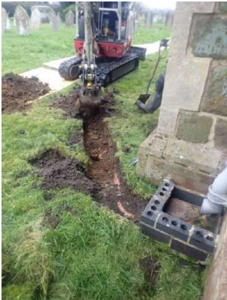
Plate 12: Excavation of the trench from the first gully, from the north-west
