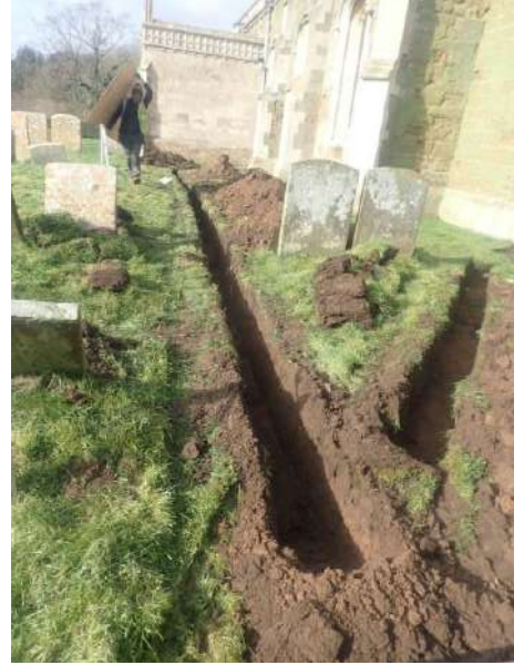
Plate 132: Excavation of main service trench and of the trench from the third gully, from the east
