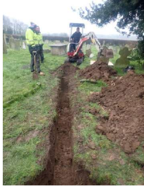
Plate 66: Excavation of the main service trench, from the west
