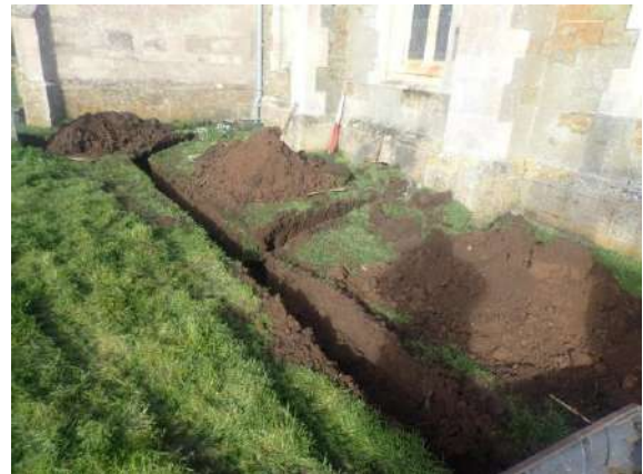
Plate 117: Excavation of main service trench, from the east
