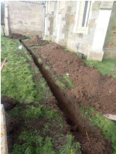
Plate 123: Excavation of main service trench, from the east
