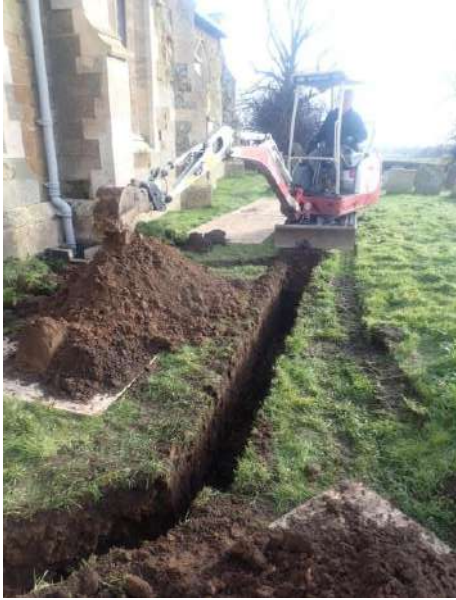
Plate 110: Excavation of main service trench, from the west
