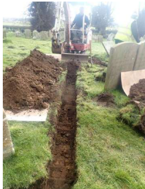
Plate 129: Excavation of main service trench, from the west
