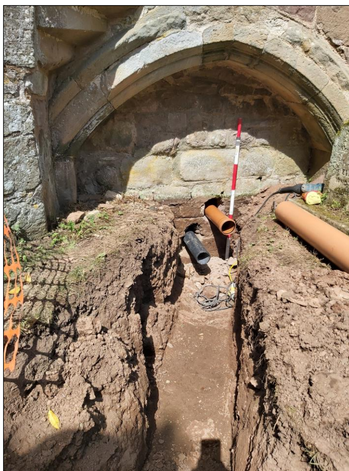
Plate 3: View looking NNE showing insertion of pipe through the wall to connect with internal WC.
