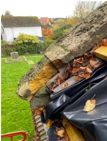
Photo 3 – Fractured kneeler stone to east end of north aisle
