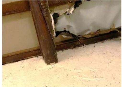
Photo 6 – Fracturing of roof purlin and damage to ceiling panel.
