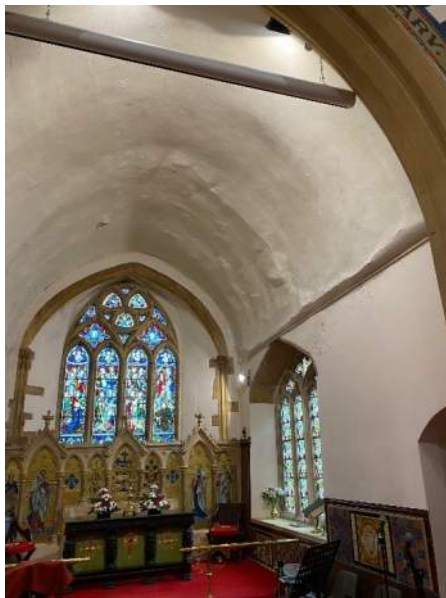
Photo 9 – Degraded plaster work to barrel-vaulted ceiling of Chancel.
