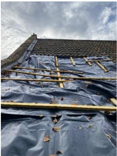
Photo 2 - Roof temporarily sheeted above east end of north aisle
