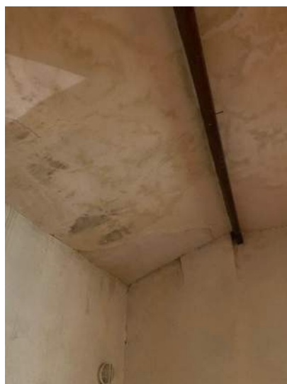
Photo 7 – Damaged ceiling structure over organ. Down stand purlin appear sound
