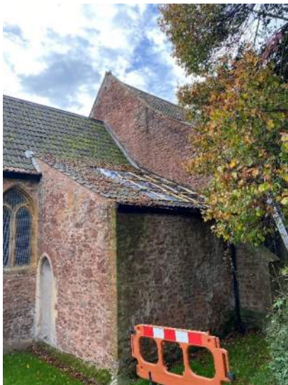
Photo 1 – Roof temporarily sheeted above organ room
