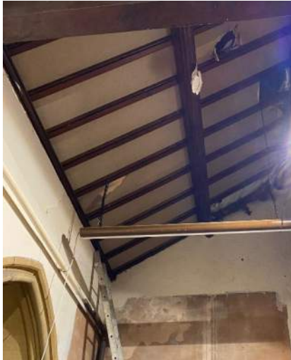
Photo 5 – Damage to ceiling panels of north aisle. Fracturing of masonry above east window.
