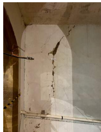
Photo 8 – Area of severe ceiling fracturing within the organ room. Fracturing to the north wall.
