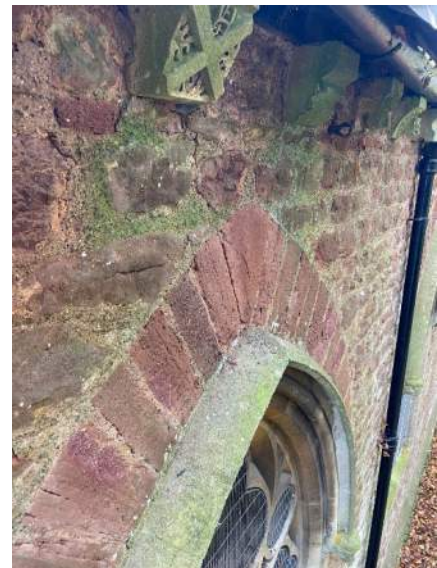
Photo 4 – Failing keystone and fracturing of masonry above (north aisle, east end)
