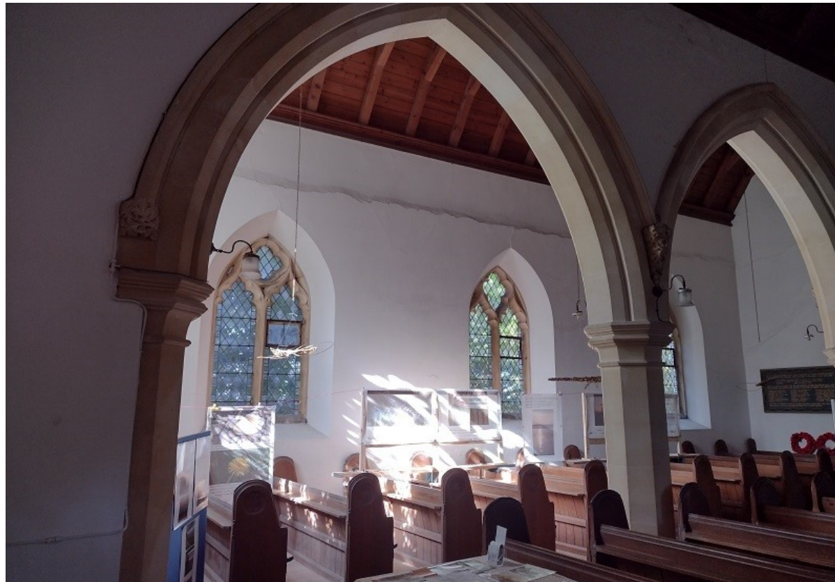
The north aisle, set to become our community area
