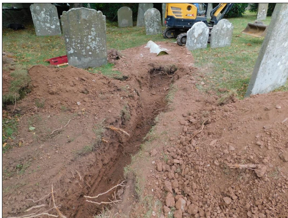
Plate 2: Trench connecting pit to the existing drain run: view NE
