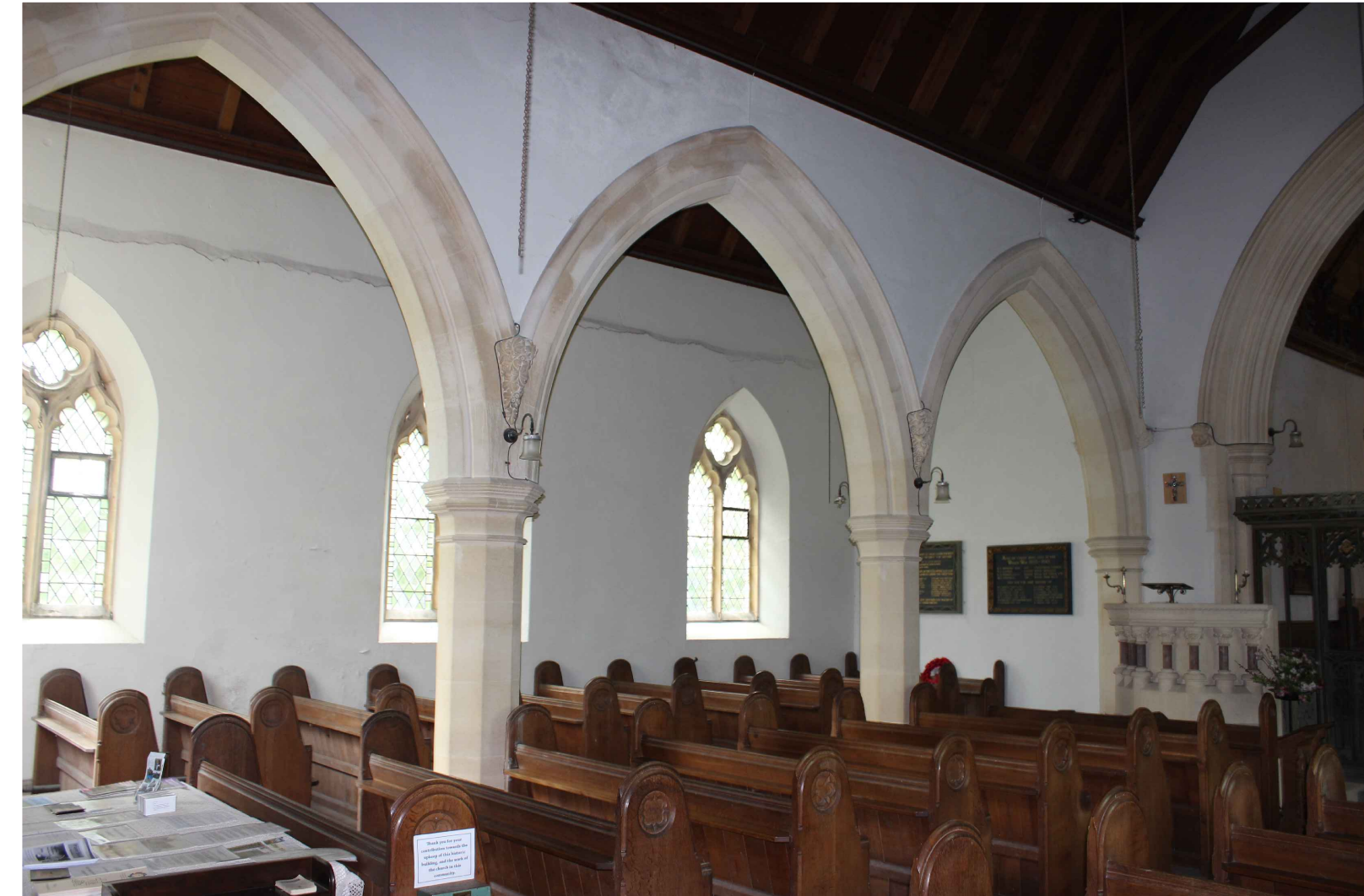
North Aisle from Nave looking North-East showing columns/arcade
