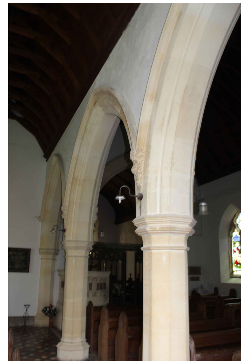
North Aisle looking East showing columns/arcade
