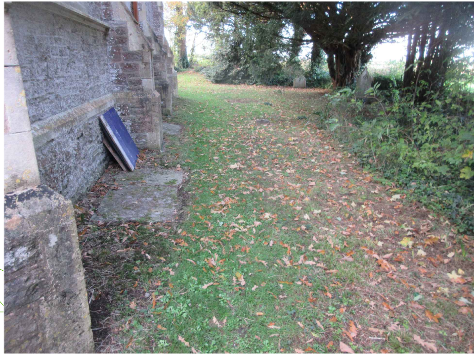
Location for Trench Arch System looking West
