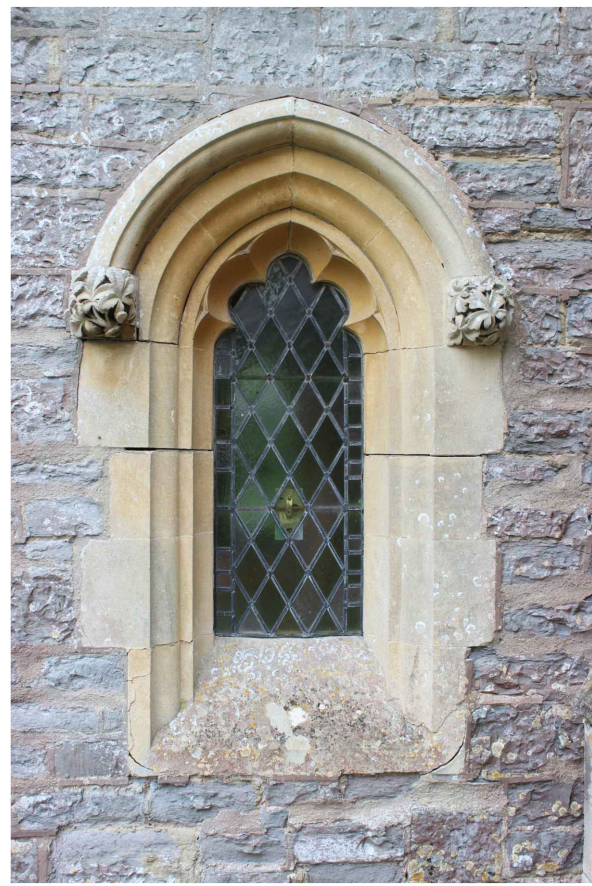
WINDOW SVI - SOUTH PORCH
