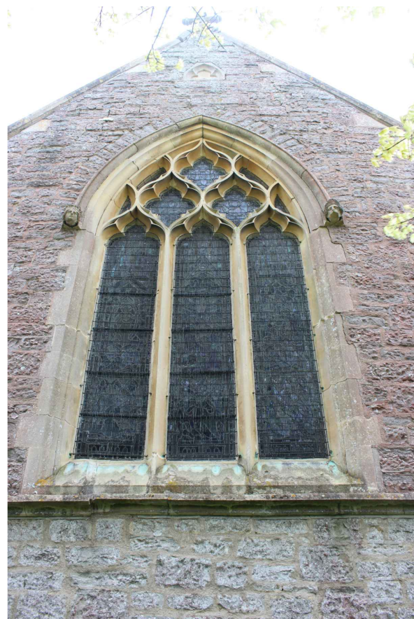
WINDOW EI (EAST WINDOW - CHANCEL)
