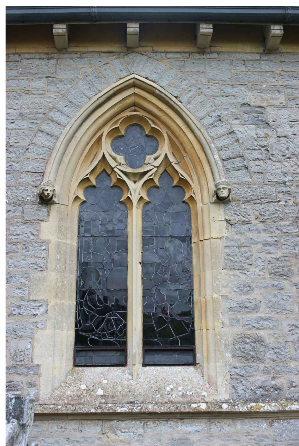
WINDOW SV (NAVE)
