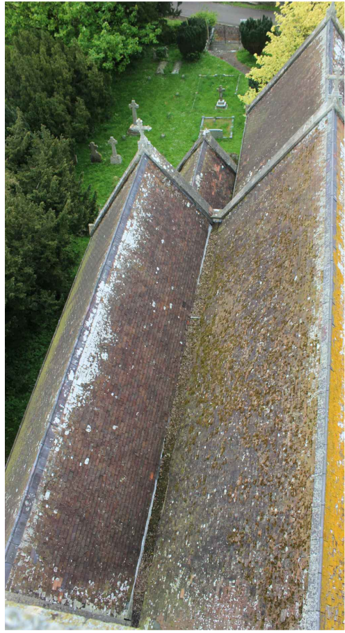
Photos of roofs from top of the tower
