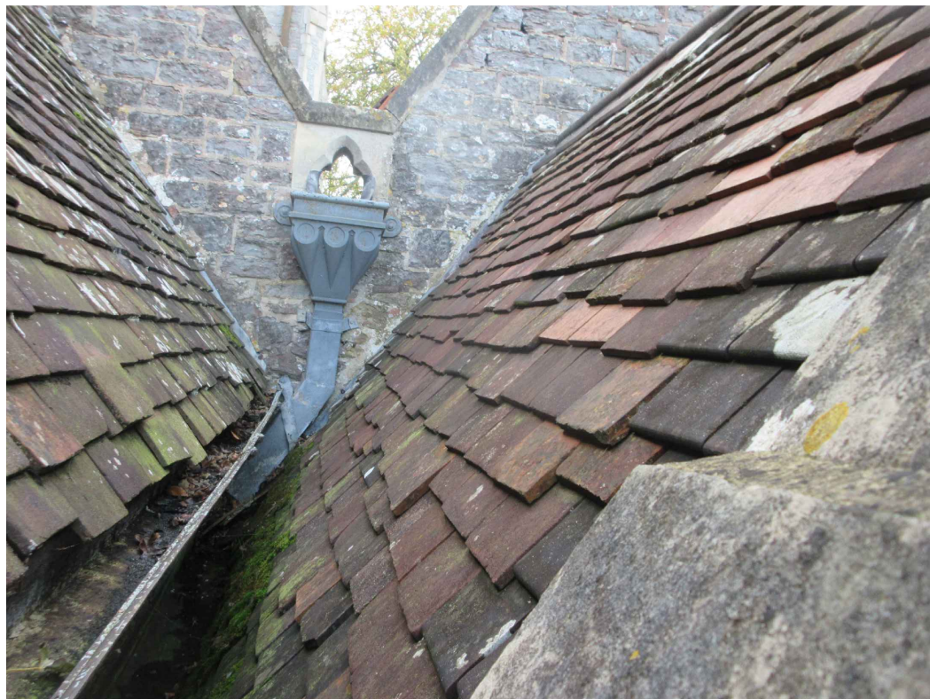
Photo of valley gutter above vestry
