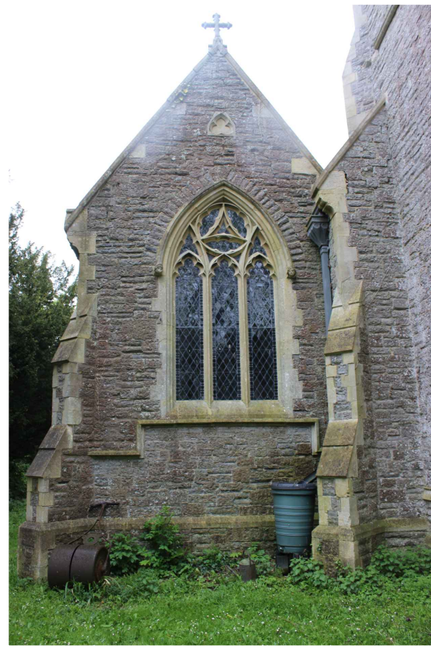
WEST END OF NORTH AISLE
