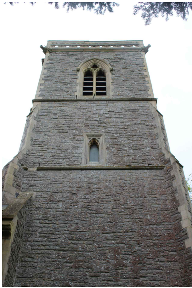
NORTH ELEVATION OF TOWER
