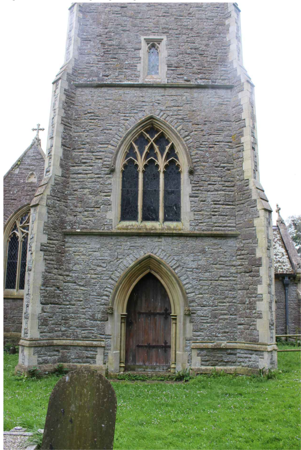
WEST ELEVATION OF TOWER
