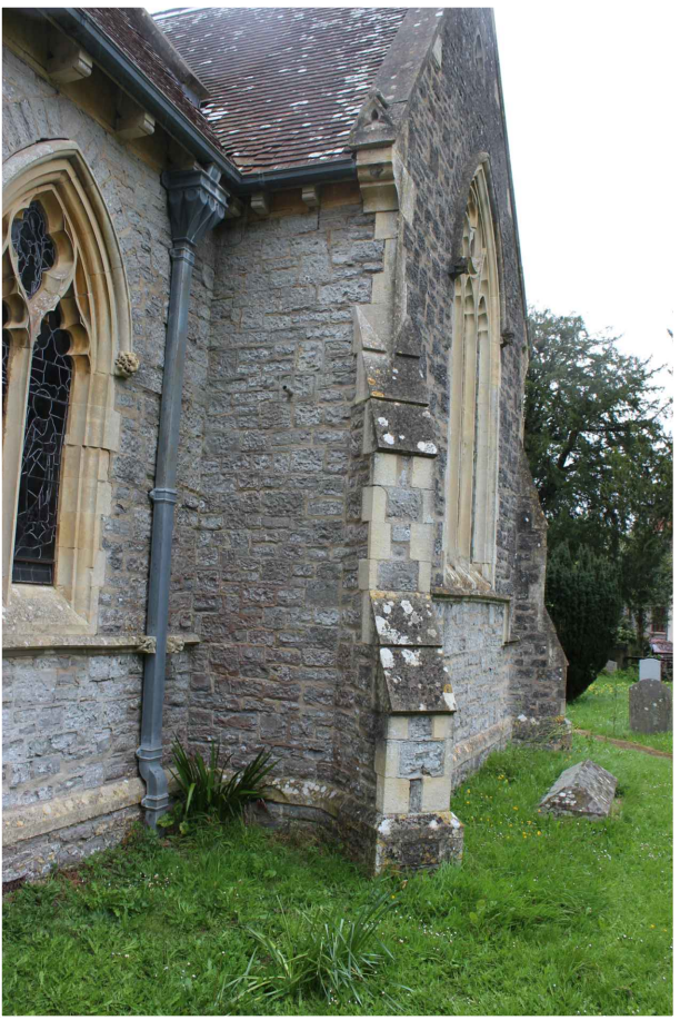
WEST SIDE OF SOUTH CHAPEL/ ORGAN CHAMBER
