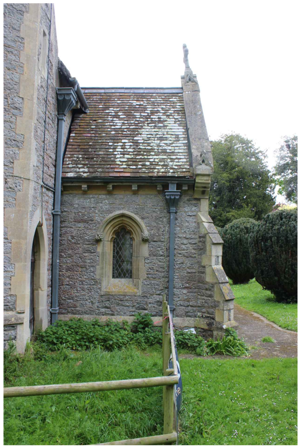
WEST SIDE OF SOUTH PORCH
