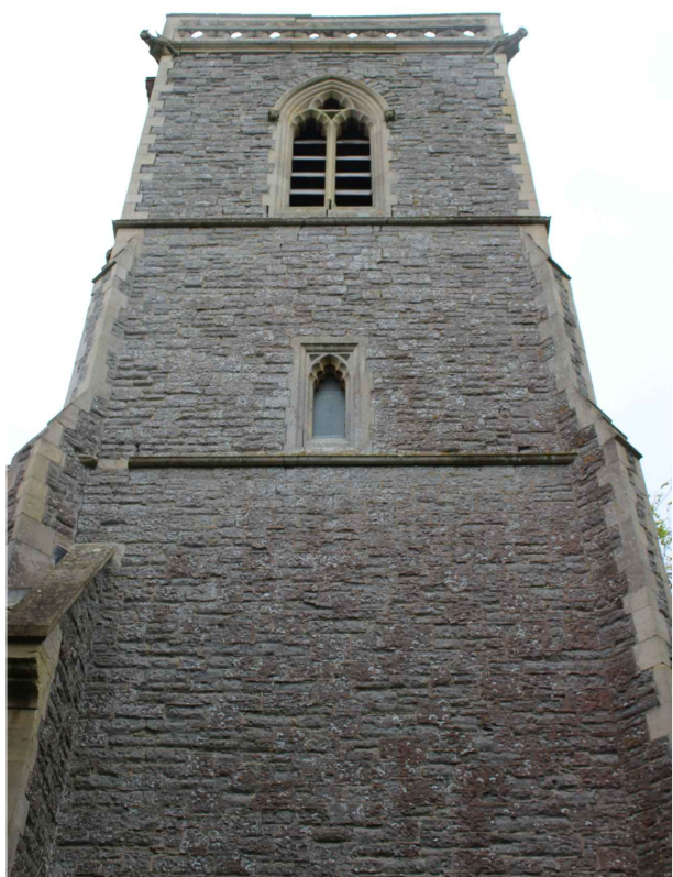
NORTH ELEVATION OF TOWER (UPPER STAGES)
