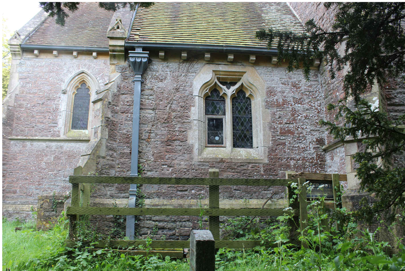
NORTH ELEVATION OF EXISTING VESTRY
