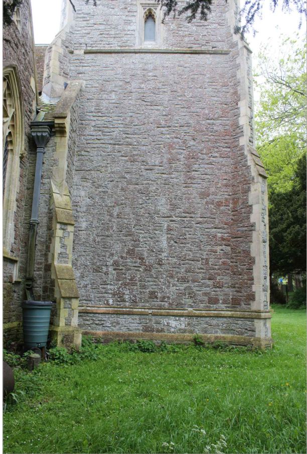
NORTH ELEVATION OF TOWER (LOWER STAGE)
