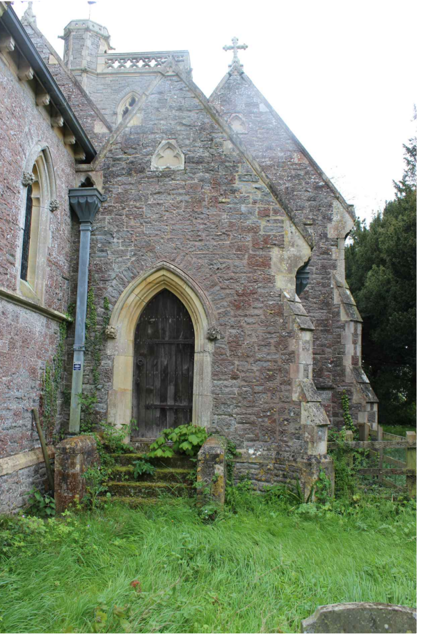
EAST ELEVATION OF EXISTING VESTRY
