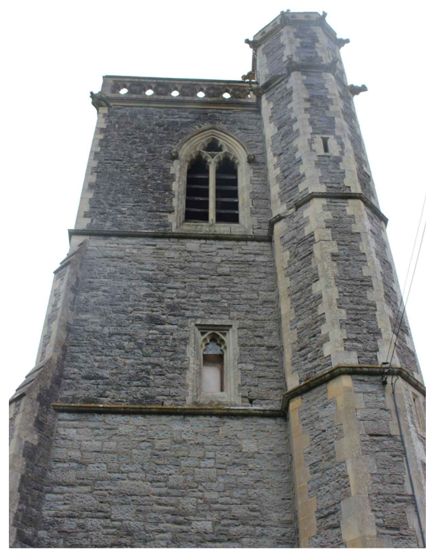
SOUTH ELEVATION OF THE TOWER (UPPER STAGES)
