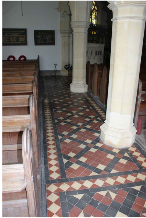
North Aisle floor tiling
