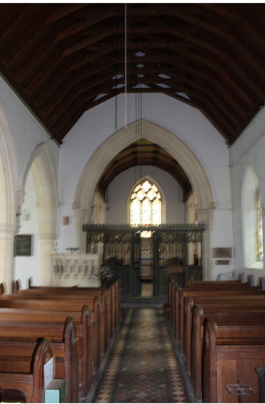
The Nave looking East
