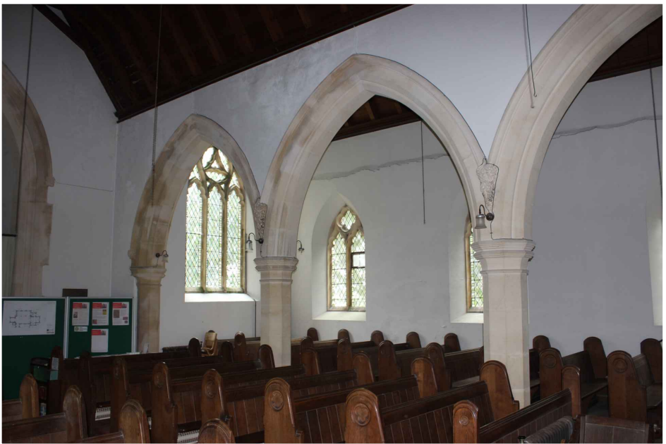
The Arcade looking North-West
