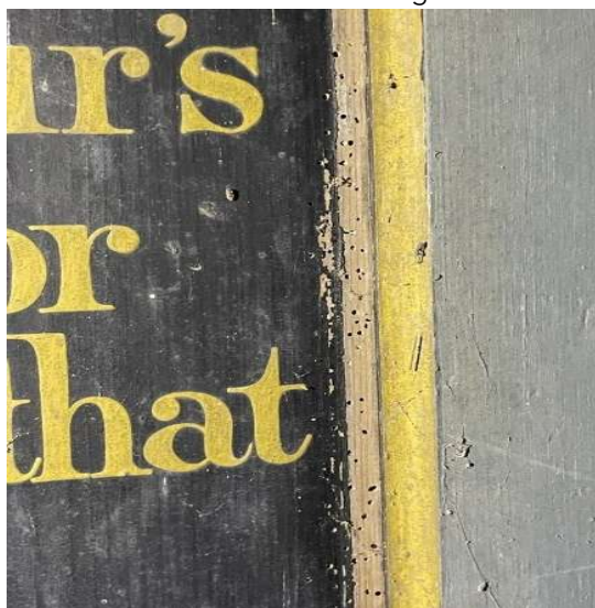
Figure 16 The frame is made up of several components, including the moulds and the hollow carved frieze. This construction is sturdier than the commemoration board (the black inner board), which may explain why the frame is in better condition than the inner -pai
