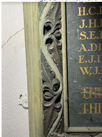
Figure 3 The outer and inner frame borders are painted sage green, and the wavy line that runs between the ornately carved leaves is also painted sage green. The carved leaves are exposed dark wood with remnants of faded gold paint.
