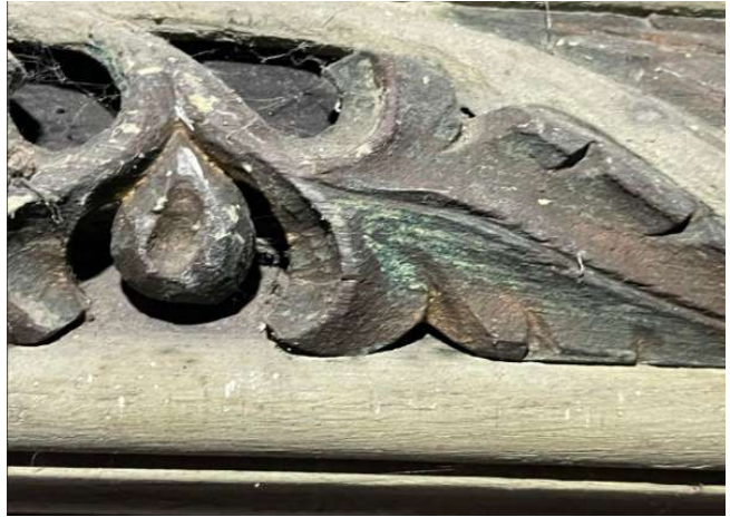
Figure 21 Green oxidation is visible on the carved sections, which may indicate that the substrate was coated with a gold-like paint, such as bronze or copper alloys. This type of paint tends to oxidize in the presence of moisture.
