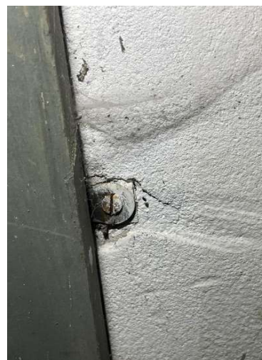
Figure 15 One of the four wall brackets that attach the boards to the wall.
