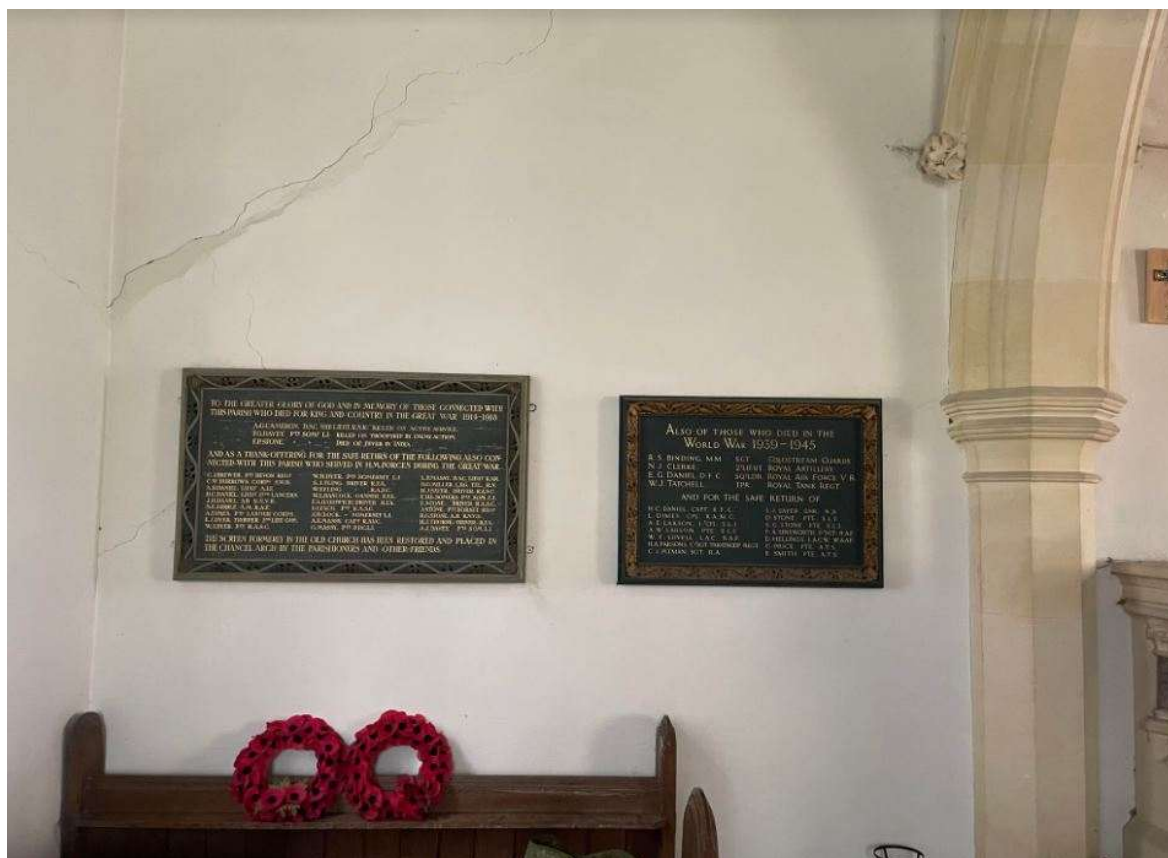
Figure 1 The war memorial plaques are located on the east wall of the north aisle
