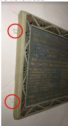
Figure 5 The memorial is attached to the wall with four brackets, two on each side.
