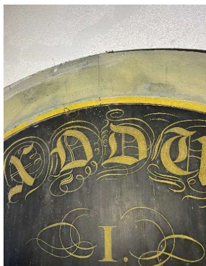
Figure 11 A close up look at the board in natural light is showing a yellow decorative calligraphy on a black background. The inner frame mould is also painted the same colour. The outer mould is painted in a thin layer of greyish green. The substrate is not primed therefore it is easy to see the wooden pattern.
