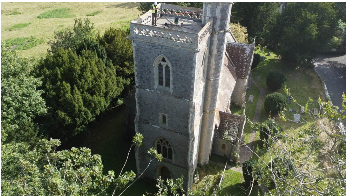
Figure 7 - DJI_0198 St Mary Magdalene Church Tower West Elevation
