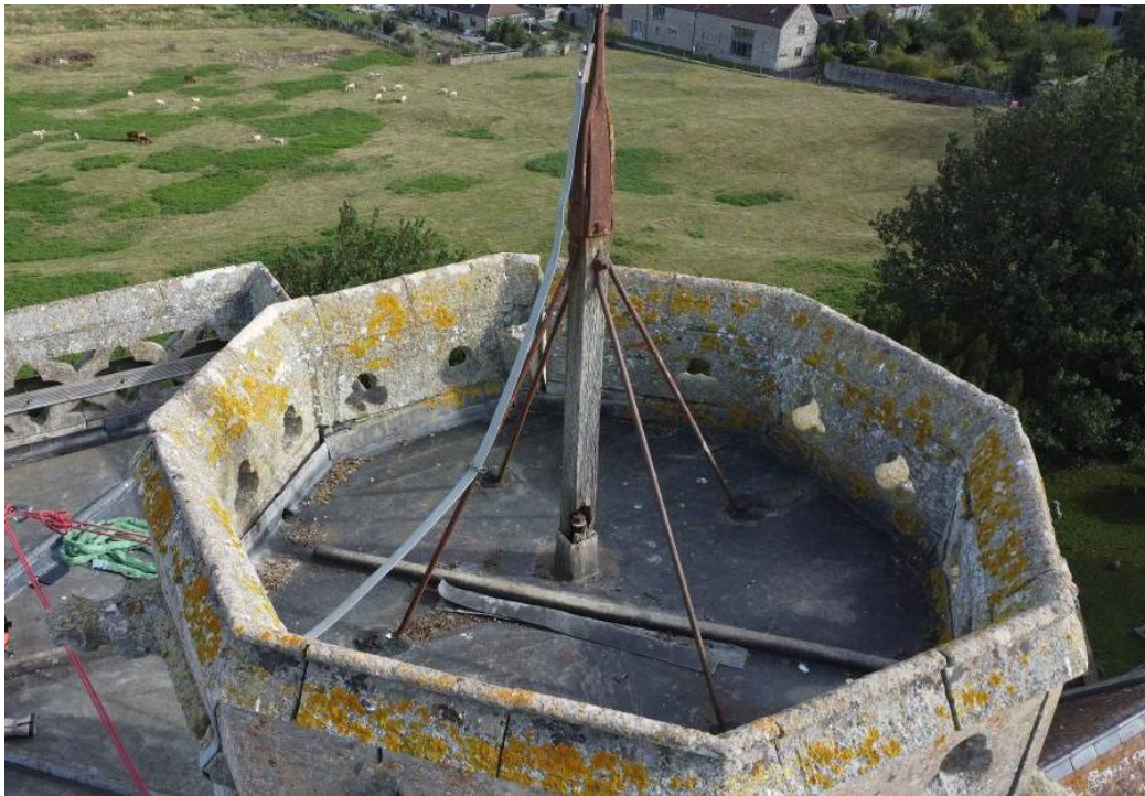
Figure 51 - Weather Vane Base in Stair Turret Roof
