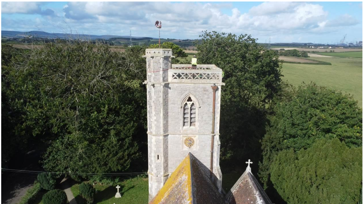
Figure 9 – DJI_0193 St Mary Magdalene Church Tower East Elevation
