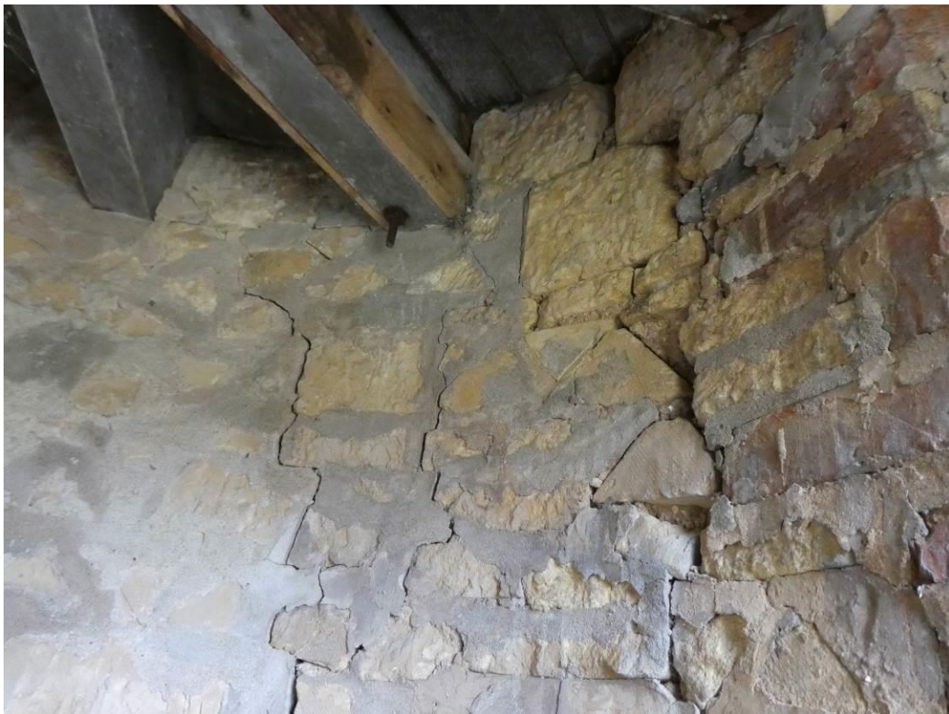
Figure 45 - P1000416 Example Open Joint Systems Inside Stair Turret Tower
