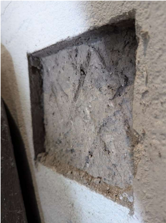
Figure 12 Upper two coats of plaster removed to reveal the grey plaster scratch-coat
