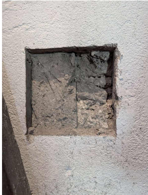
Figure 13 Further partial removal of the plaster scratch coat to reveal the stone core of the wall
