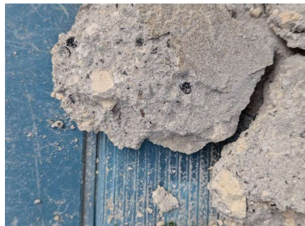
Figure 10 Detail of sample of original bedding and pointing mortar submitted for laboratory analysis
