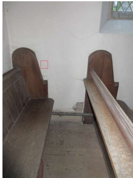
Figure 2 Location for internal plaster removal at the west end of the north aisle wall (1.2.1)
