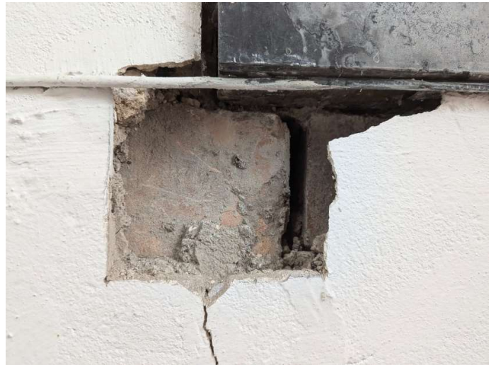
Figure 21 Second coat of plaster removed to reveal the brickwork inner skin of the wall
