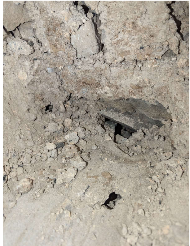
Figure 8 Detail of the wall core within the void
