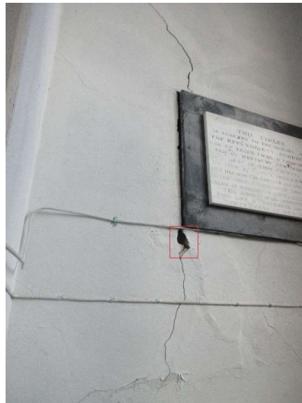
Figure 4 Location for plaster removal on the east wall of the organ chamber beneath the wall monument (1.2.3)
