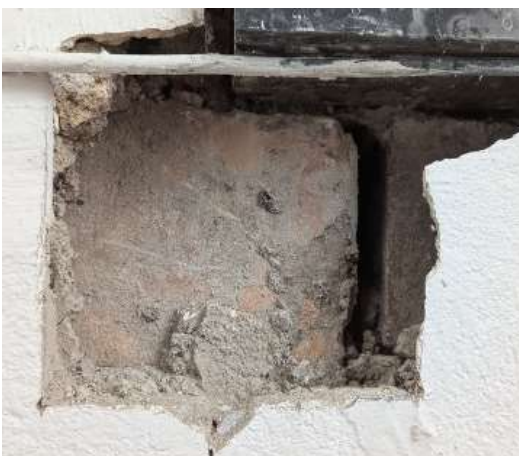
Figure 22 Detail of the brickwork and open joint
