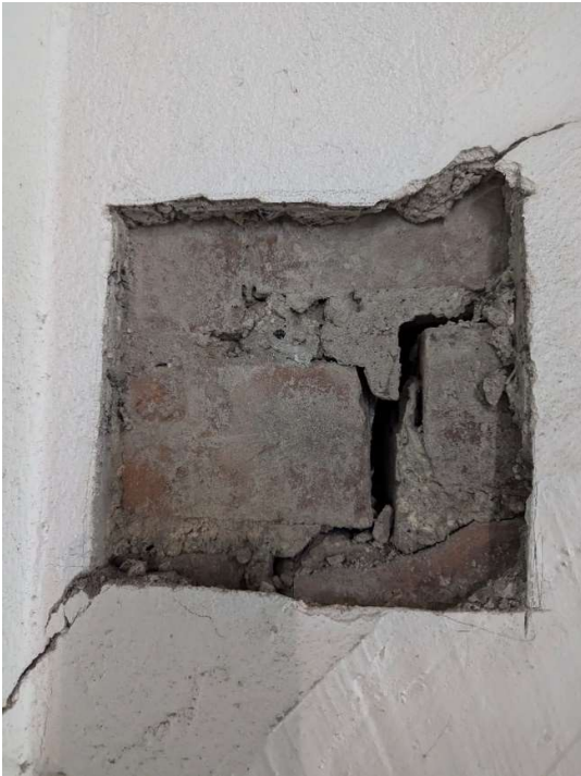
Figure 18 Second coat of plaster removed to reveal the brick inner skin of the wall
