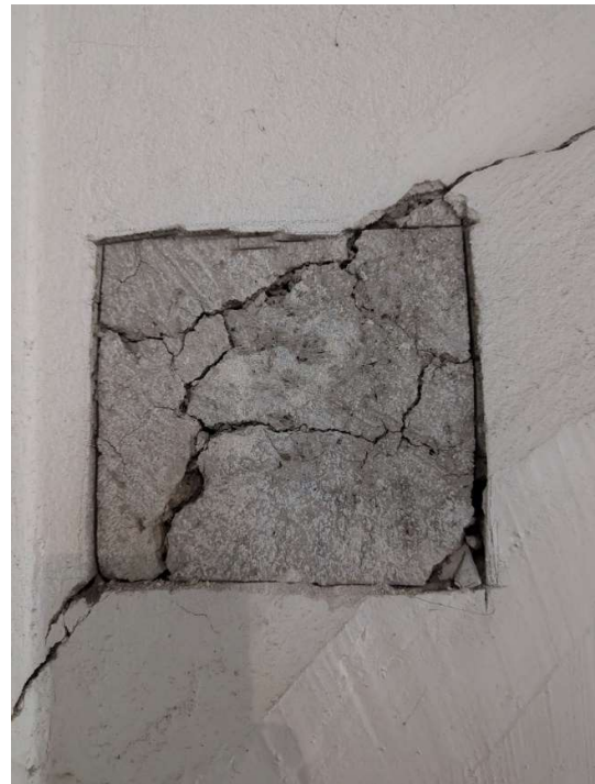
Figure 17 The window with topcoat plaster removed, revealing the second coat beneath
