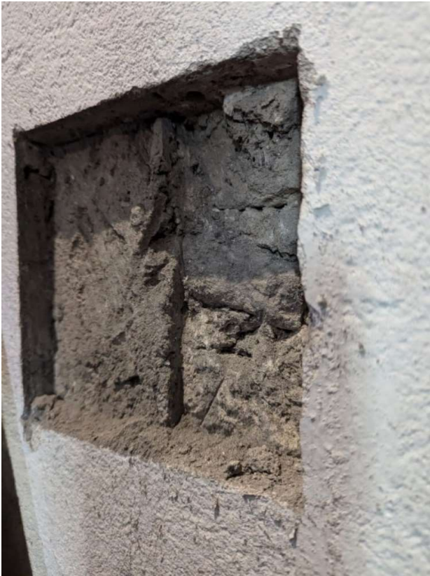
Figure 14 Detail of the partially removed scratch coat and rubble stone core
