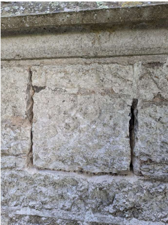
Figure 5 The stones with joints raked-out, prior to removal
