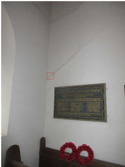
Figure 3 Location for internal plaster removal at the east end of the north aisle (1.2.2)
